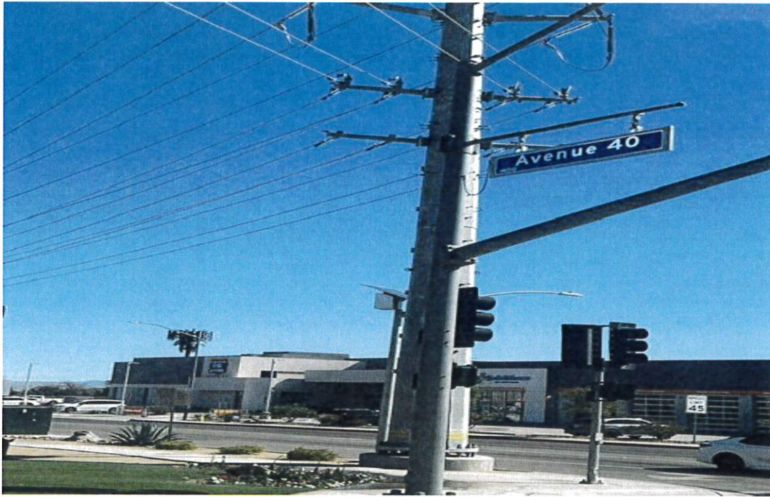
Photo 9: Views of CA Line steel structure at Avenue 40 and Adams Street.
