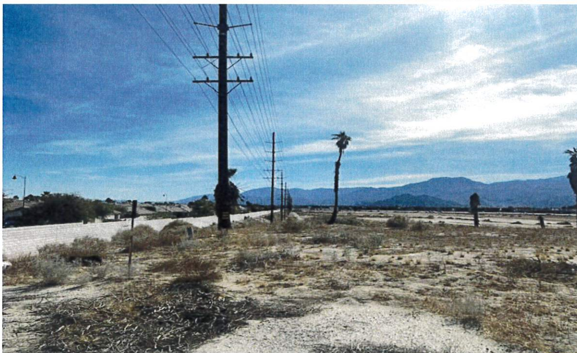
Photo 1: View south along north/south alignment of CA Line.
