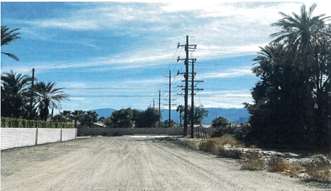
Photo 6: View of CA Line south through Sun City Shadow Hills.
