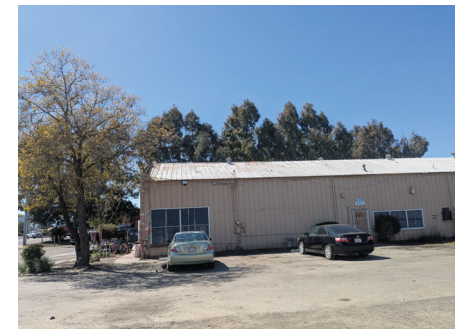
⑥ Facing west from project southeast corner near Pacheco Blvd.
