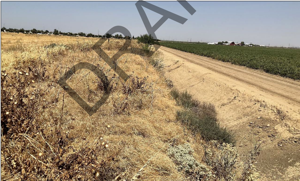
Figure 4-7 Aboveground portion of the lateral with evidence of vegetation intrusion, facing north.
