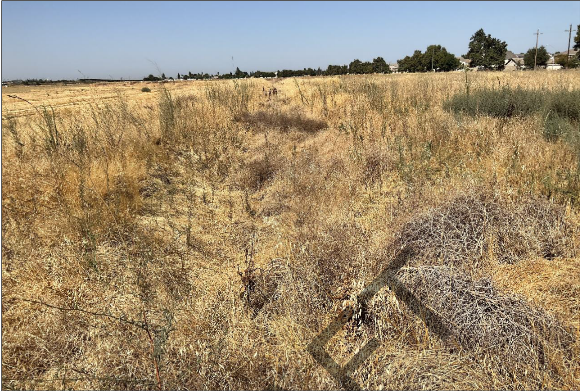
Figure 4-11 Earthen ditch with severe vegetation intrusion from east end of the segment, facing west.
