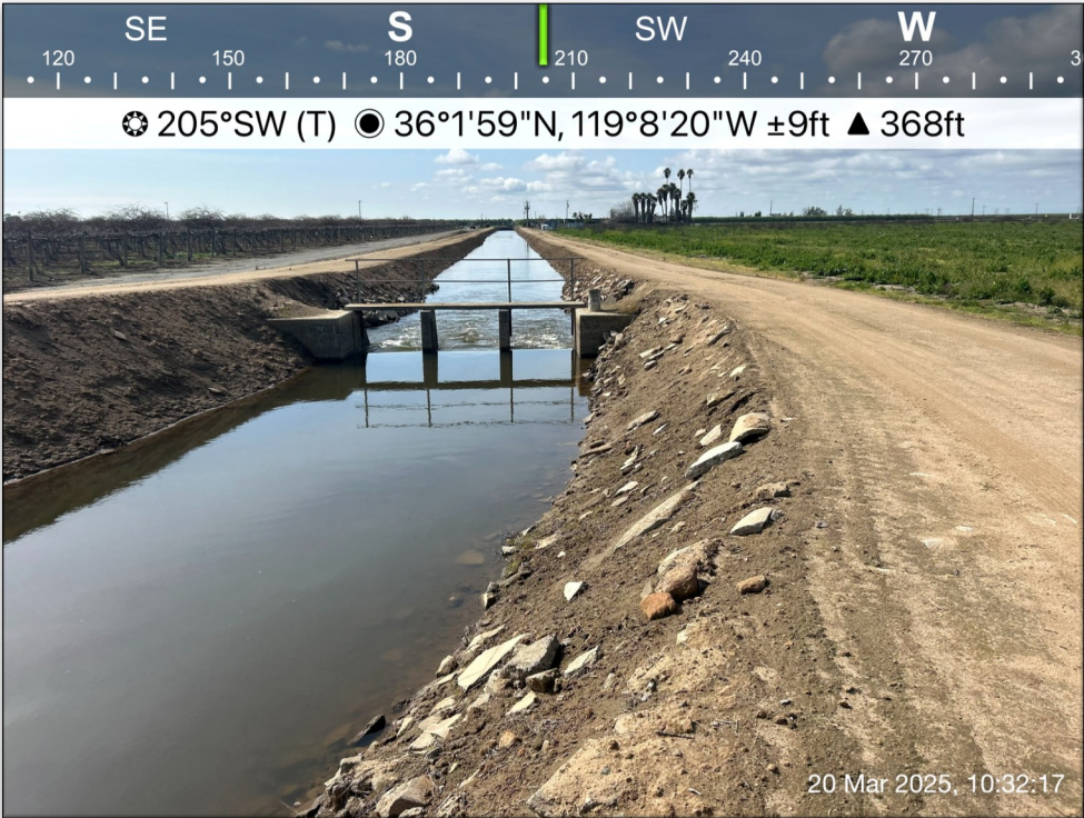
Photograph 8 Canal diversion structure along Casa Blanca Ditch.
