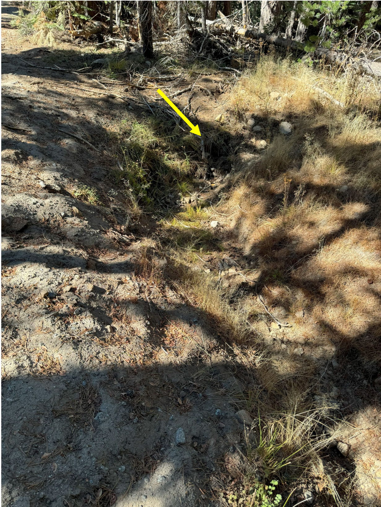
Photo 5. Looking east at the drainage along Road 8S10 downhill from the project site that will likely be used for site runoff. The arrow points to the existing culvert. The drainage would be rocked.
