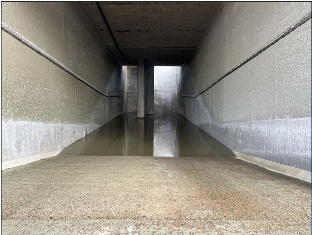
Figure 4.4-8. Flame trench at SLC-6.
