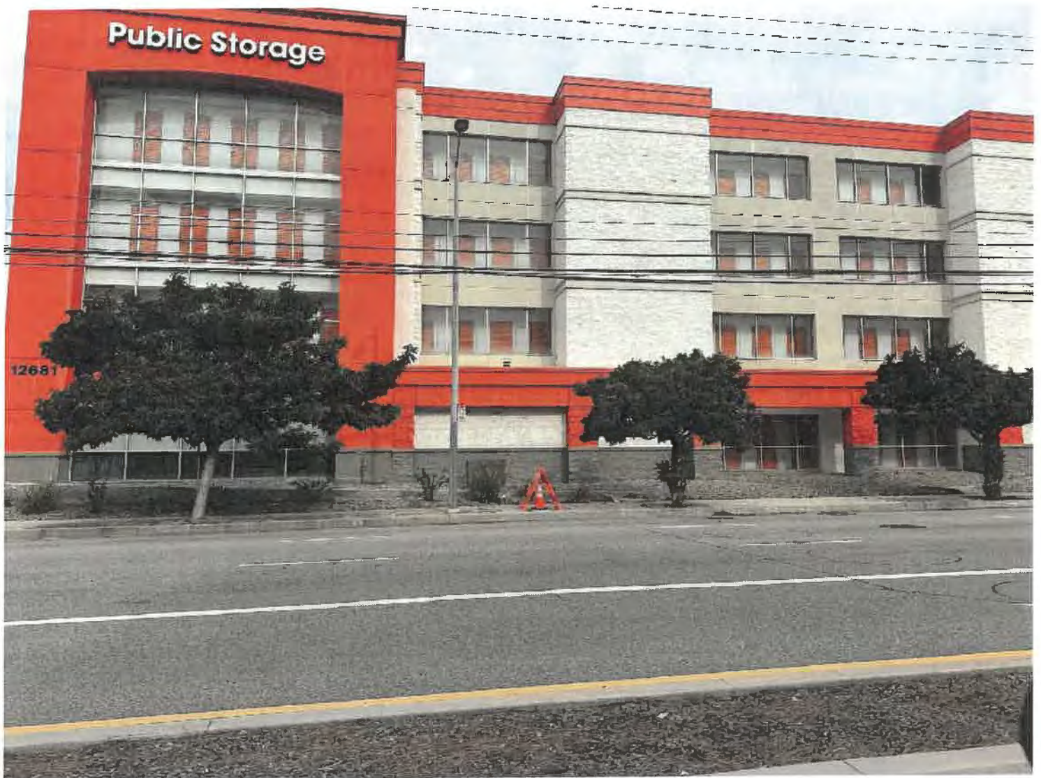
PHOTO 3 - Nine (9) Bronze loquat ( Eriobotrya deflexa ) street trees #1 - #9 will receive no impact and will be retained and protected in place.
