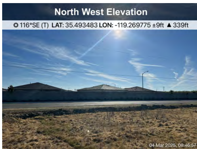
Photograph 6. Existing residential development to the east of the Project Site.
