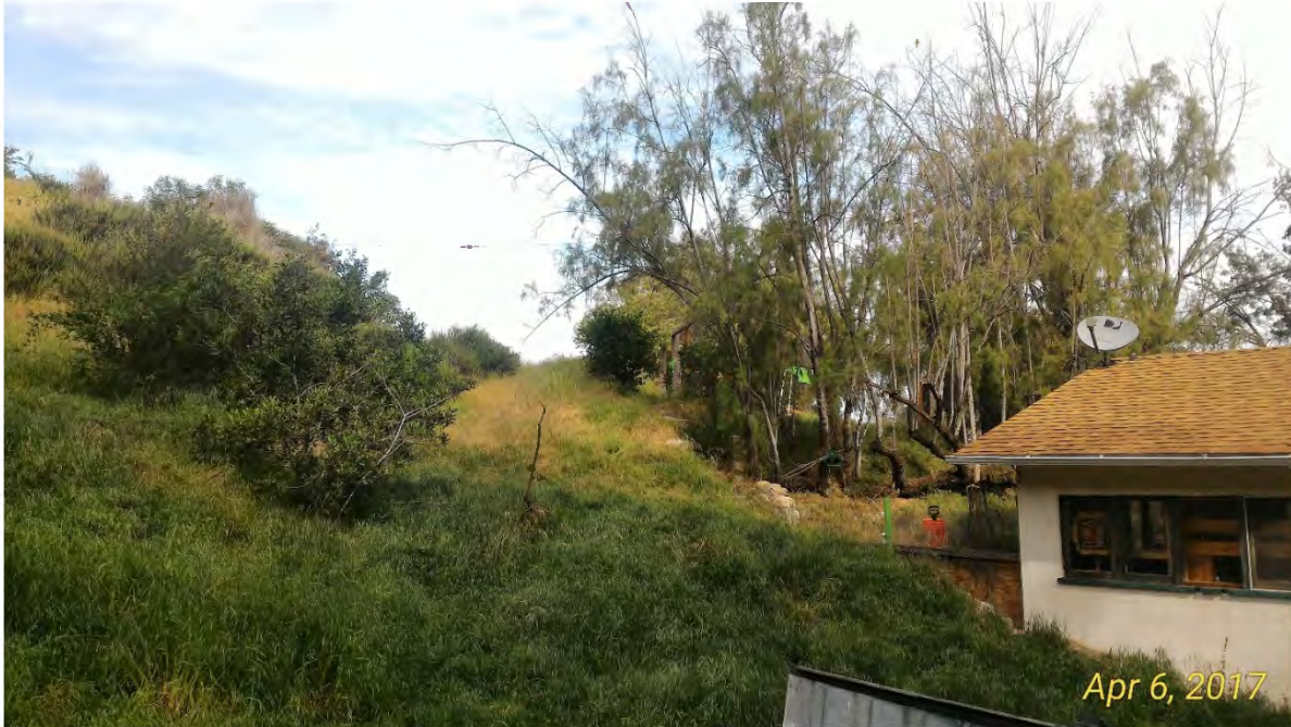
Photograph 3. Residential structure on developed portion of project site. View looking northwest.
