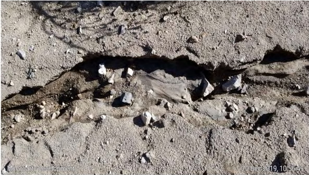
Photograph 13. Top-down view of western drainage feature. Note: visible bed and bank.
