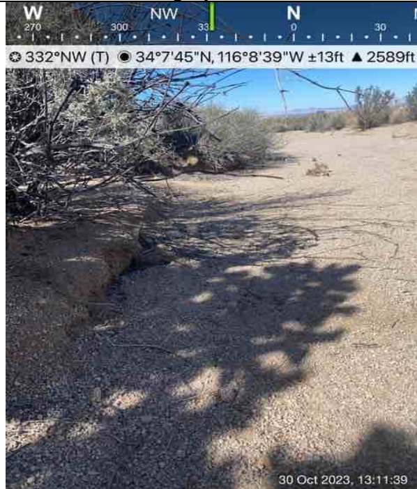
Photo 2: Facing northwest. View of shelving along Drainage B.
