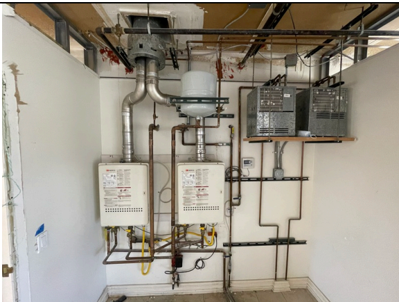
17. View of water heater and electrical hookups on third floor renovation of main building on Subject Property
