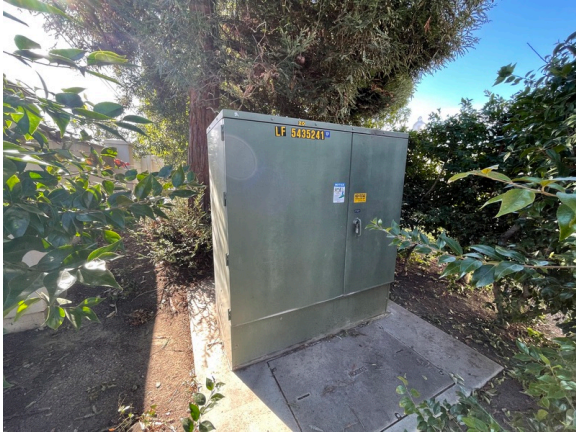
19. Oil-filled transformer located on concrete pad on eastern portion of Subject Property
