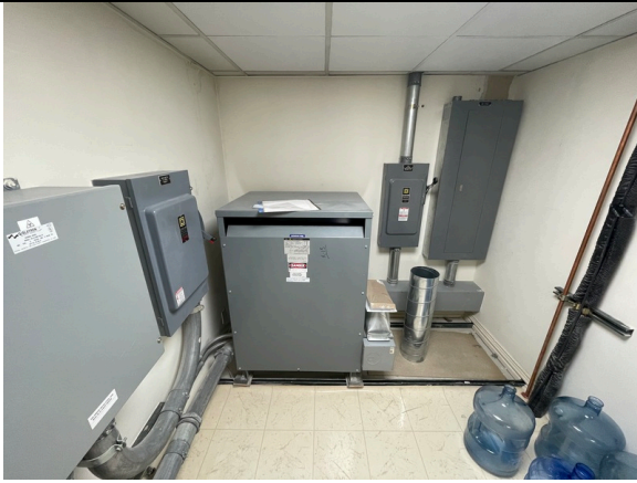
1. Dry-style transformer located in maintenance room in main building on Subject Property
