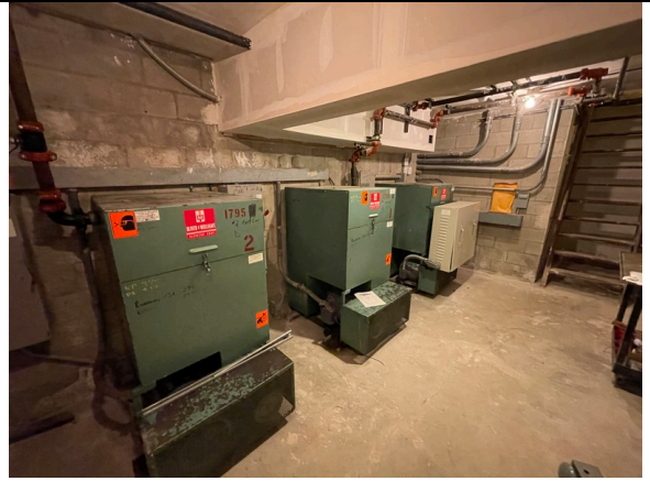
2. Elevator systems located within partial basement area within main building on Subject Property
