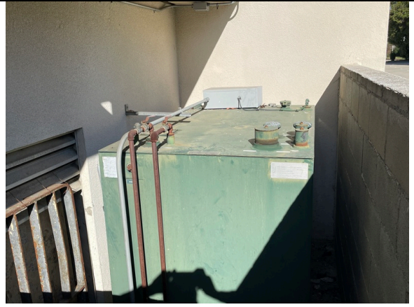
8. 500-gallon diesel AST attached to emergency generator located within enclosure in maintenance building
