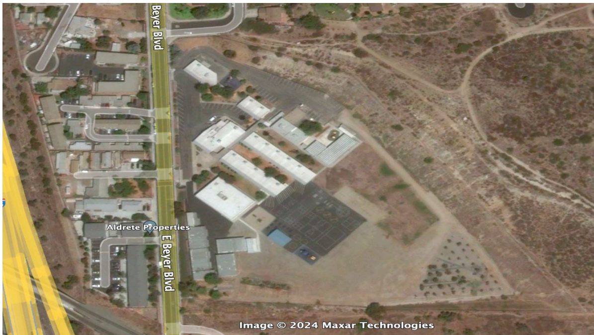
Photo 20: Google Earth aerial imagery from August 13, 2012, that depicts the former Beyer Elementary School still standing within the proposed Project footprint.
