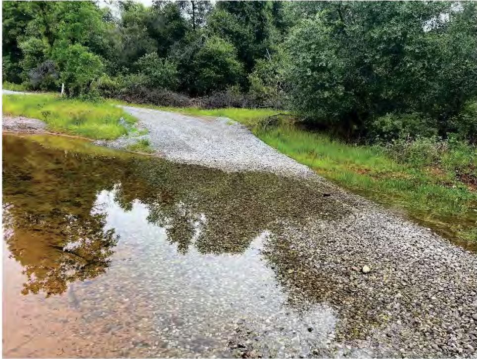
Photo 1: Low water crossing over access road
