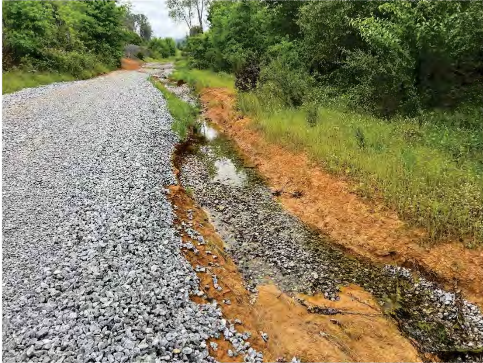
Channelization along the existing access road
