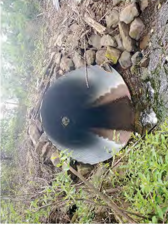
Figure 2a. Existing Culvert Inlet
