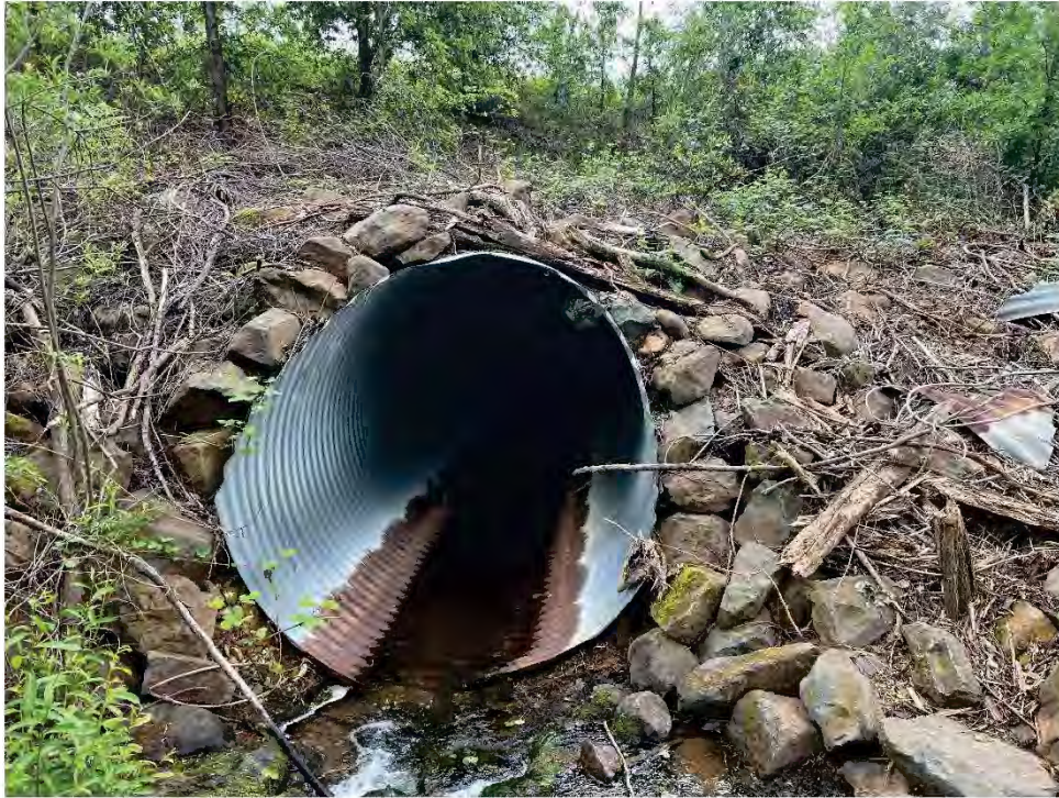
Existing CMP culvert to be replaced
