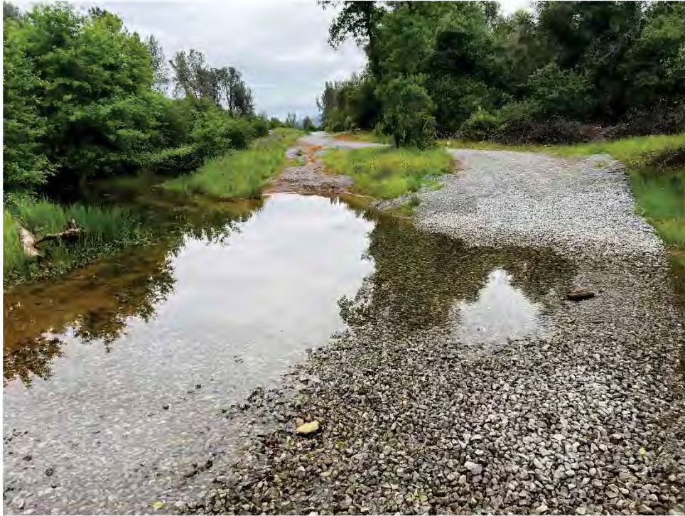
Low water crossing of Newtown Creek along the railroad access road
