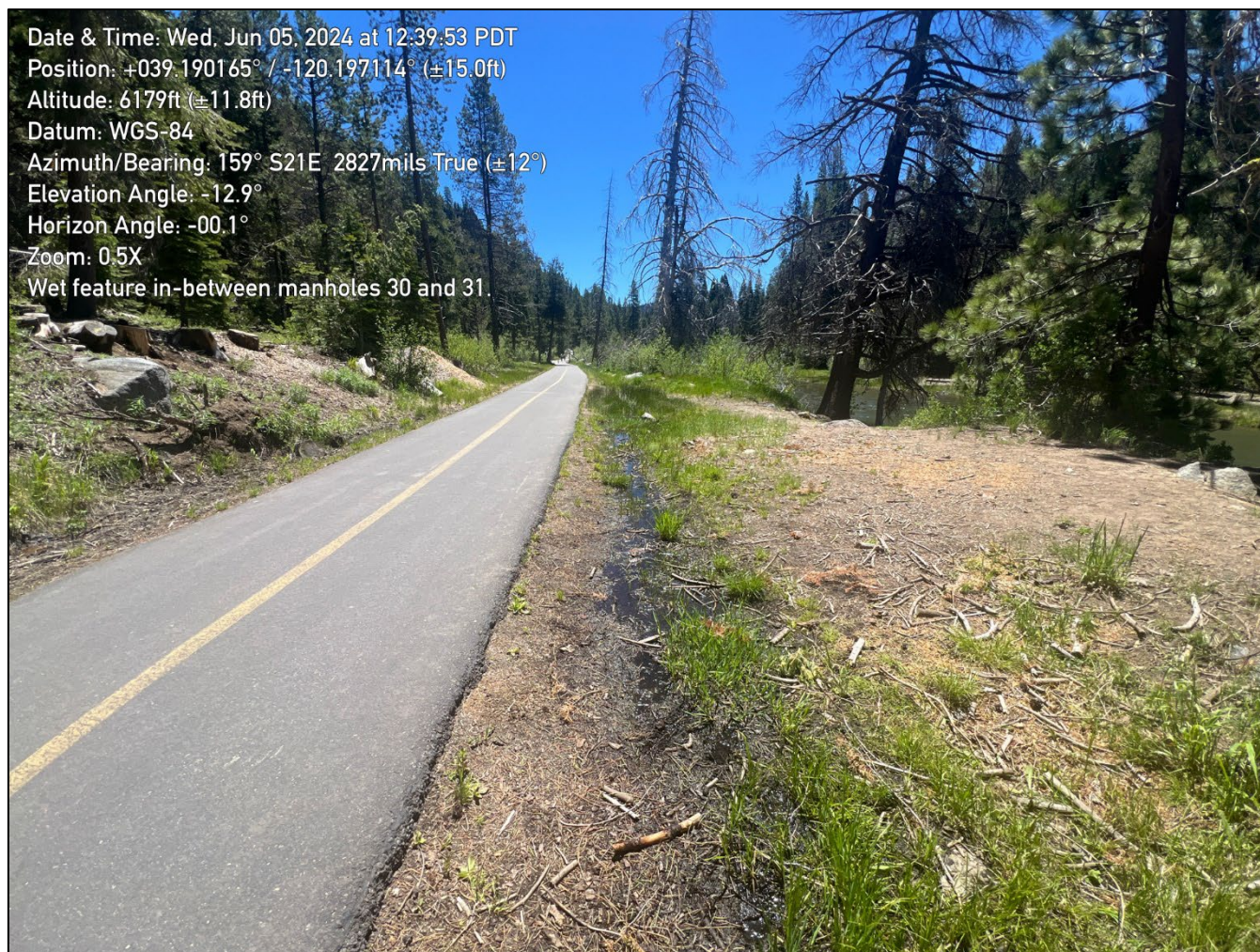
Photograph 3. Wet ponded area adjacent to the multi-use path.
