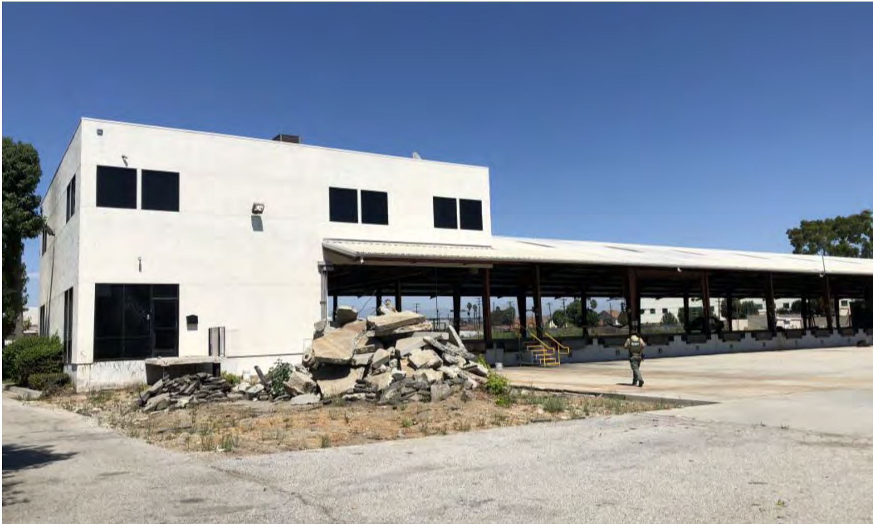
View northeast of Building C.
