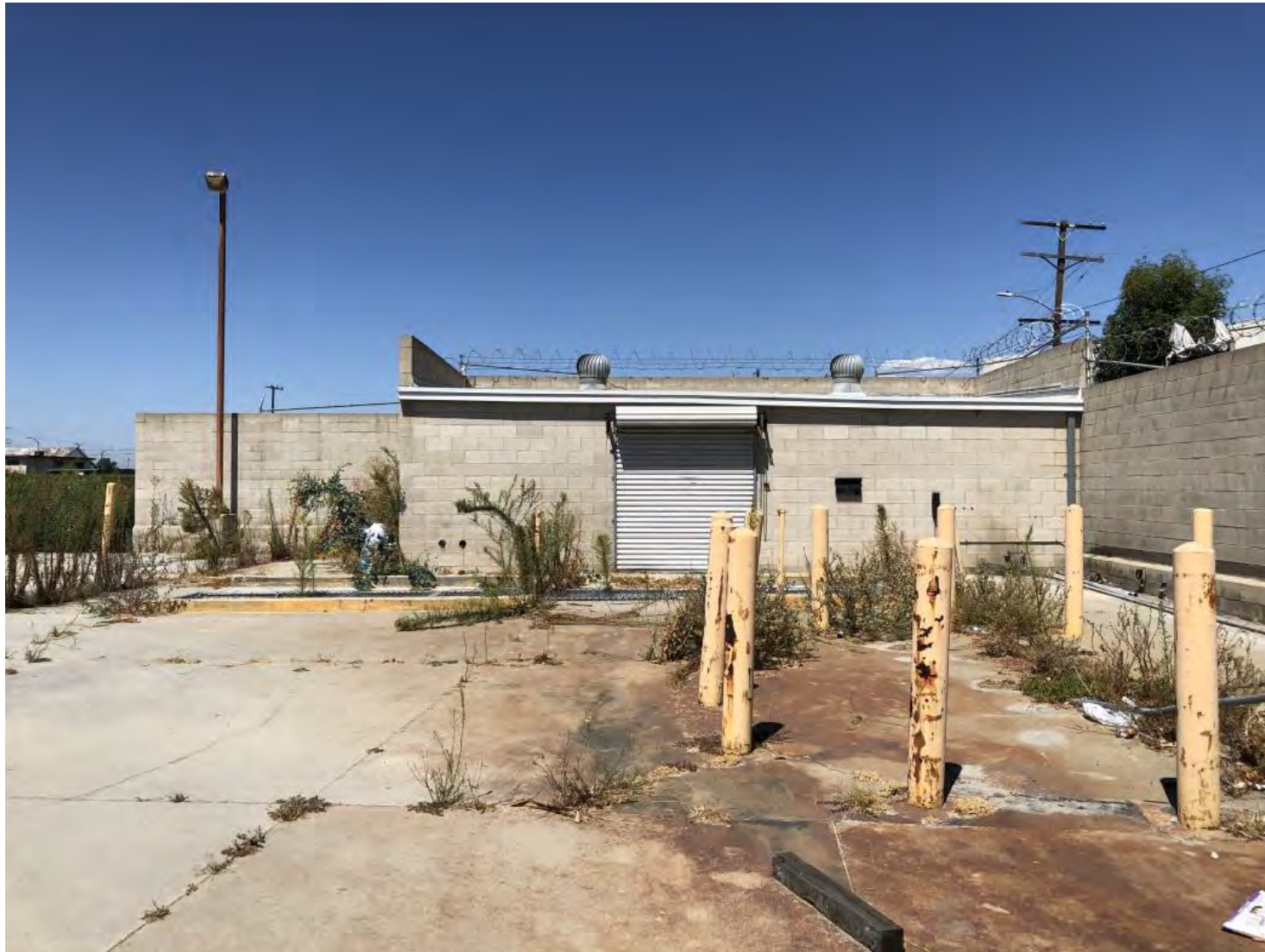
View north of Building E.
