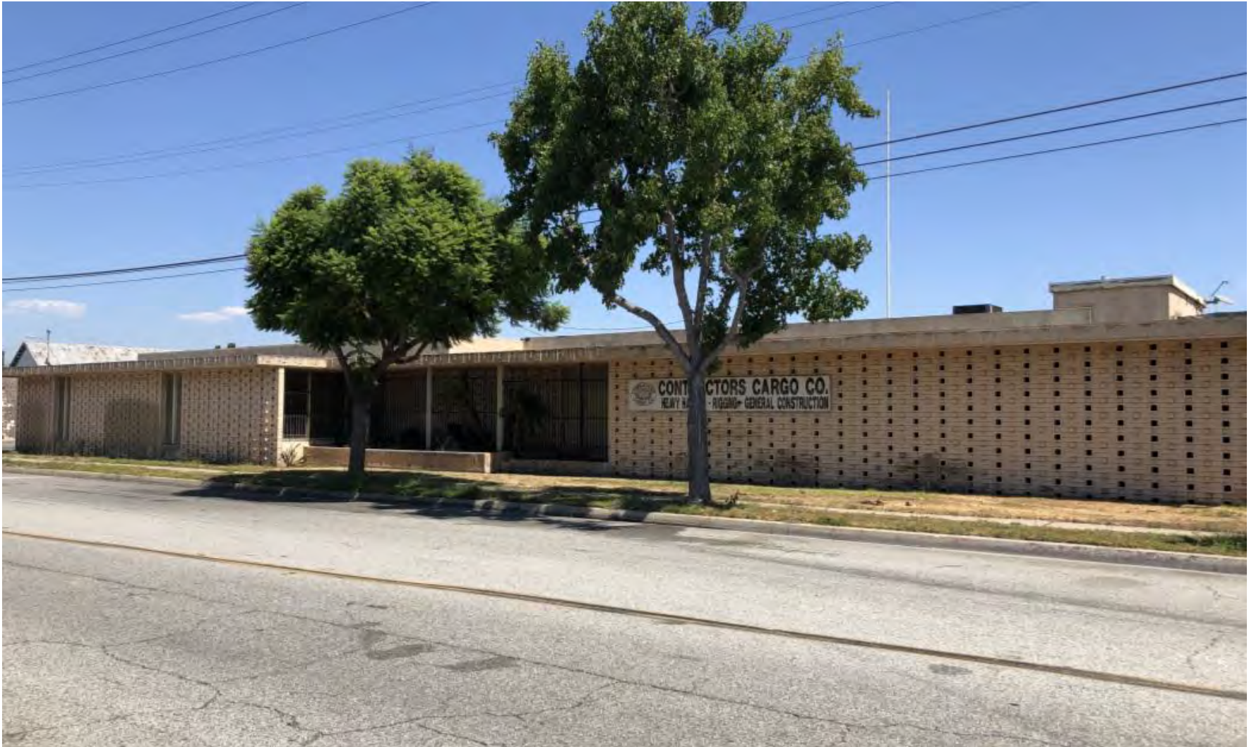
View northwest of the front (west) elevation of Building A from S. Alameda Street.
