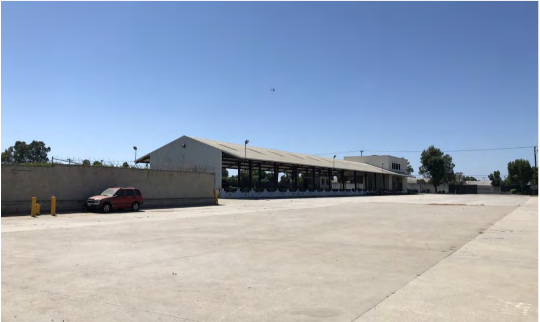
View southwest of Building D.
