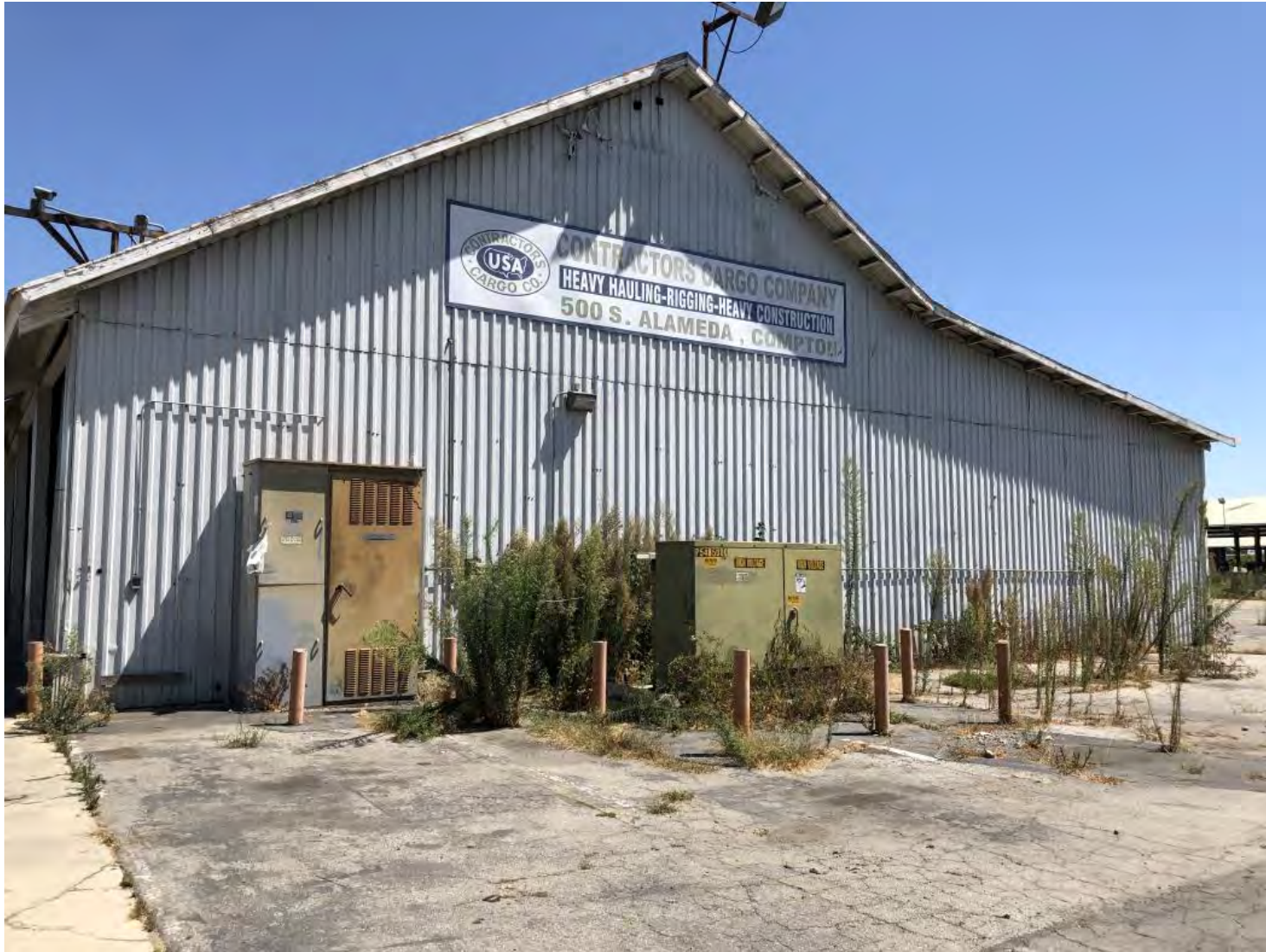
View east of the west elevation of Building B.
