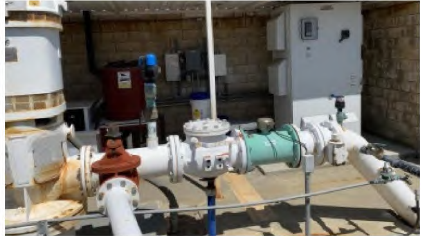
Photograph 2. Existing Lost Canyon 2A well vertical turbine pump.
