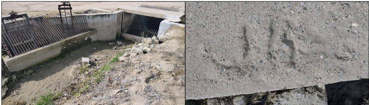
Culvert to the east. Left : underground canal entrance, view to the east; right : "JR 56" written on top of the culvert
