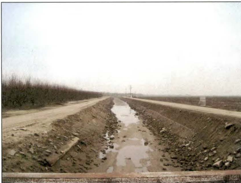
Photo 1. View of Main Canal, looking north.
