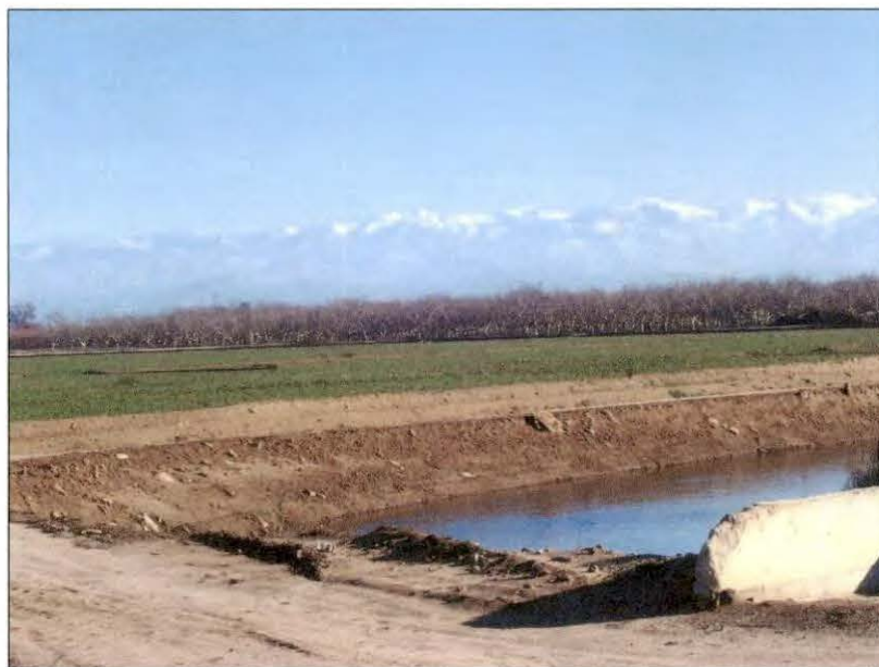
Photo 2. View of Main Canal, looking east.
