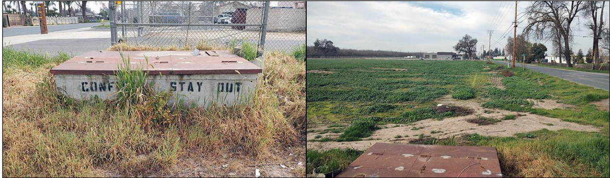
Canal elements and path. Left : access box, view to the east; right : path of canal from box, view to the west
