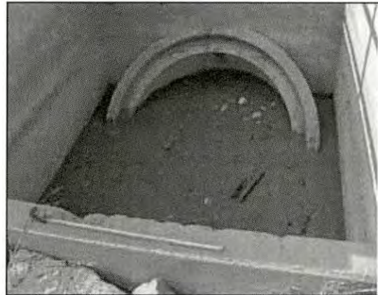
Figure 4, Frame 267. Segment 1 culvert underneath Road 148. Tape measure extended to 3 feet.
