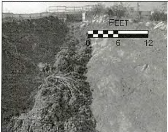
Figure 3, Frame 266. Segment 1 underneath the Big Creek Transmission Line. Facing west.
