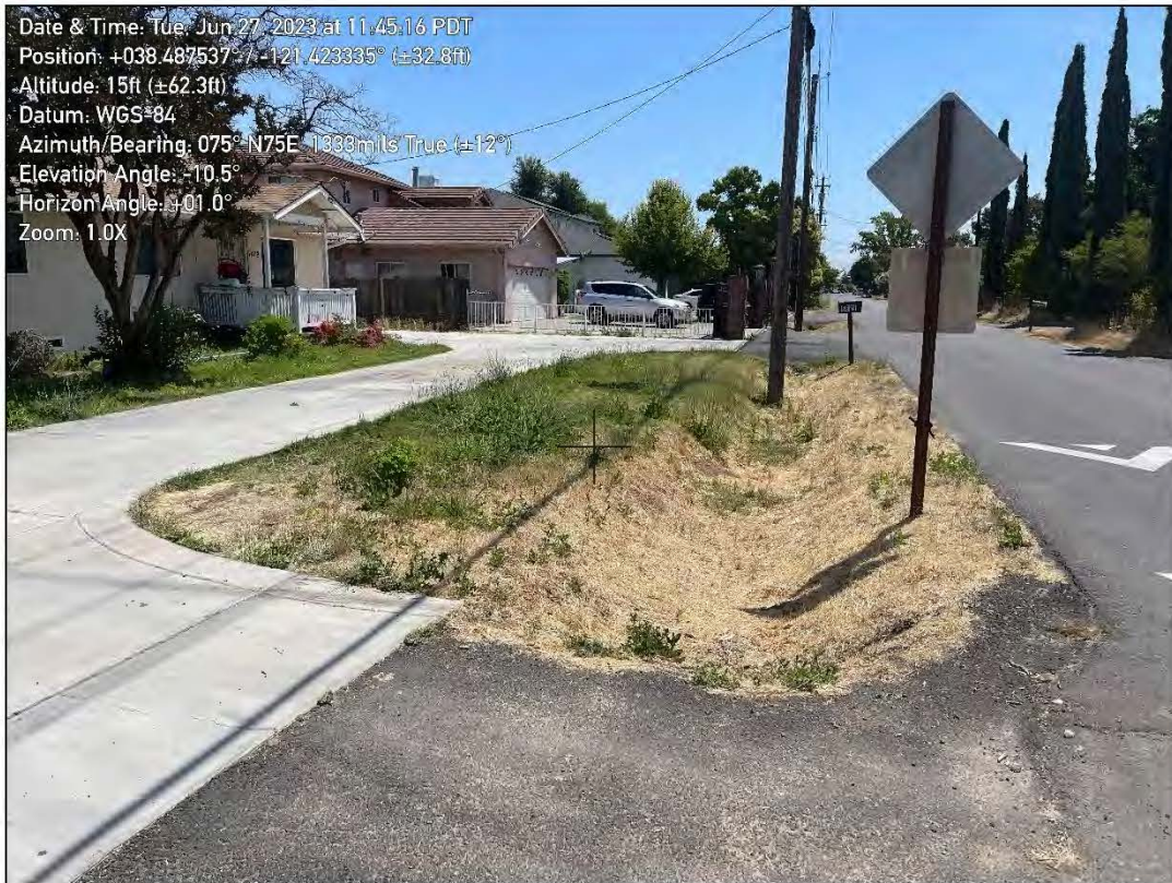
Facing east at the non-aquatic resource roadside ditch along Fleming Avenue.
