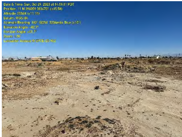
Cracked soils indicative of ponding water, northwest corner of site facing south.
