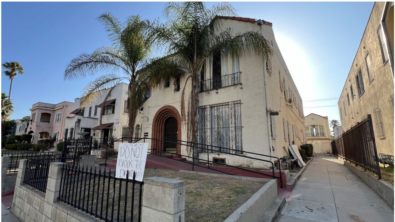
Figure 20: 3825 Flower Drive (Parcel 8), view looking southwest. GPA Consulting, September 2024.
