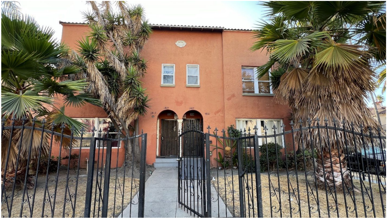
Figure 15: 3801 Flower Drive (438 W. 38 th Street, Parcel 3), view looking west. GPA Consulting, September 2024.
