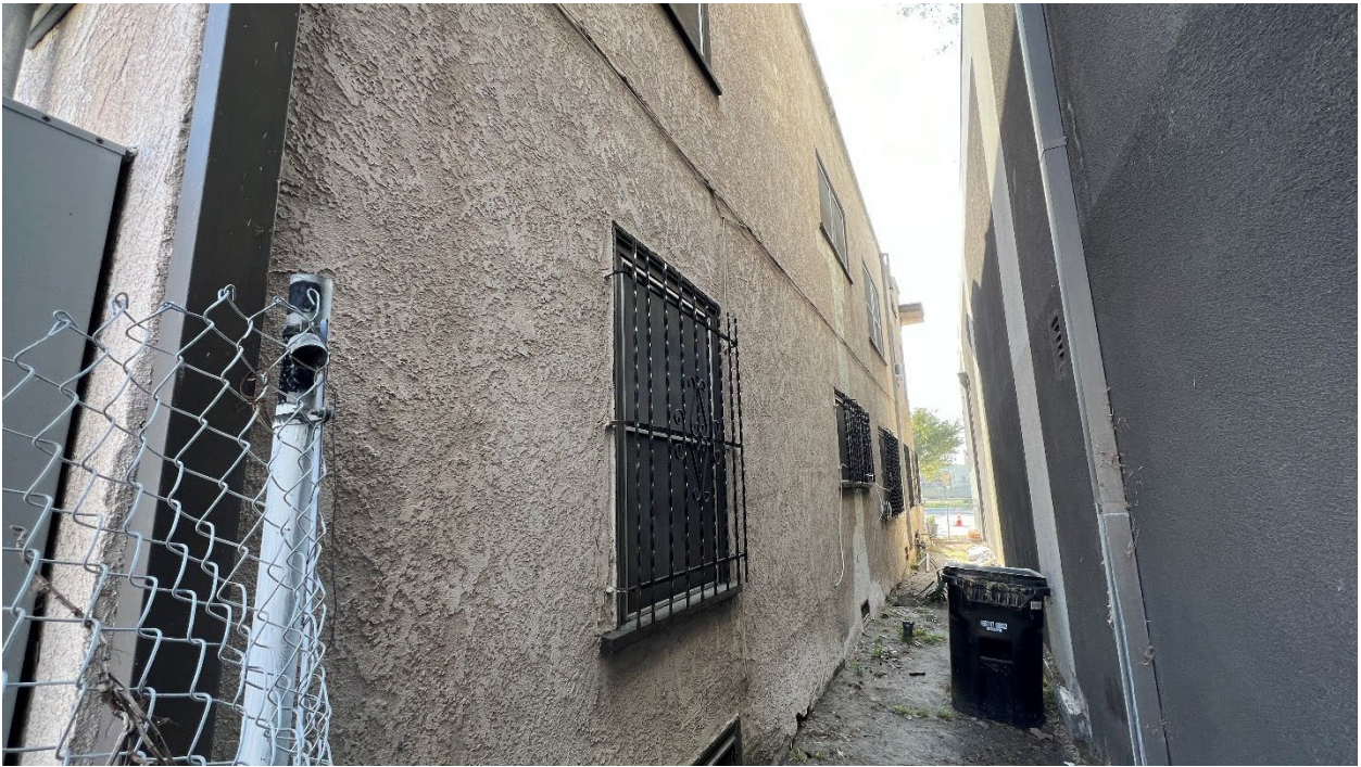
Figure 10: 3822 S. Figueroa Street, north (side) elevation, looking southwest. GPA Consulting, September 2024.
