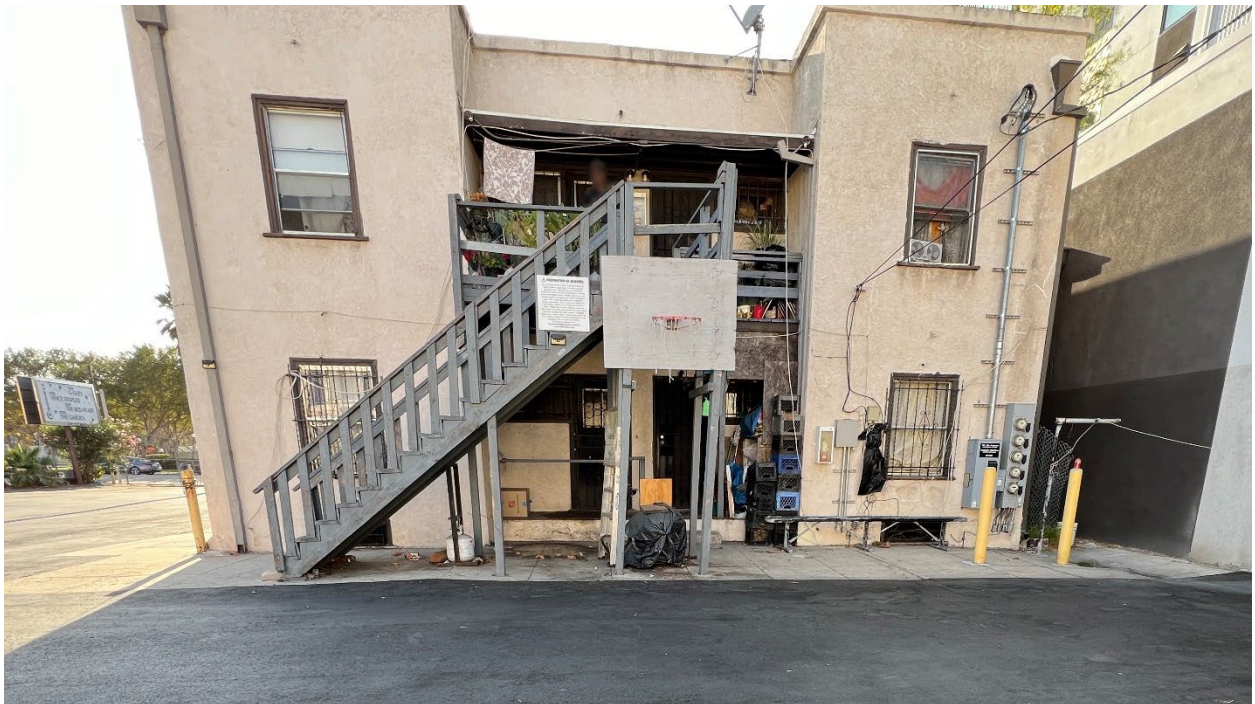
Figure 9: 3822 S. Figueroa Street, east (rear) and elevation, looking west. GPA Consulting, September 2024.
