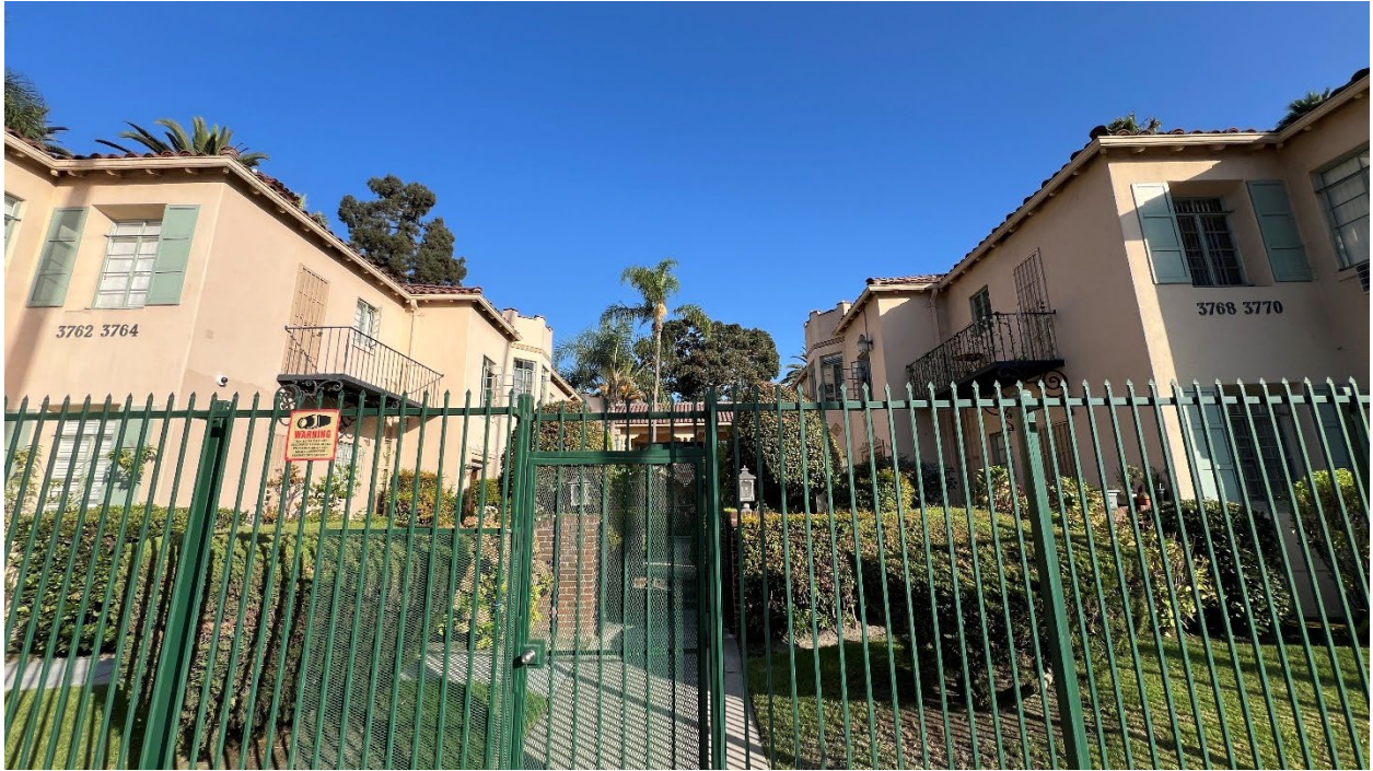
Figure 23: Zobelein Estate/Zobelein Courtyard Apartments (B1), view looking east. GPA Consulting, September 2024.
