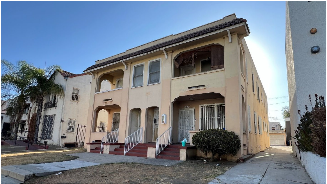
Figure 19: 3821 Flower Drive (Parcel 7), view looking southwest. GPA Consulting, September 2024.
