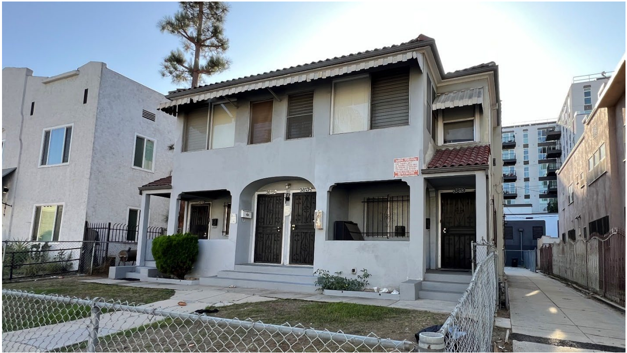
Figure 17: 3813 Flower Drive (Parcel 5), view looking southwest. GPA Consulting, September 2024.
