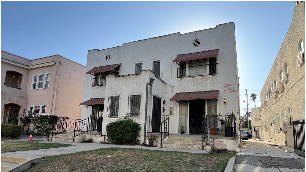
Figure 21: 3831 Flower Drive (Parcel 9), view looking southwest. GPA Consulting, September 2024.
