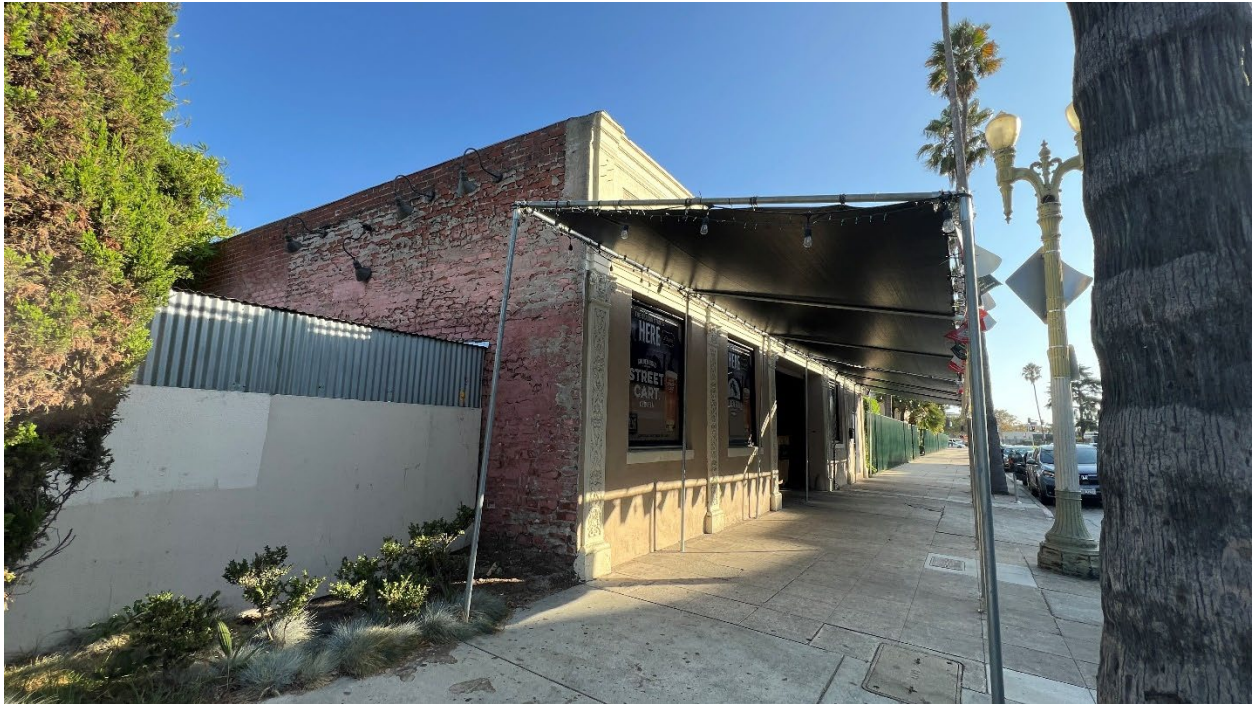
Figure 25: Zobelein Estate/Zobelein Courtyard Apartments (B3), view looking southwest. GPA Consulting, September 2024.
