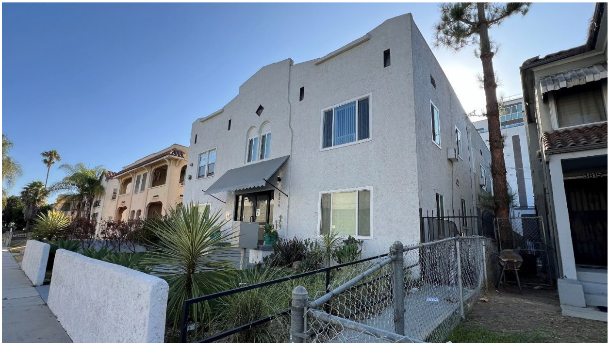
Figure 18: 3819 Flower Drive (Parcel 6), view looking southwest. GPA Consulting, September 2024.
