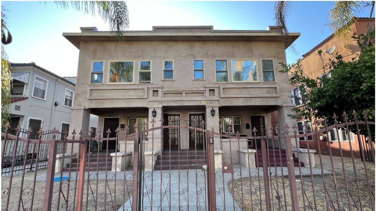
Figure 16: 3809 Flower Drive (Parcel 4), view looking west. GPA Consulting, September 2024.
