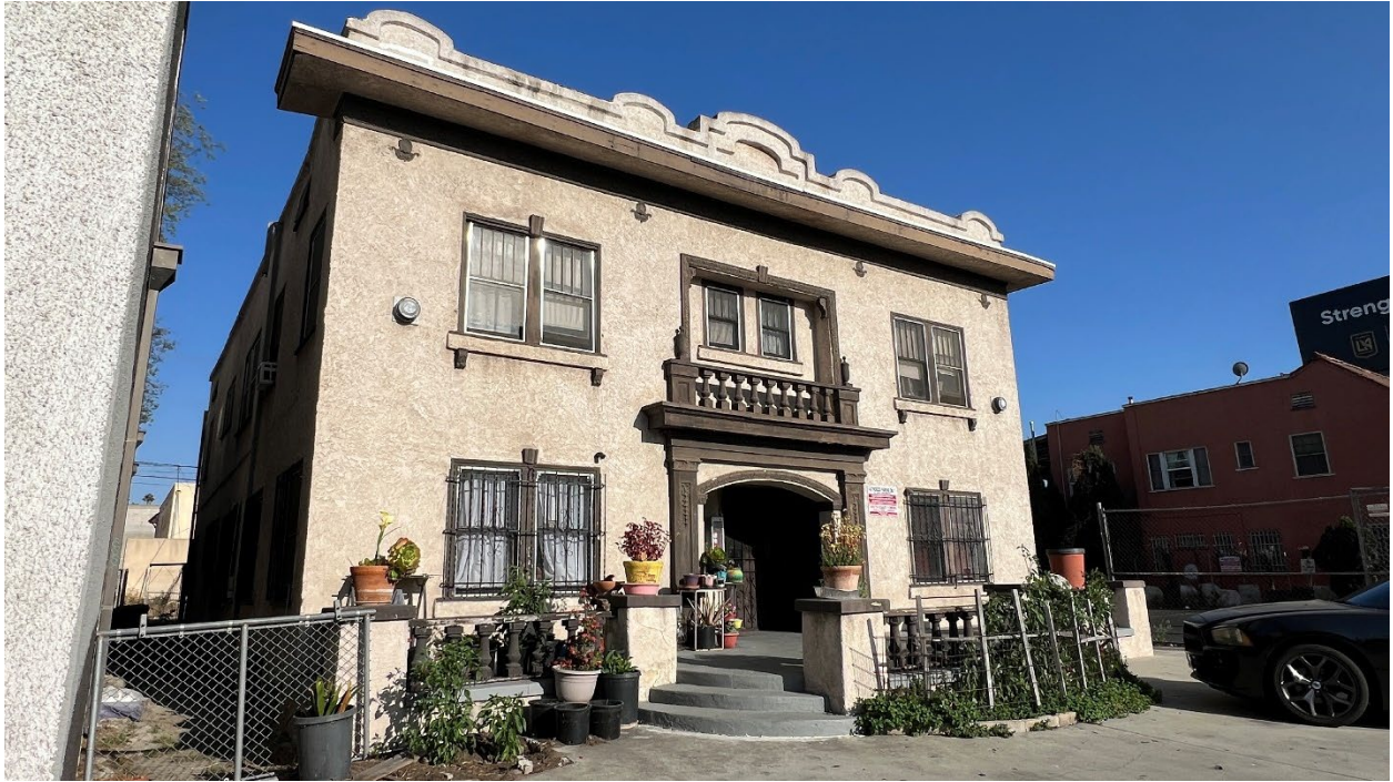
Figure 6: 3822 S. Figueroa Street, west (front) and north (side) elevations, looking southeast. GPA Consulting, September 2024.
