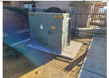
Photo No.7 – Pad-mounted electrical transformer located adjacent and west of the Heritage Community Center building.
