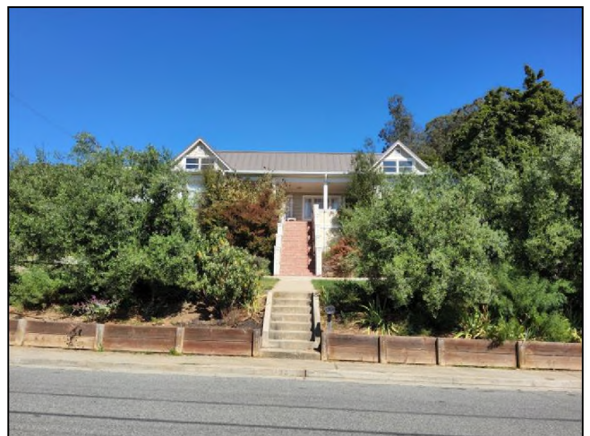
Photo 3822. 1332 Navellier St., view to northeast
