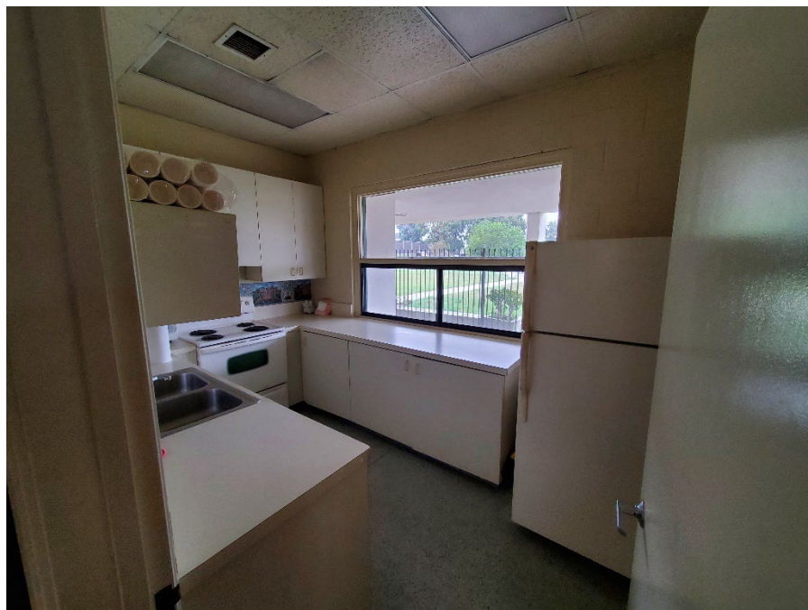
Photograph 18: View of the Kitchen in the Preschool Building. The undercoating of the sink visible on the left of the photo was identified as ACM.
