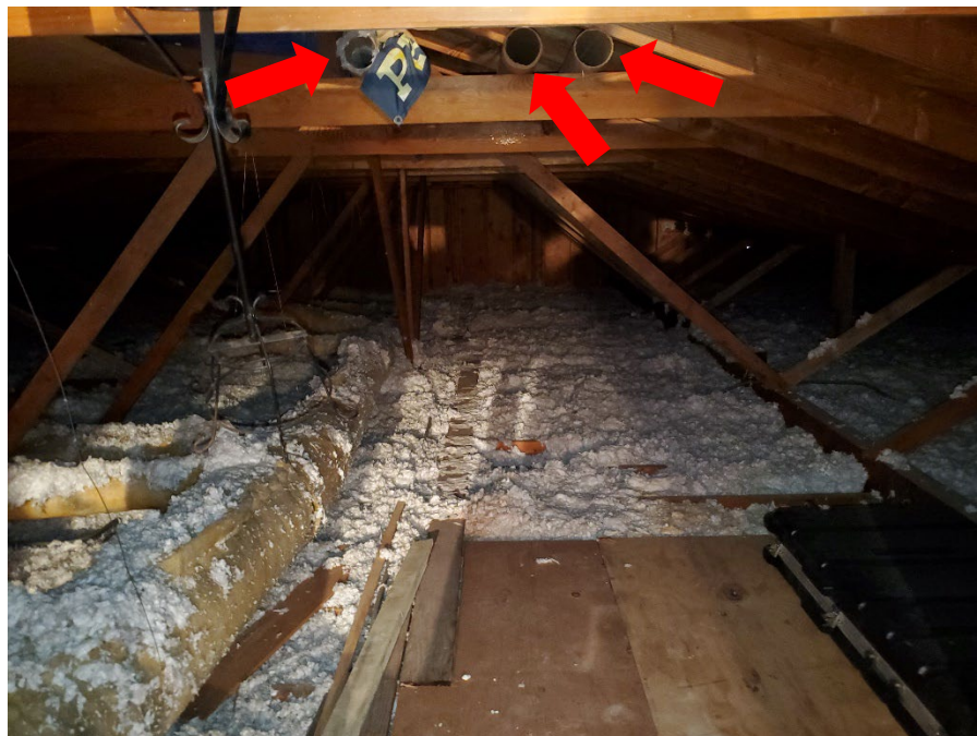
Photograph 22: View of potential additional transite flues (see markers) in the Church Building attic.
