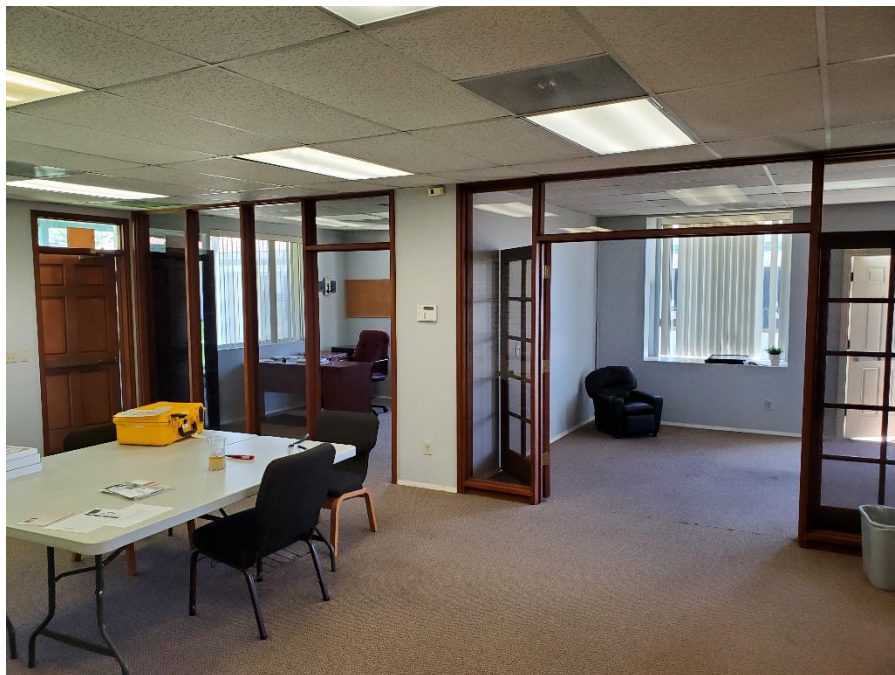
Photograph 10: View of southern portion of the Office Building. Typical acoustic panel ceilings, drywall walls, and carpet floors are visible.
