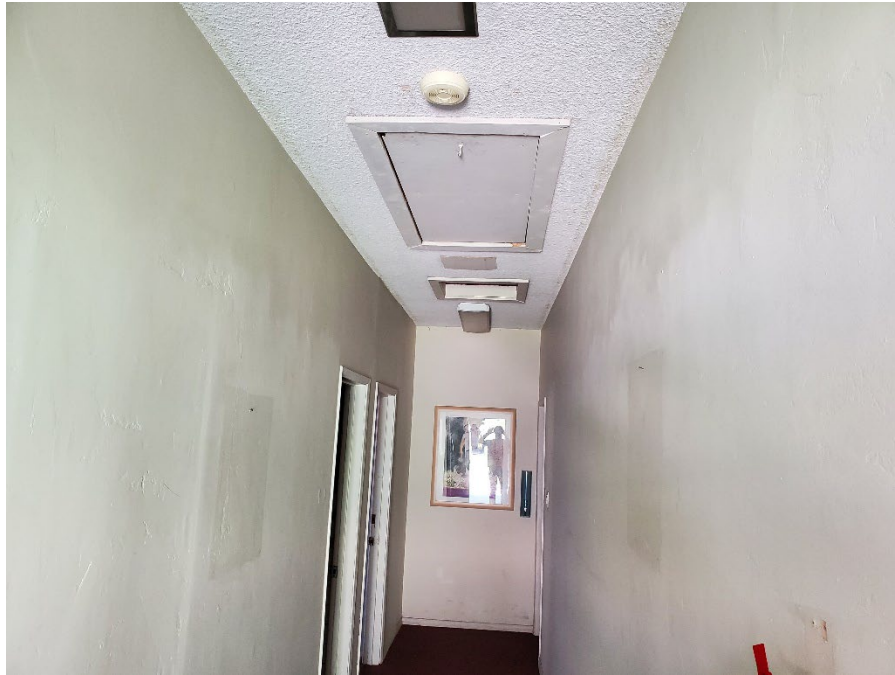
Photograph 11: View of North Hall of Office Building. The spray-applied ceiling and vinyl tile beneath carpeting from this area north were identified as ACM. The plaster walls were identified as ACCM.
