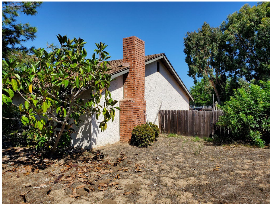
Photograph 2: View of the chimney at the Residence. Caulking at the brink-stucco joint was identified as ACM.
