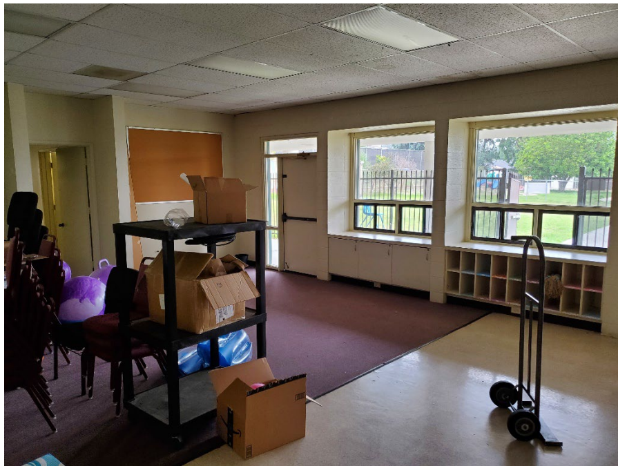
Photograph 16: View of typical Classroom in the Preschool Building. Typical acoustic panel ceiling, drywall and concrete masonry unit walls, and carpet and vinyl sheet floors are visible.
