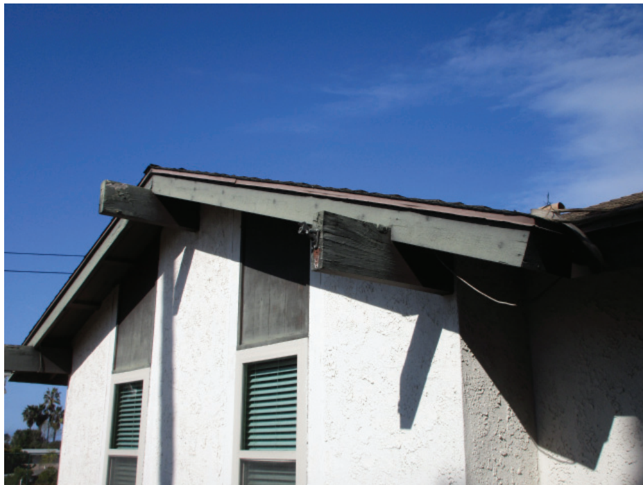
Photo 58: Looking northwest at the three 4x rafter tails supporting the gable roof.
