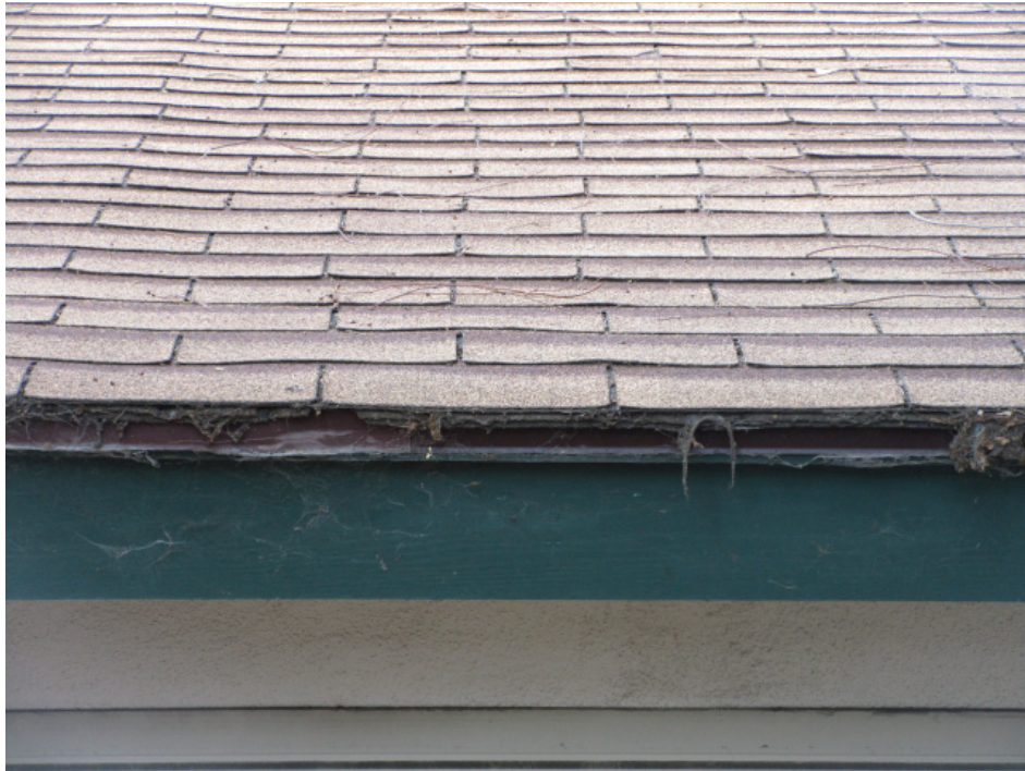
Photo 15: Detail photo showing the non-original asphalt shingle roofing at the main Church building.
