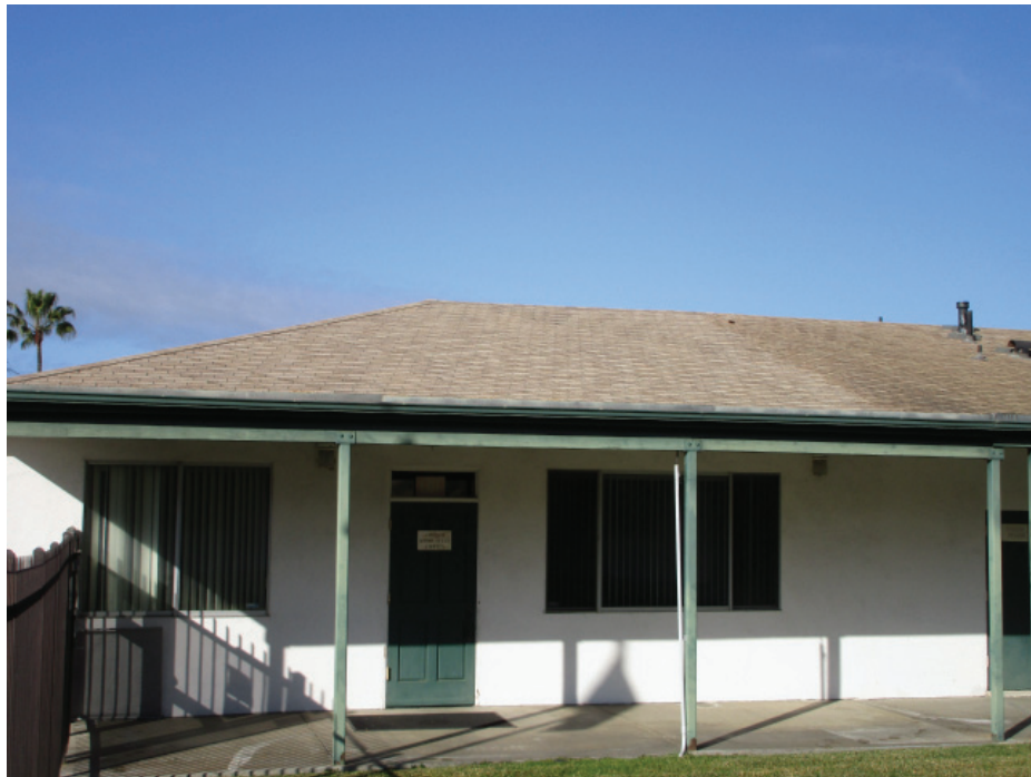
Photo 31: Looking west at the east side of the 1989 addition at the rear of the Fellowship Hall. The asphalt shingles, aluminum windows, hollow metal door, and metal weep screed at the base of the wall all differ from the original construction.
