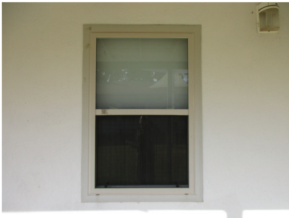
Photo 34: Detail photo showing a typical vinyl replacement single-hung window with vinyl trim surround.
