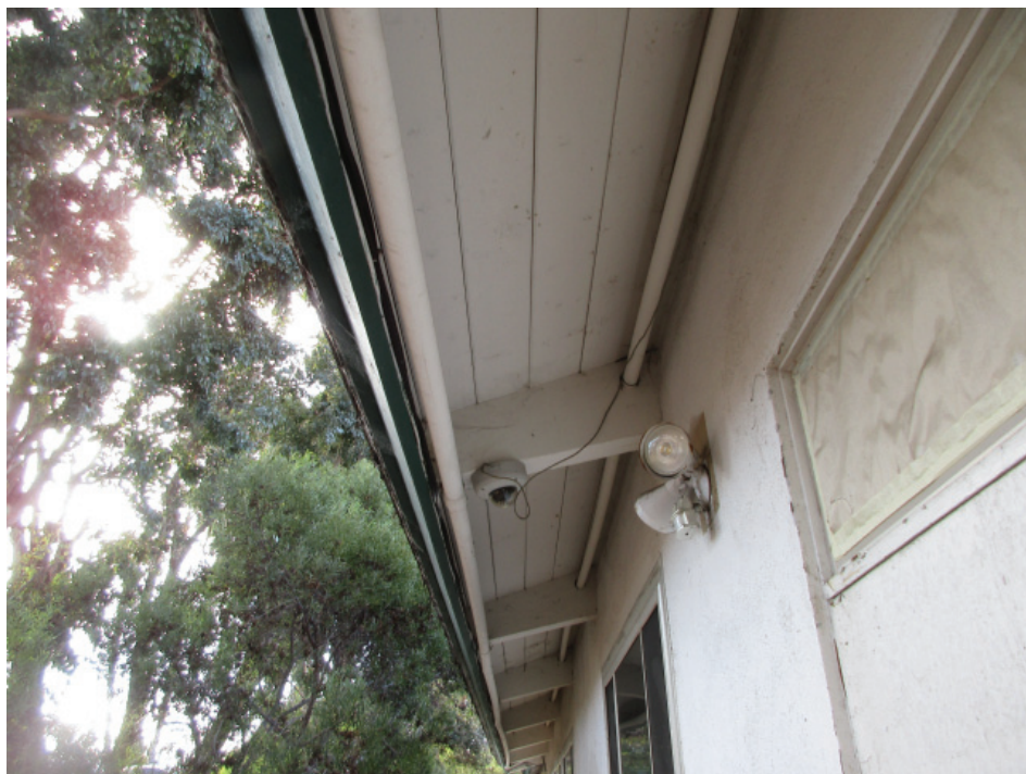
Photo 12: Detail photo of the main Church building showing the open roof eave overhang at the east facade with exposed shaped rafter tails and 1x v-groove T&G decking.
