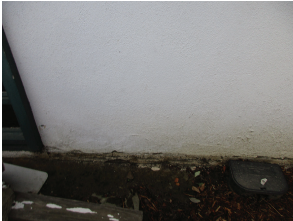
Photo 11: Detail photo showing the smooth sand texture stucco finish at the main Church building.
