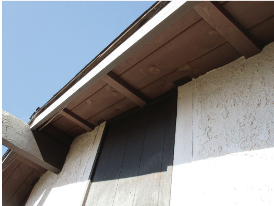
Photo 57: Detail photo showing the underside of the open gable rake at the primary south facade with exposed purlins and wood decking.
