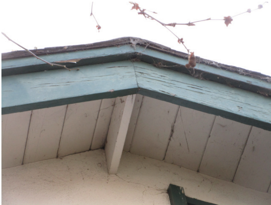
Photo 13: Detail photo showing the open roof rake at the north facade of the main Church building.
