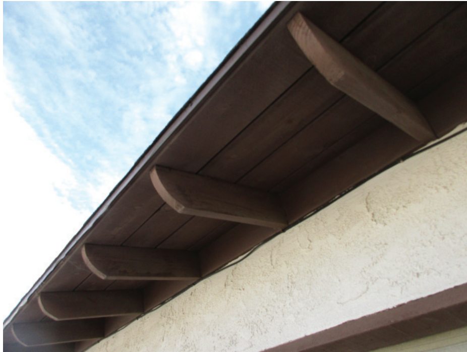
Photo 59: Detail photo showing the curved rafter tails at the secondary west facade.
