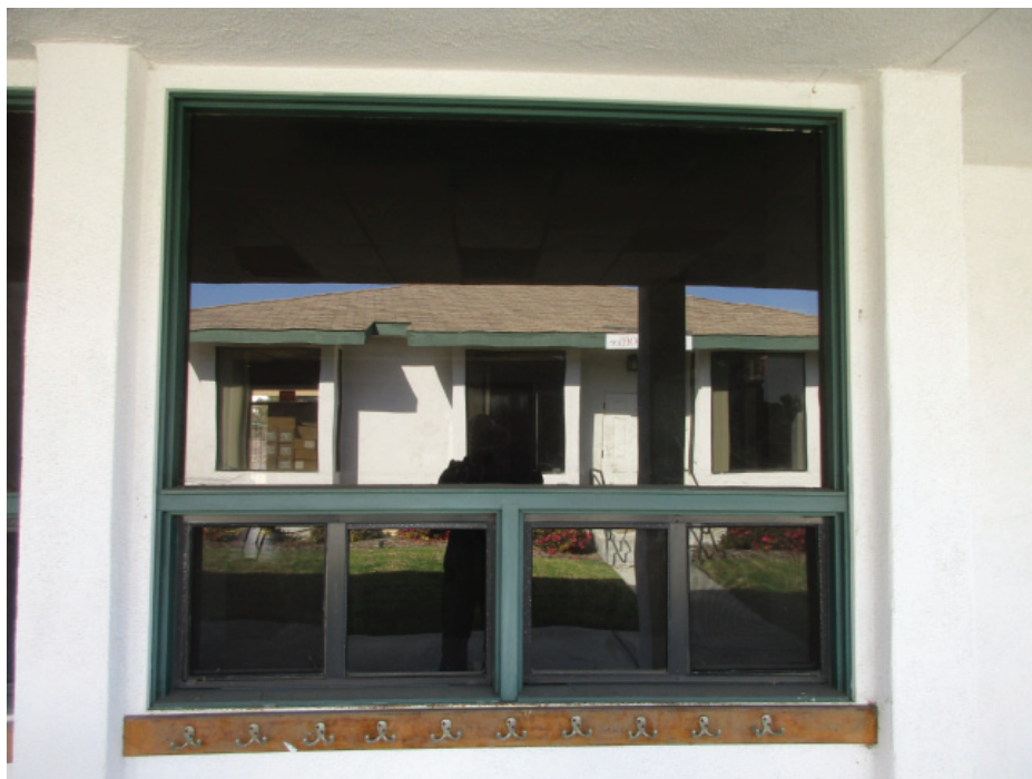
Photo 48: Detail photo showing a typical window configuration at the Preschool consisting of a wood framed fixed window over two aluminum slider windows.
