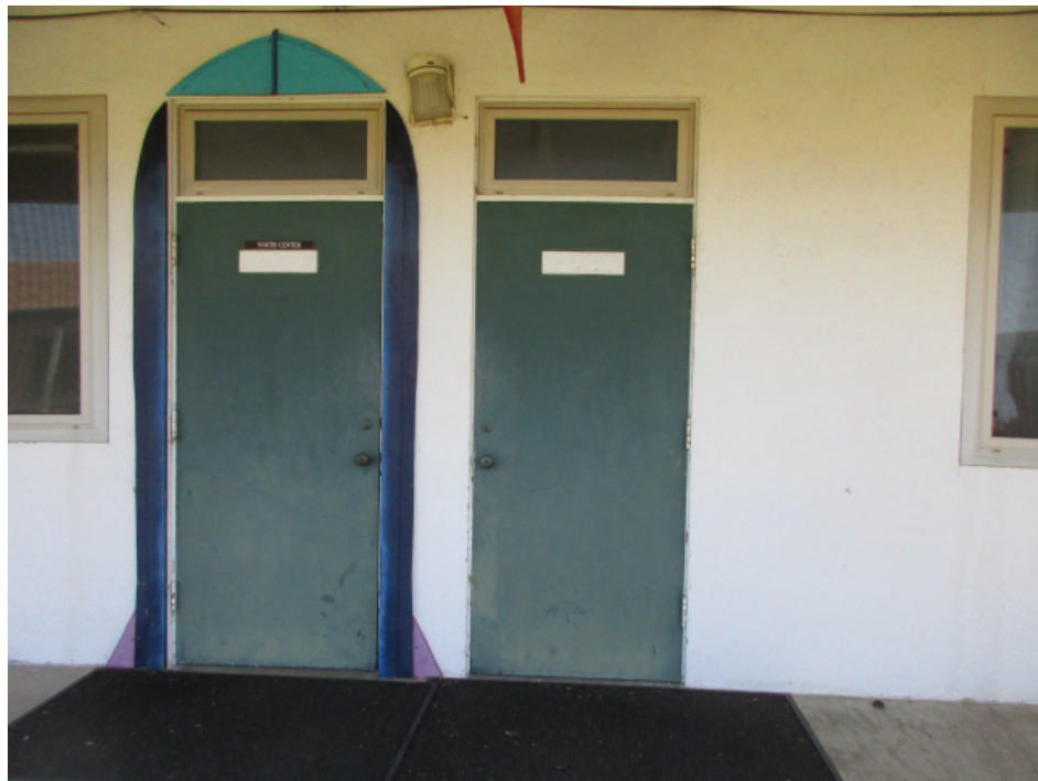
Photo 22: Detail photo showing a typical wood flush door with replacement vinyl transom above at the main Church building.
