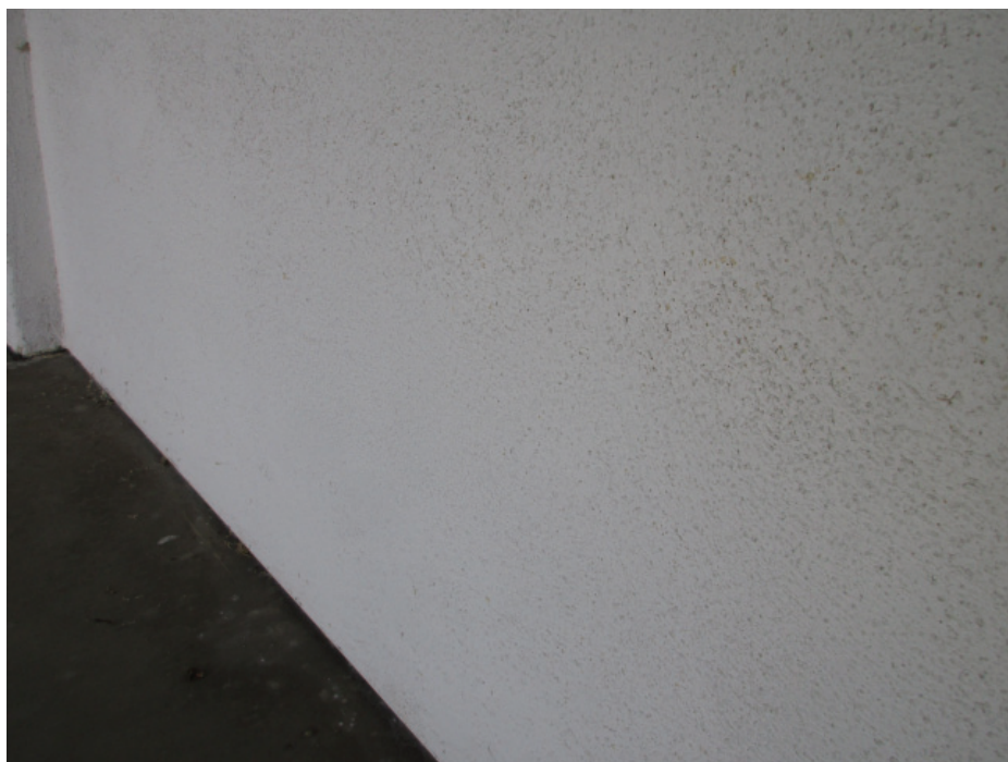
Photo 43: Detail photo showing the rough sand texture stucco finish at the Preschool building.
