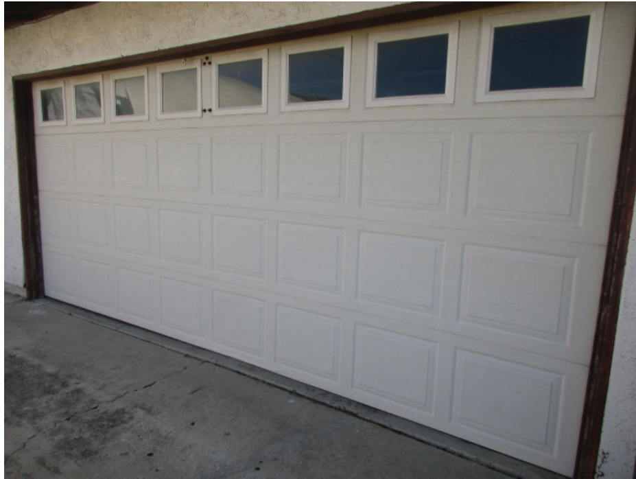
Photo 63: Detail photo showing the contemporary sectional tilt-up garage door.
