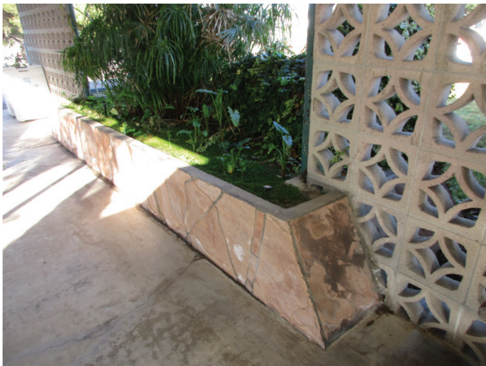
Photo 18: Detail photo showing the cast-in-place concrete planter with flagstone veneer similar to the veneer at the northeast corner of the main Church building.
