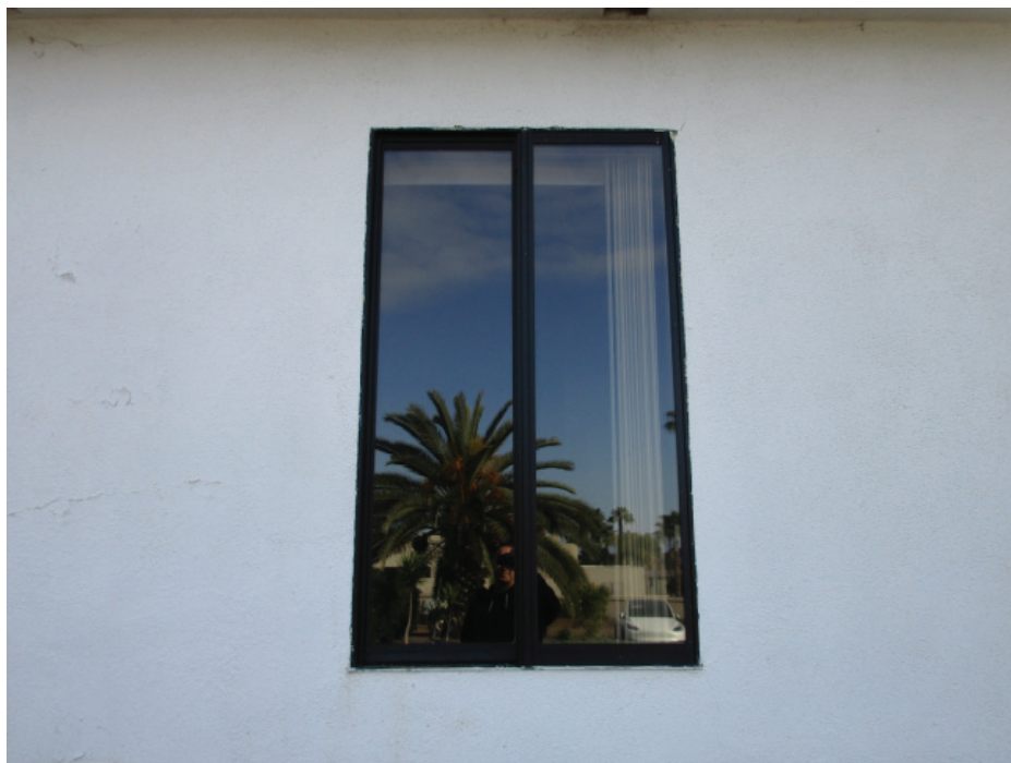
Photo 38: Detail photo showing a non-original aluminum slider window at the west facade of Fellowship Hall.
