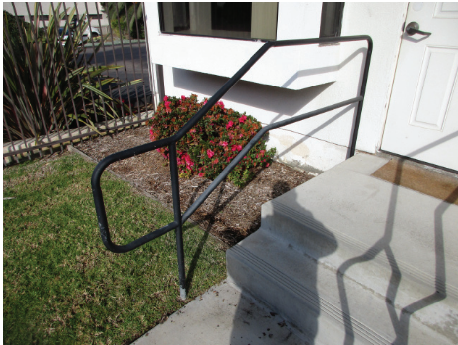
Photo 37: Detail photo showing the non-original cast-in-place concrete stairs and pipe metal railing at the rear facade of Fellowship Hall.
