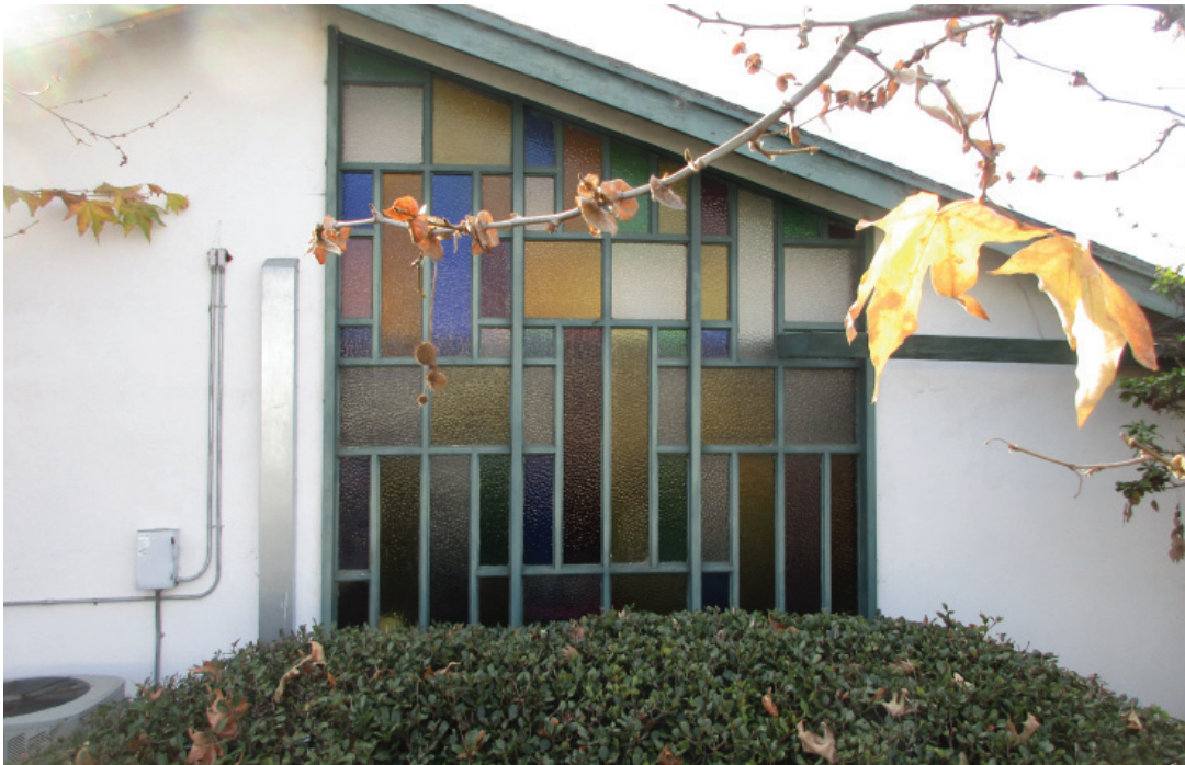
Photo 19: Detail photo showing the wood framed decorative floor-to-ceiling stained glass windows. The feature includes obscure glazing with an irregular wood mullion grid pattern.
