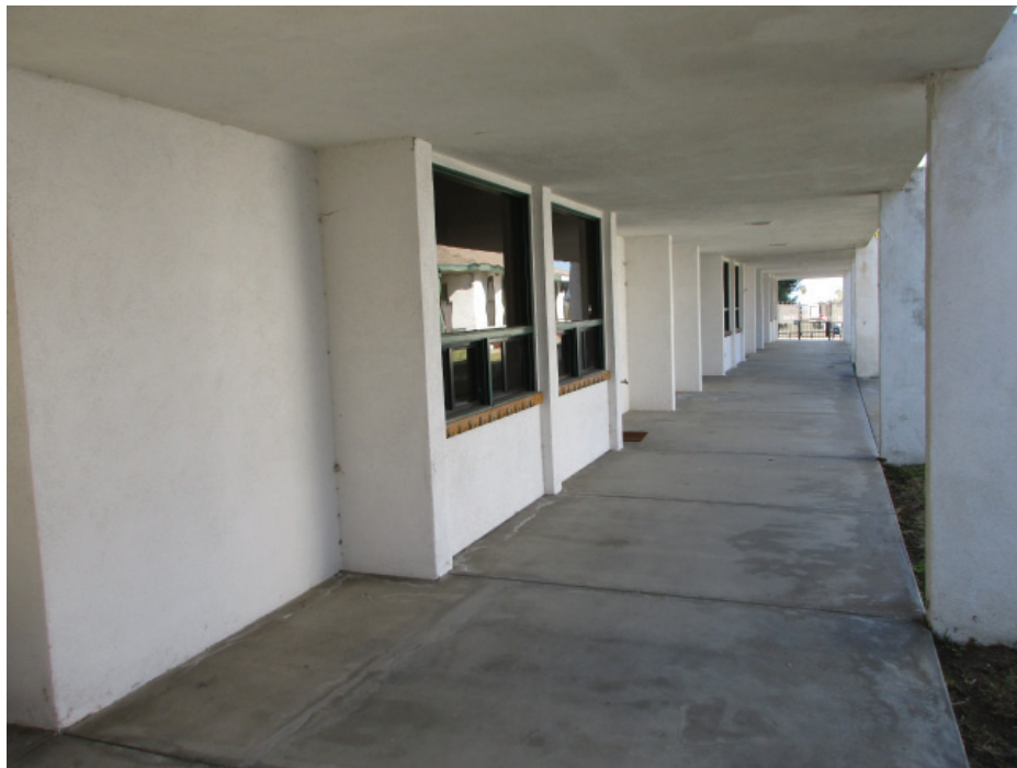
Photo 46: Looking west along the breezway at the north side of the Preschool building showing the enclosed stucco ceiling and columns with cast-in-place concrete walkway.
