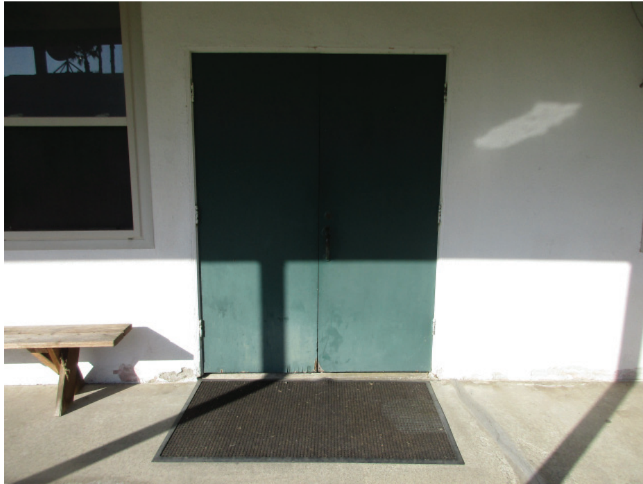
Photo 33: Typical wood flush door at the Fellowship Hall.
