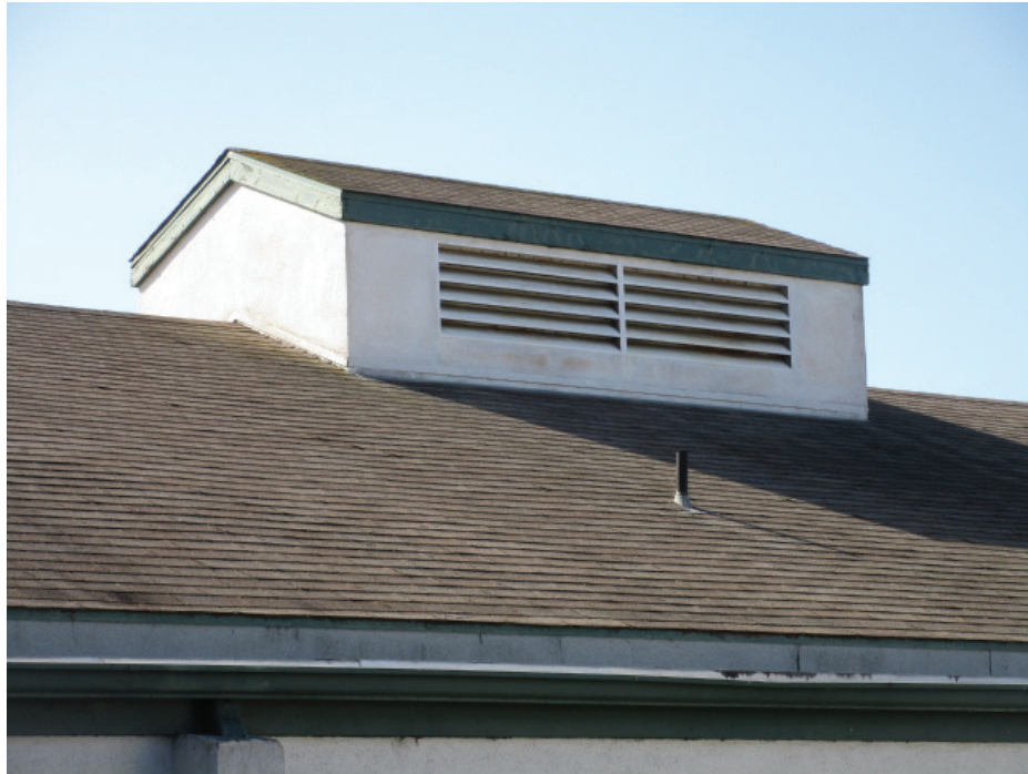
Photo 45: Detail photo showing one of the mechanical penthouses with metal louvers at the north and south sides.
