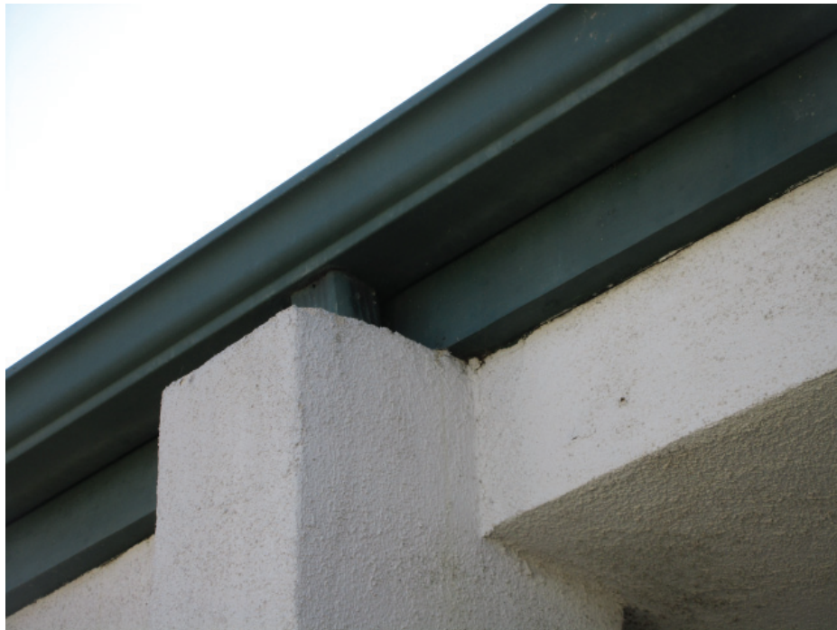
Photo 47: Detail photo showing a typical downspout concealed by a breezeway column.
