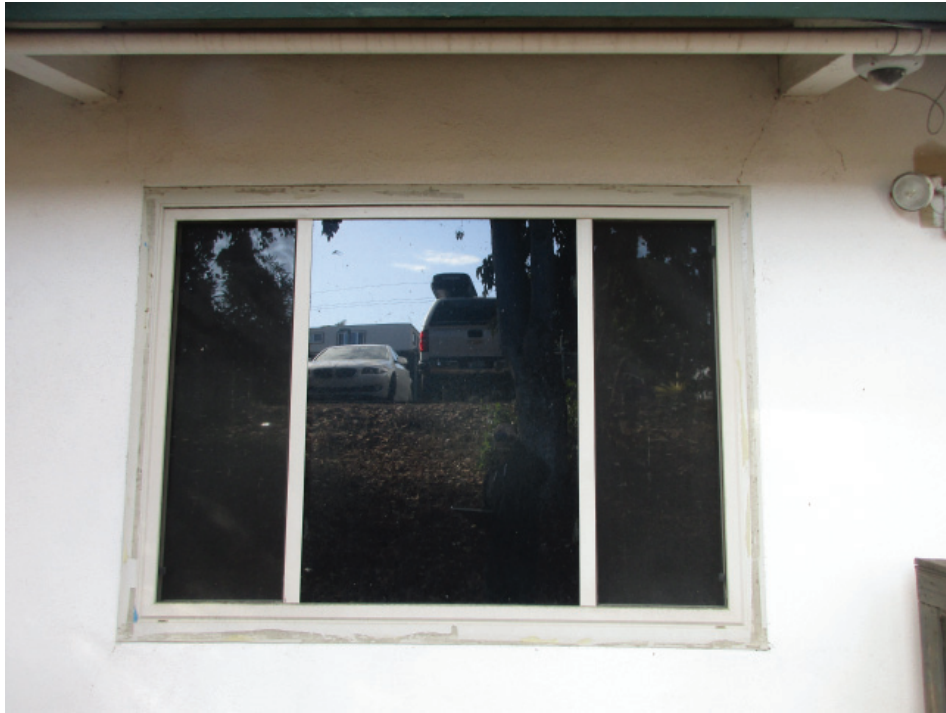
Photo 21: Detail photo showing a typical vinyl replacement window and frame at the main Church building.
