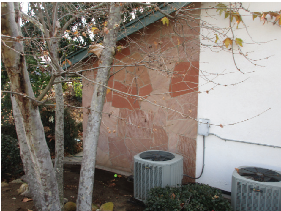
Photo 20: Detail photo showing the flagstone veneer at the northeast corner of the main Church building.
