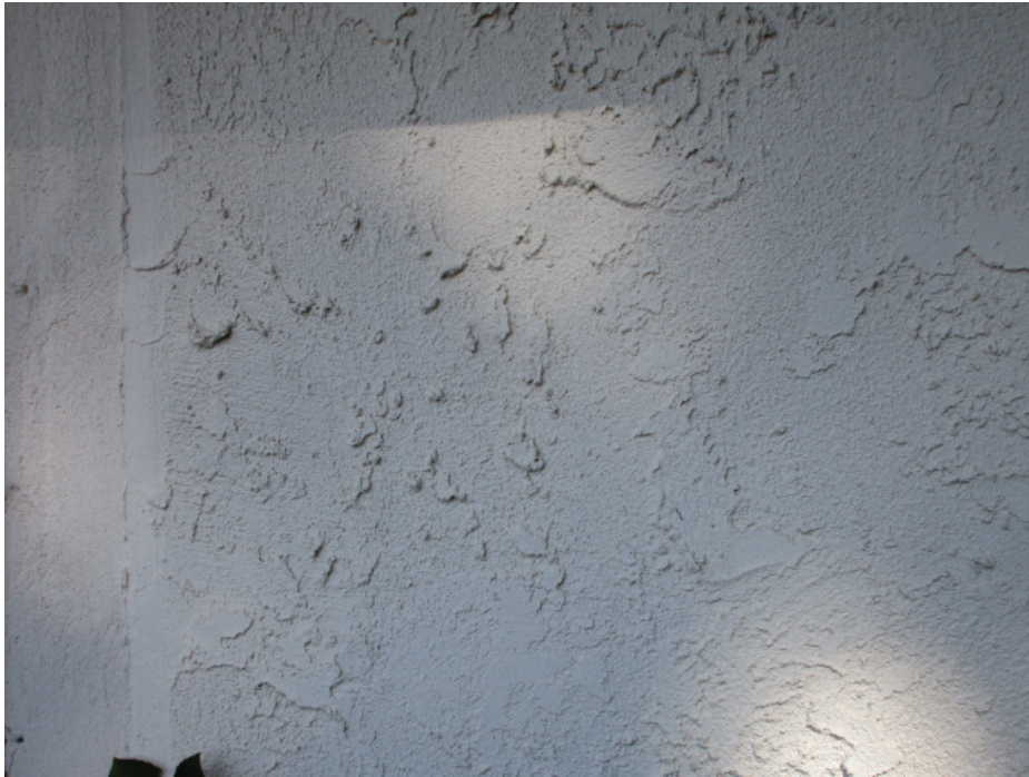
Photo 55: Detail photo showing the heavy-lace textured stucco finish.
