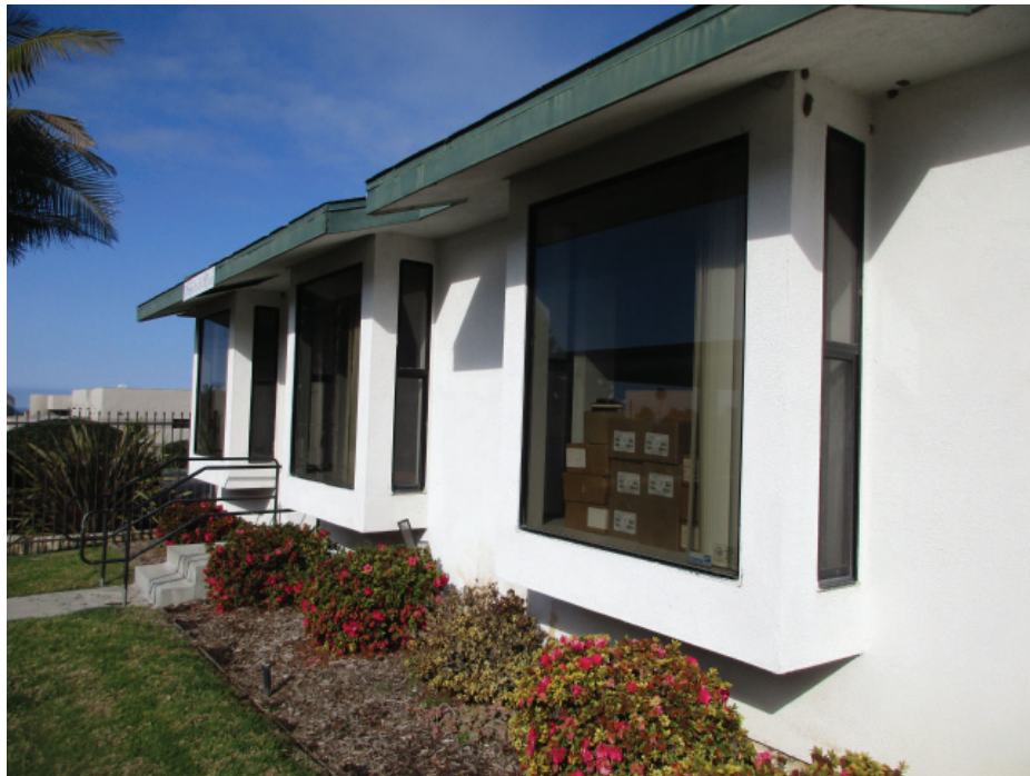
Photo 35: Detail photo showing the stucco finished angled bay windows with fixed and single-hung aluminum windows at the 1989 addition located at the rear of the Fellowship Hall.
