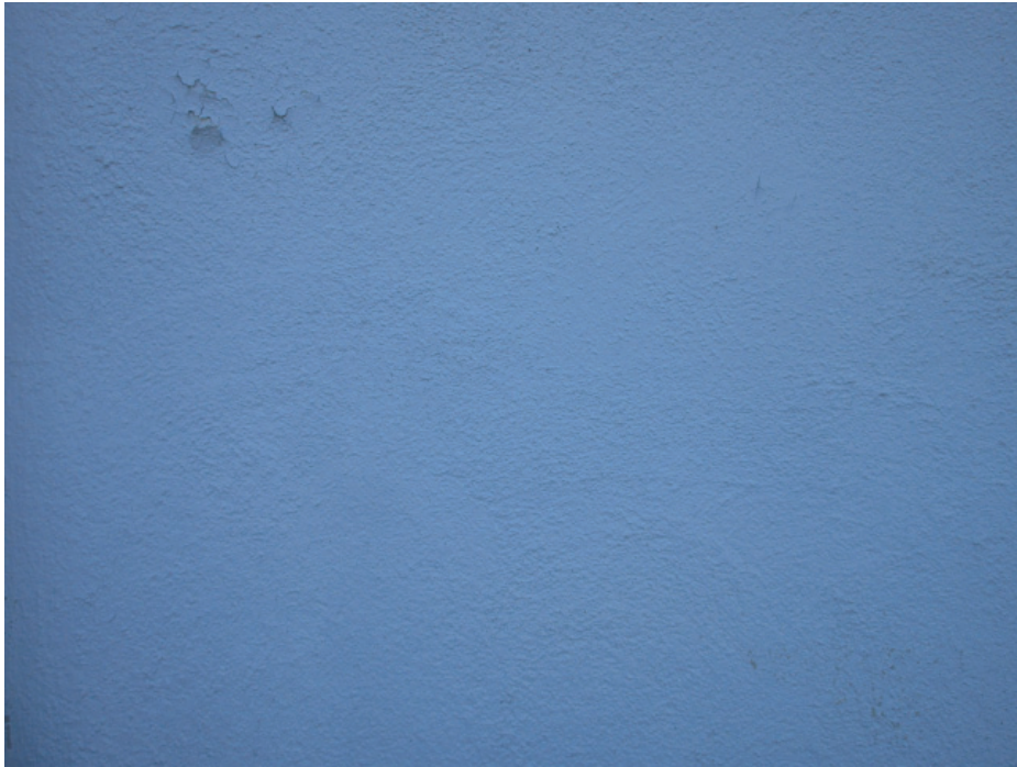
Photo 29: Detail photo showing the smooth sand texture stucco finish.
