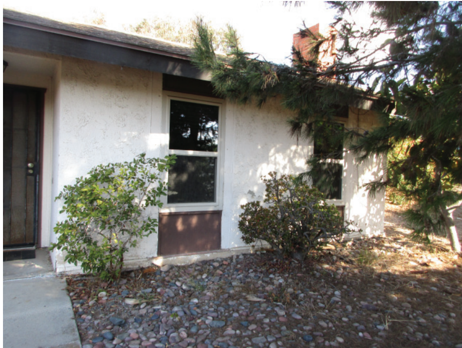
Photo 61: Detail photo showing a typical vinyl replacement window with vertical wood siding at the head and bulkhead of the window.
