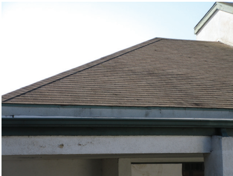
Photo 44: Detail photo showing the asphalt shingle roofing at the Preschool building.
