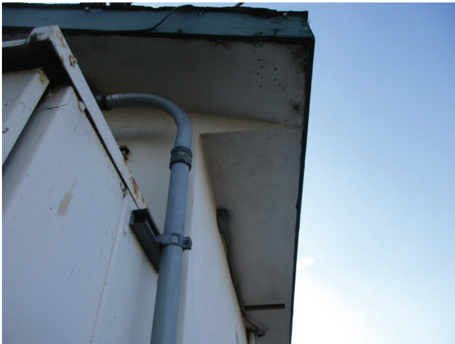
Photo 30: Detail photo showing the enclosed soffit with a smooth sand texture stucco finish.
