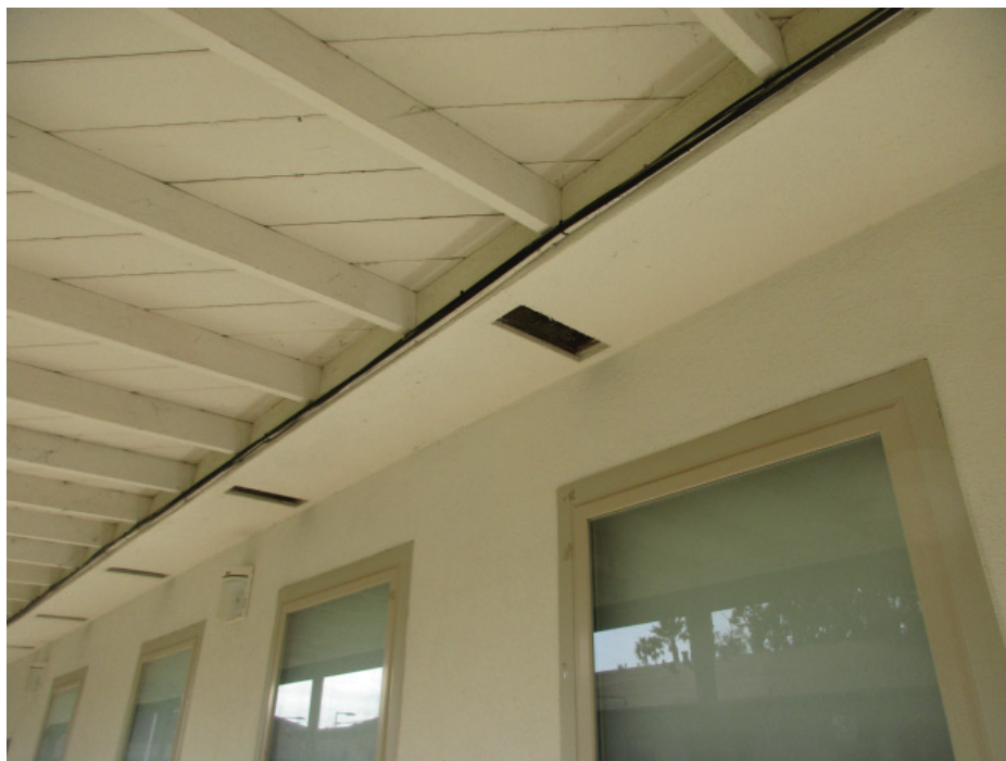
Photo 32: Detail photo showing the interaction between the covered breezeway roof and enclosed soffit at the east facade of the Fellowship Hall building.
