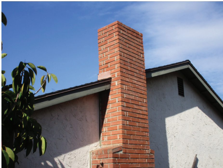
Photo 60: Detail photo showing the non-original brick masonry chimney located at the east facade.
