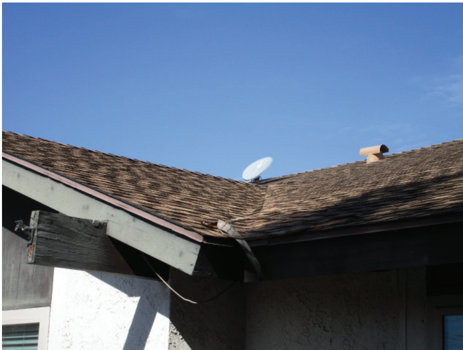
Photo 56: Detail photo showing the replacement asphalt shingle roofing finish.
