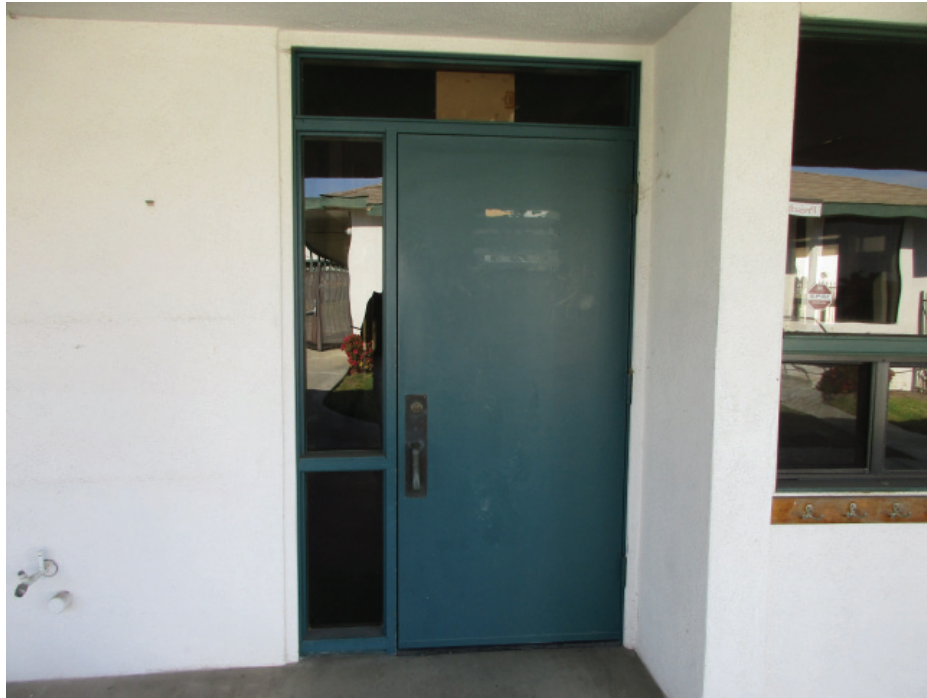
Photo 49: Detail photo showing a typical wood flush door with fixed wood framed sidelite windows and fixed transom windows.
