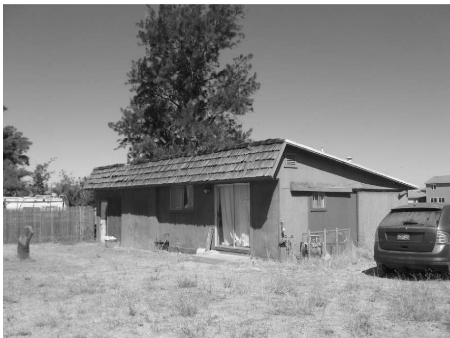
Photo 14: View of smaller unit north of the main residence.
