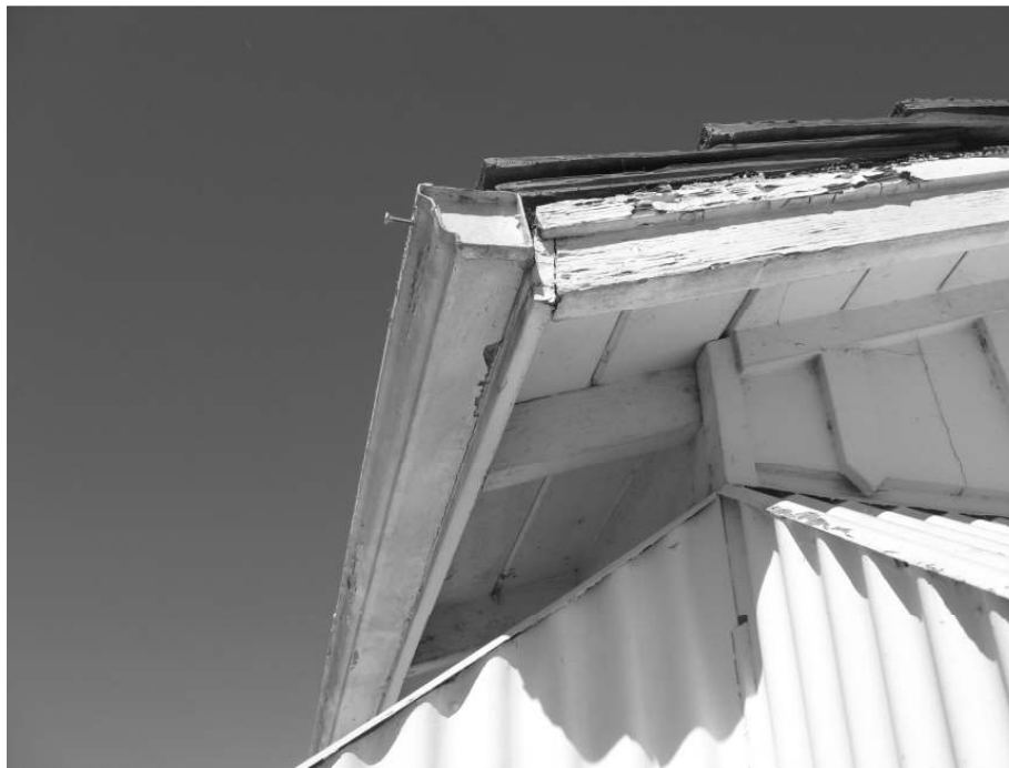
Photo 6: Detail of the open eaves with exposed rafters.
