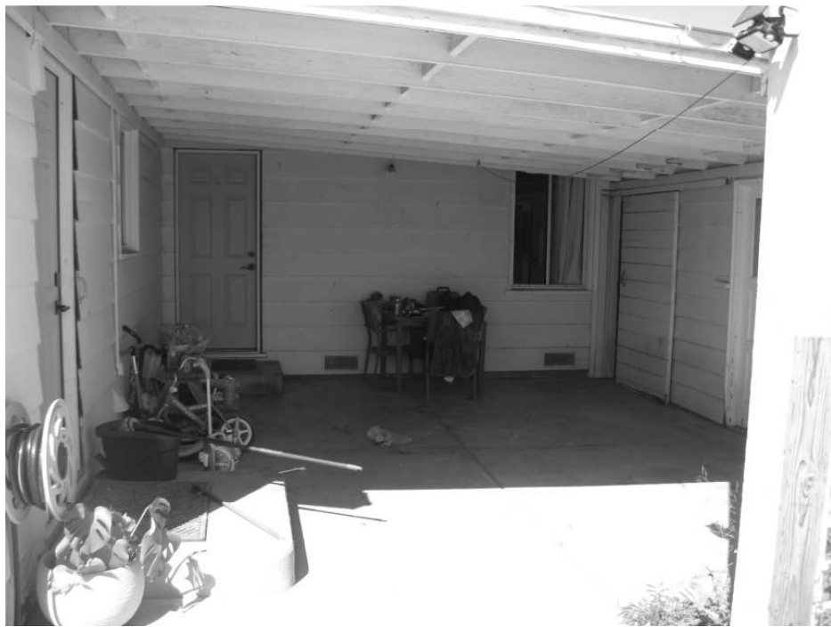
Photo 3: View of the covered entry adjacent to the garage.
