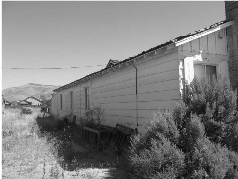
Photo 9: View along the rear (western) façade.
