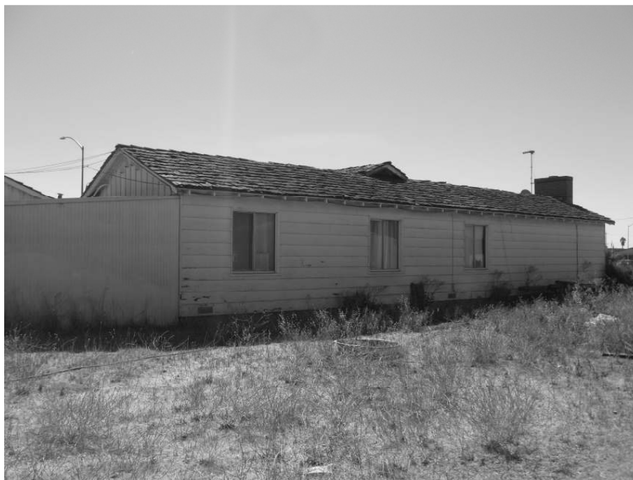
Photo 10: Oblique view of the rear façade.
