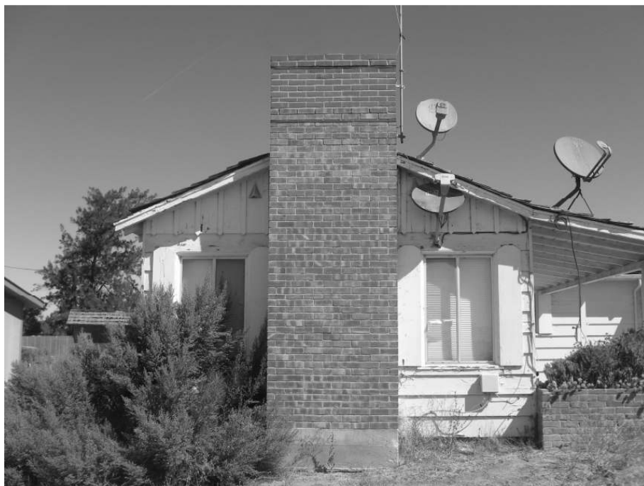
Photo 8: View of the southern façade showing brick chimney.
