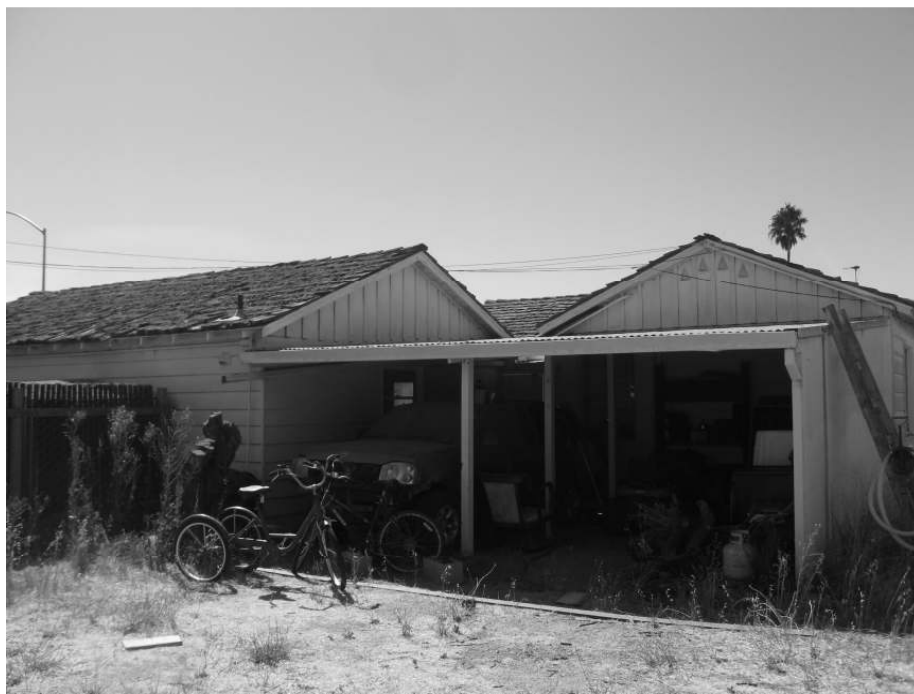
Photo 12: View of the northern façade showing carport addition.
