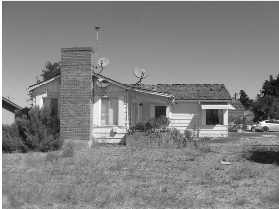
Photo 7: View of the southern façade of the residence.
