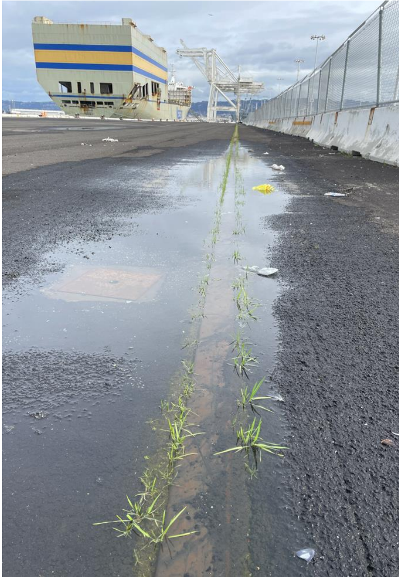
Figure 2-6 Typical Submerged Landside Crane Rail
