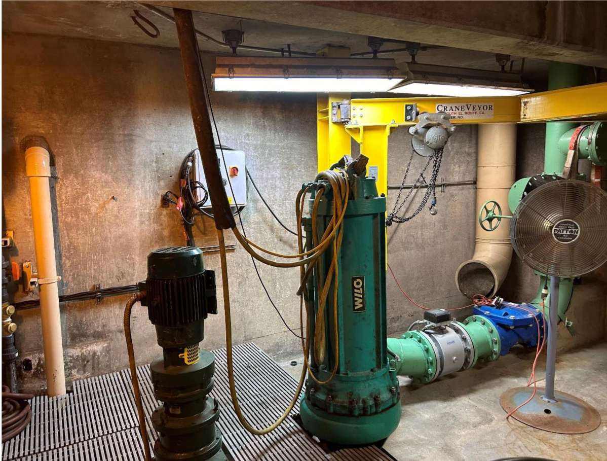
Photograph 12 View of Lower Subterranean Level of ACLS, with Grate over Suction Pipe, Gate Valve, Grinder, and Motor (Left) and Check Valve (Background Right), Facing East
