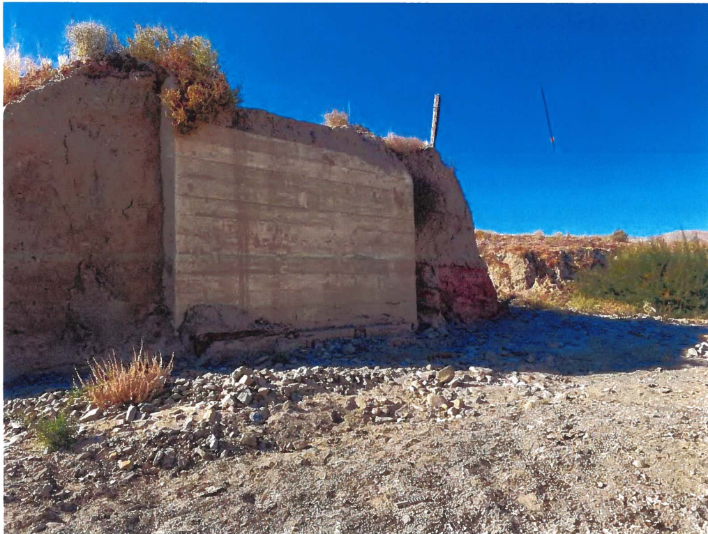
IMG_9391, view northwest, 10/30/2023, concrete retaining wall under western approach to crossing.
