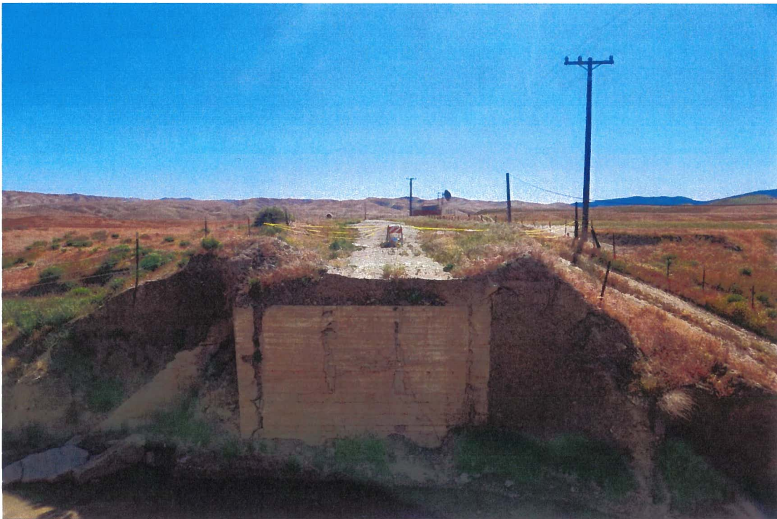
Figure 6. Photograph of New Idria Road at the bridge washout over Larios Creek.
