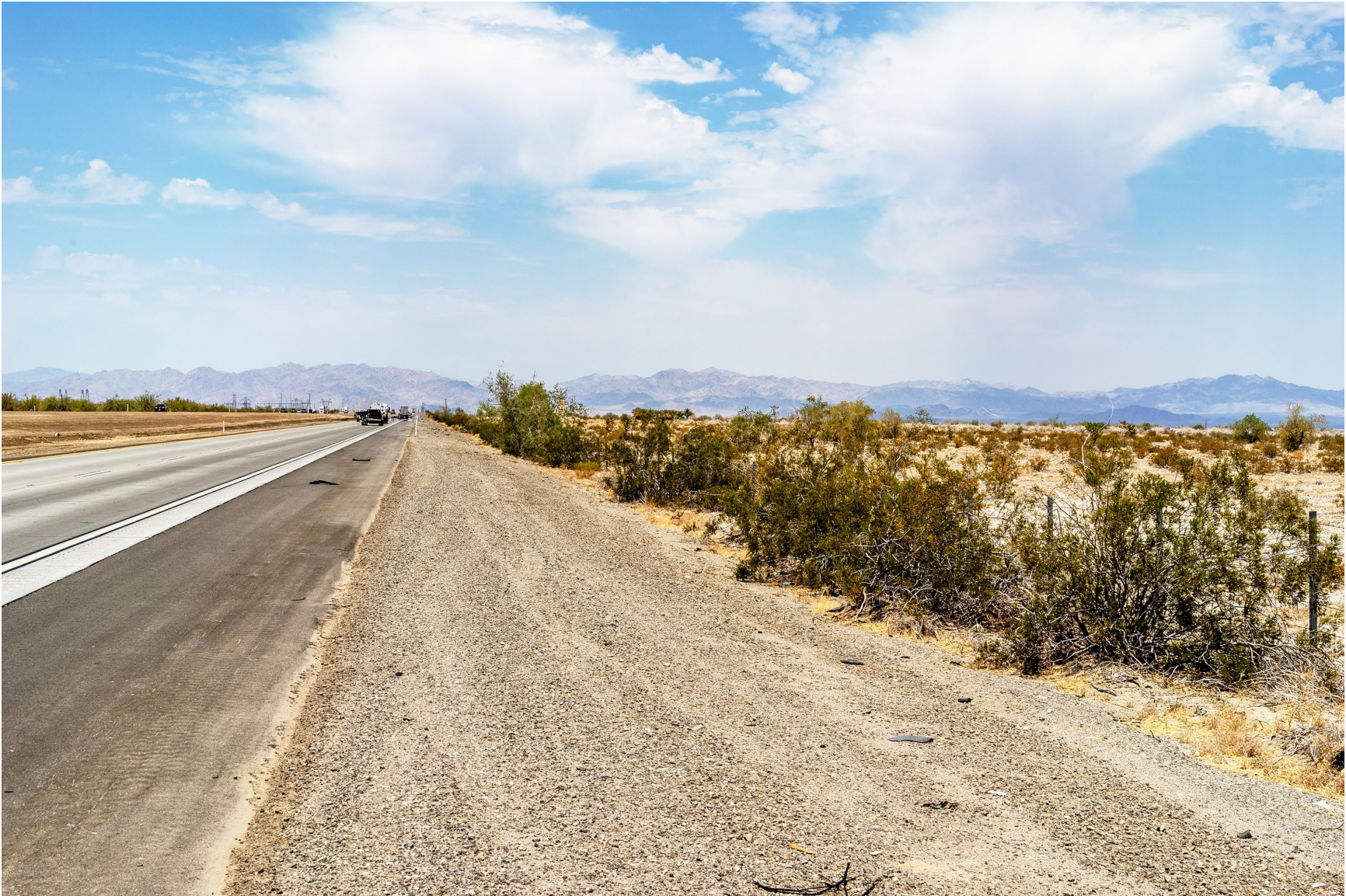
Figure 3.2-4 KOP 7 – I-10 (Westbound)
