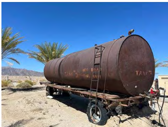
Photo #17 View of diesel AST in the water pump area.
