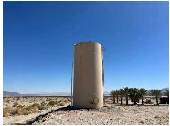
Photo #14 View of a water AST on the southwestern tract in the water pump area.
