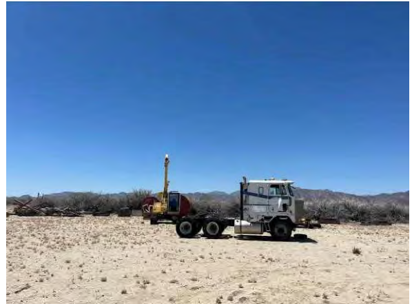
Photo #20 View of construction machinery in the central portion of the southwestern tract.
