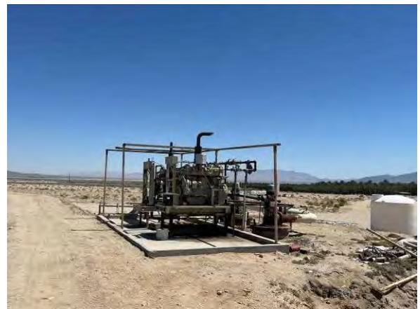
Photo #4 View of the water well located adjacent to the retention pond.
