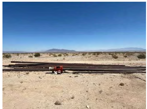
Photo #18 View of piping equipment in the water pump area.
