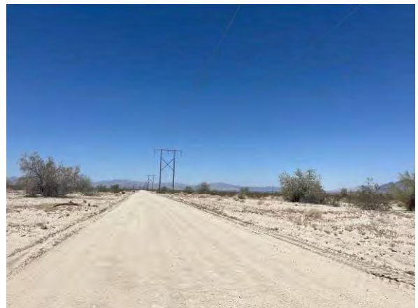
Photo #28 View of the proposed gen-tie route west of the northern tract, along the pre-existing gen-tie line.
