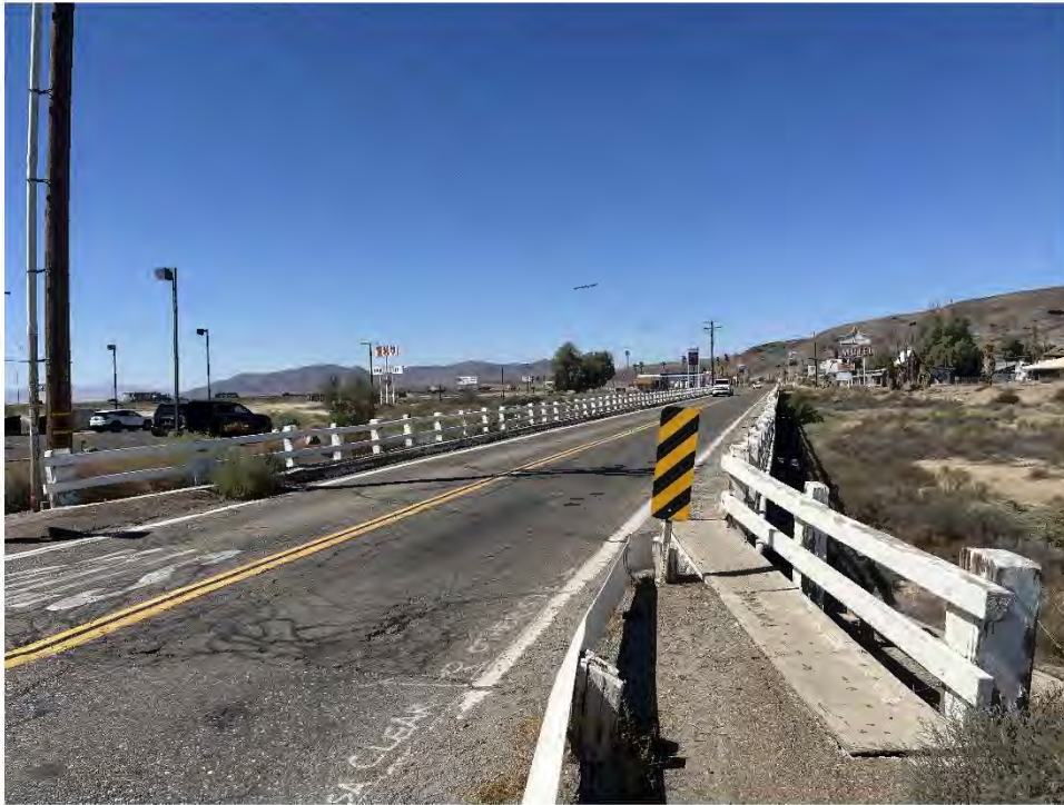
Photo 1. Representative photo of the existing Baker Boulevard Bridge (urban/barren land cover) as it crosses over the Mojave River Channel. Taken facing southwest (8/14/2024).
