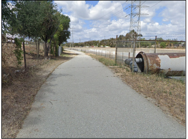
Figure 7 - Narrowed service road at the 60-in pipe bridge
