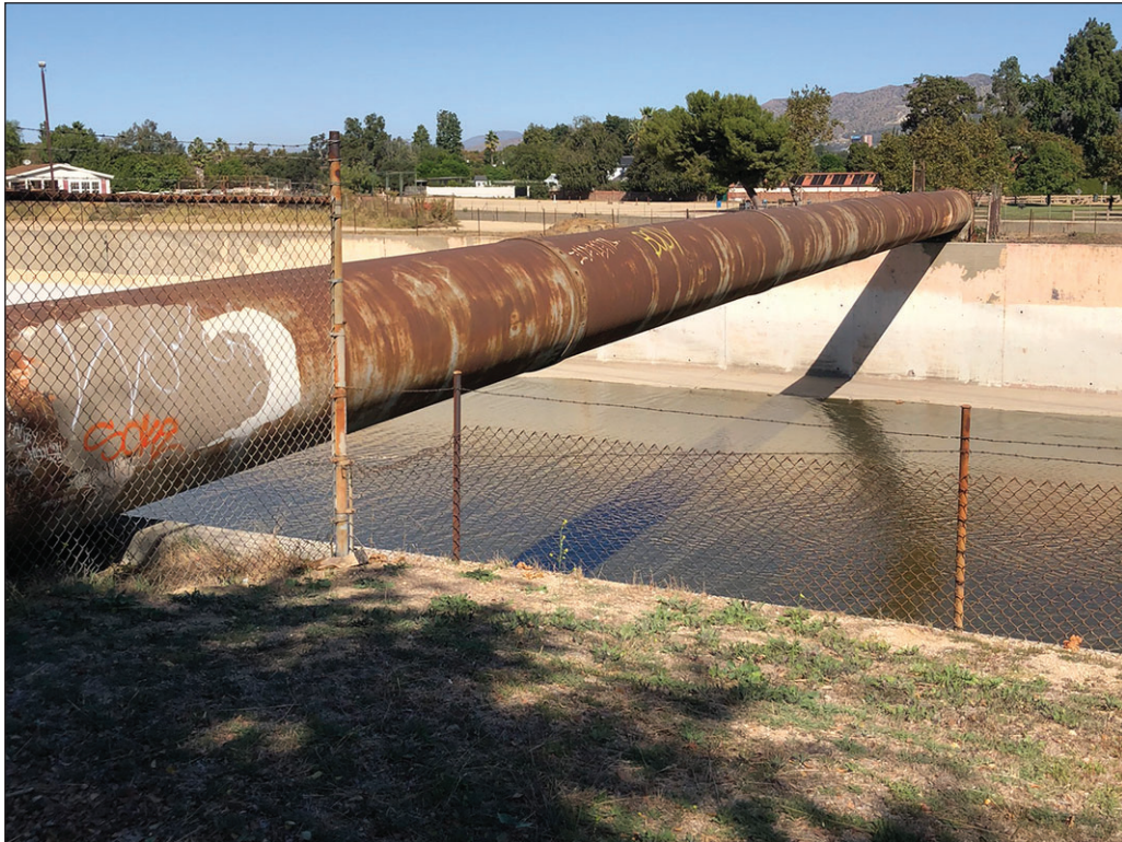
PHOTOGRAPH 6: View of the existing water/sewer pipeline crossing northward from the Project alignment.
