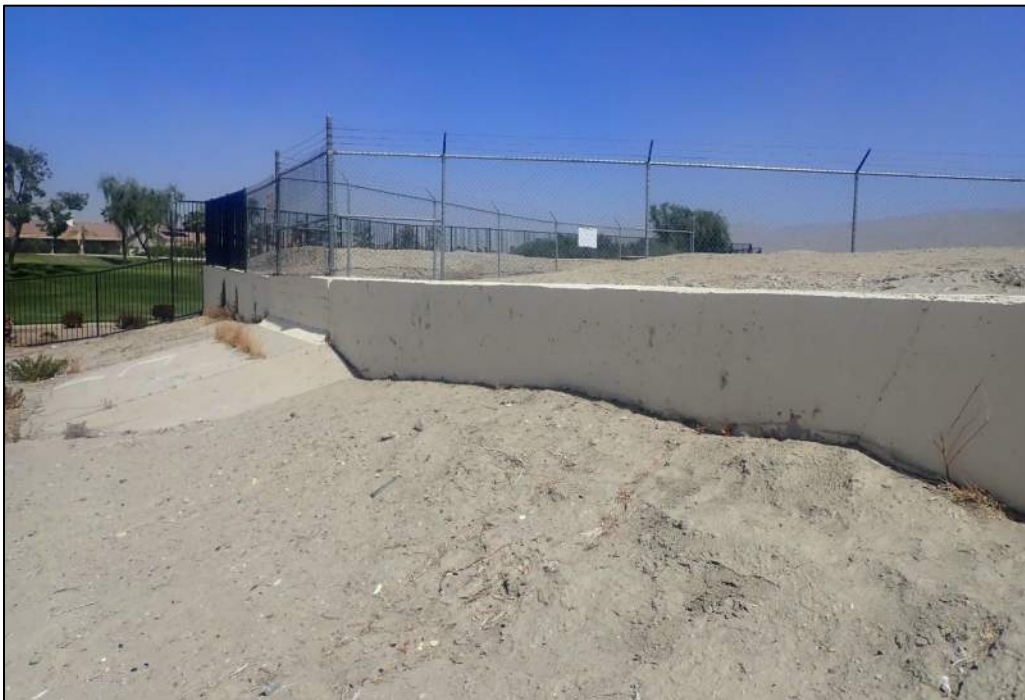
Figure 31. Closeup of concrete wall at edge of Thousand Palms Channel where siphon travels underground, and security fence.
