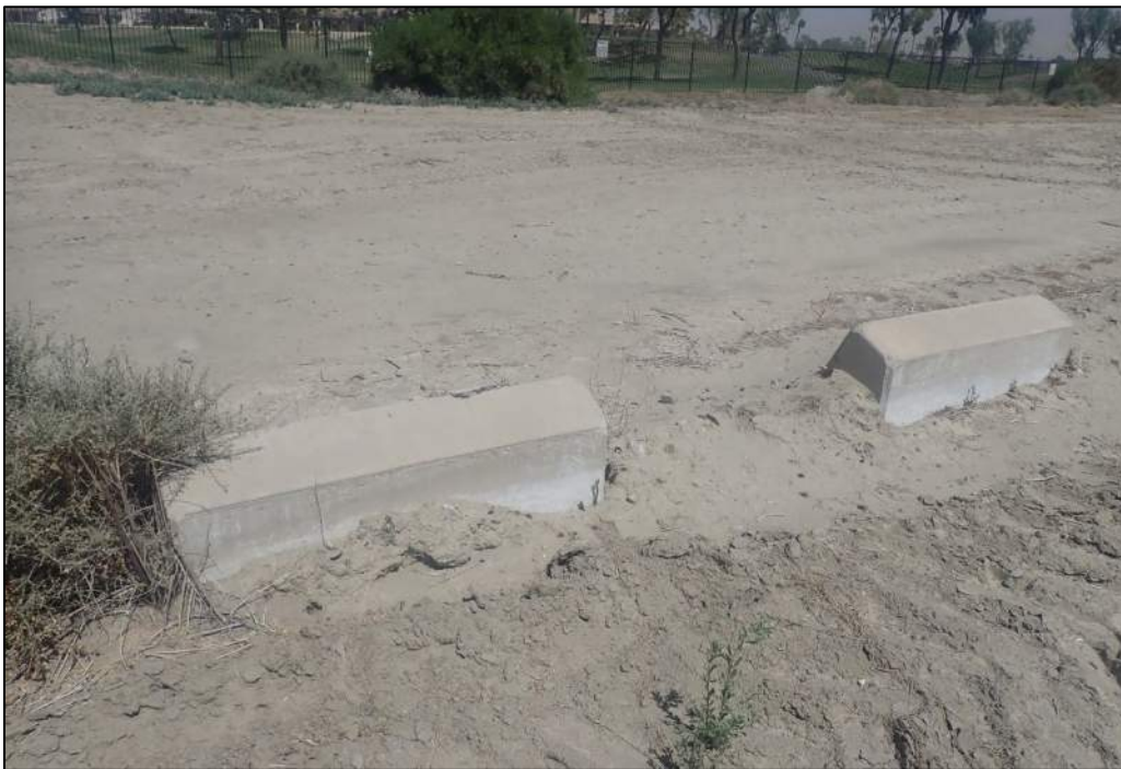
Figure 36. Closeup of concrete blocks or baffles of the drop structure.
