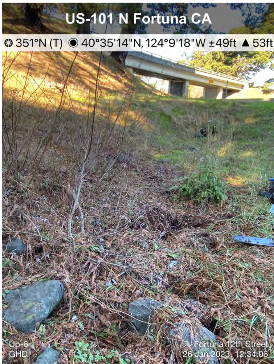
Photo 10. Location of Upland 6 in boulder filled swale with culvert.
