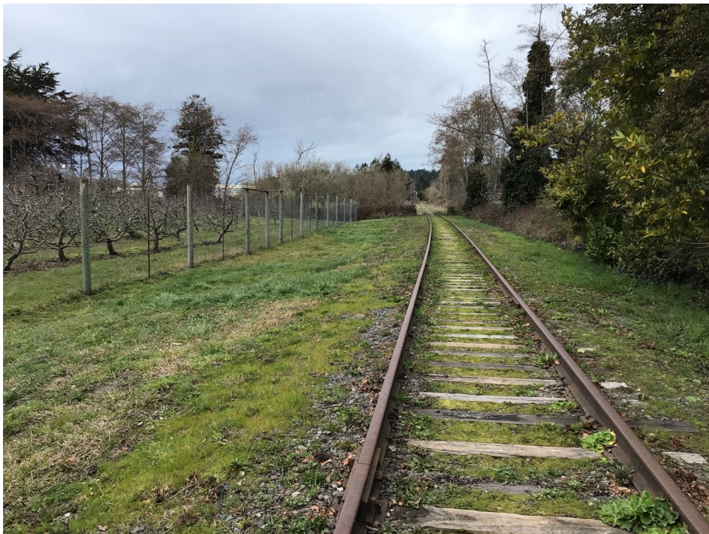
Photo C-5. Railroad tracks with mowed grasses northeast of the Newburg road and 12 th Street intersection.
