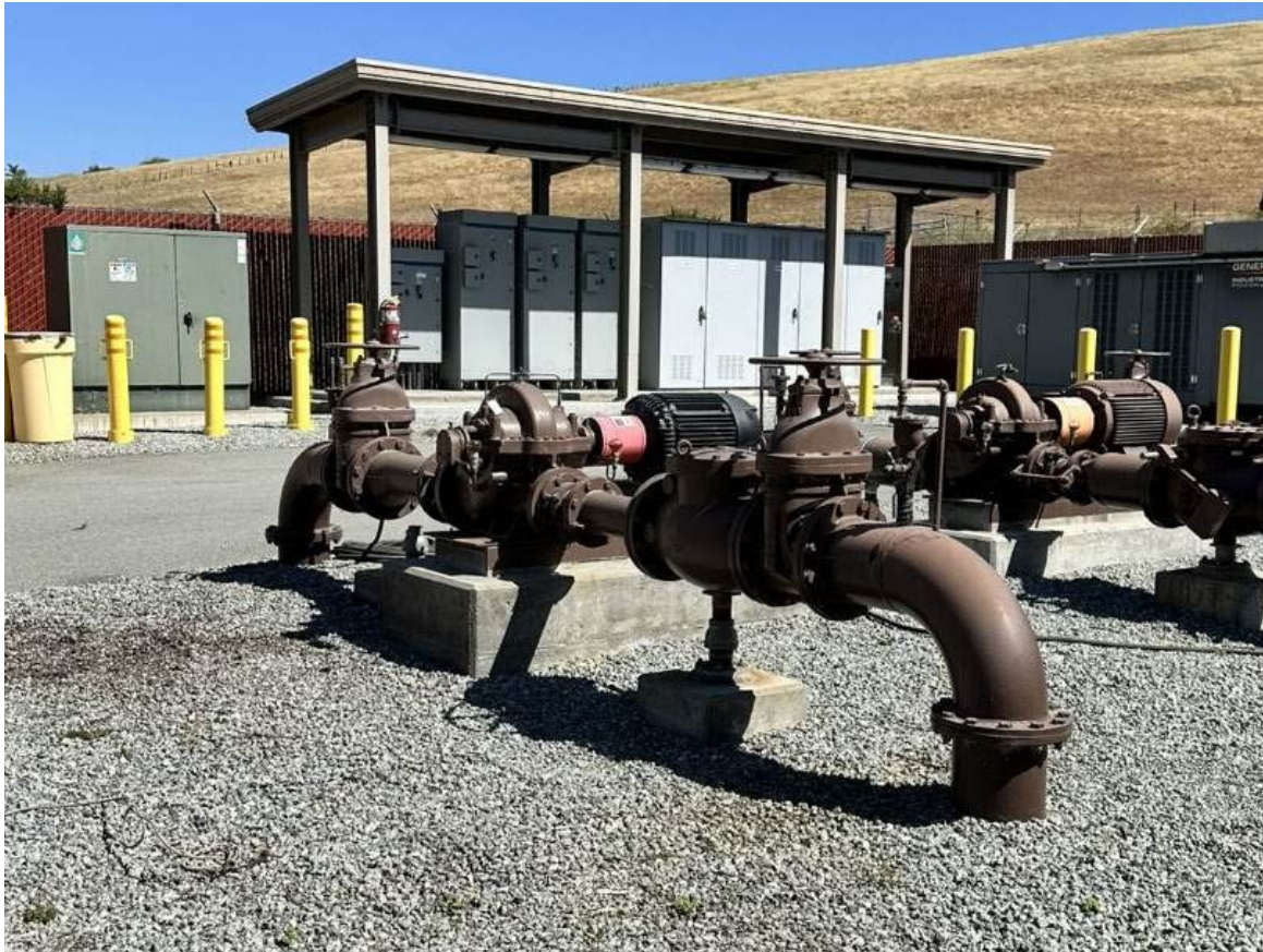
Figure 2-3: 2.25 MGD Raw Water Pump Added to the Existing Raw Water Pump Station (RWPS)
