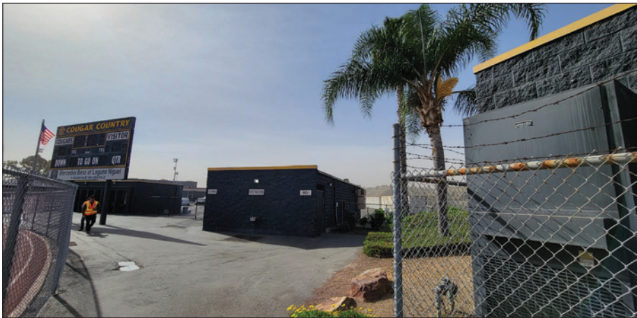
③ From the western end the track and field, looking southwest at the snack shop building, the San Diego Gas and Electric building, the restroom building, a flagpole, a scoreboard, and landscaping on the project site.
