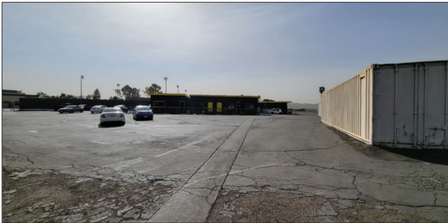
① From the northern end of parking lot #1-C, looking south at parking lot #1-C, and storage containers on the project site and the athletic-related portable classrooms in the distance.
