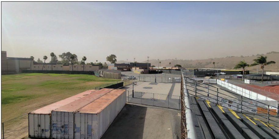
⑦ From the southern end of the home bleachers on the project site, looking southwest at the storage containers, two basketball courts, fencing, and gates on the project site.
