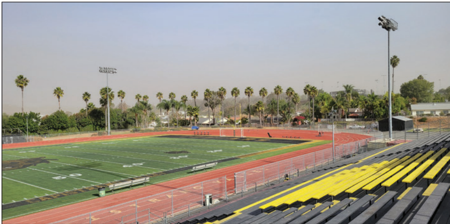
⑥ From the southern end of the home bleachers on the project site, looking north of at the home bleachers, the track and field, stadium lighting, and PA system on the project site.
