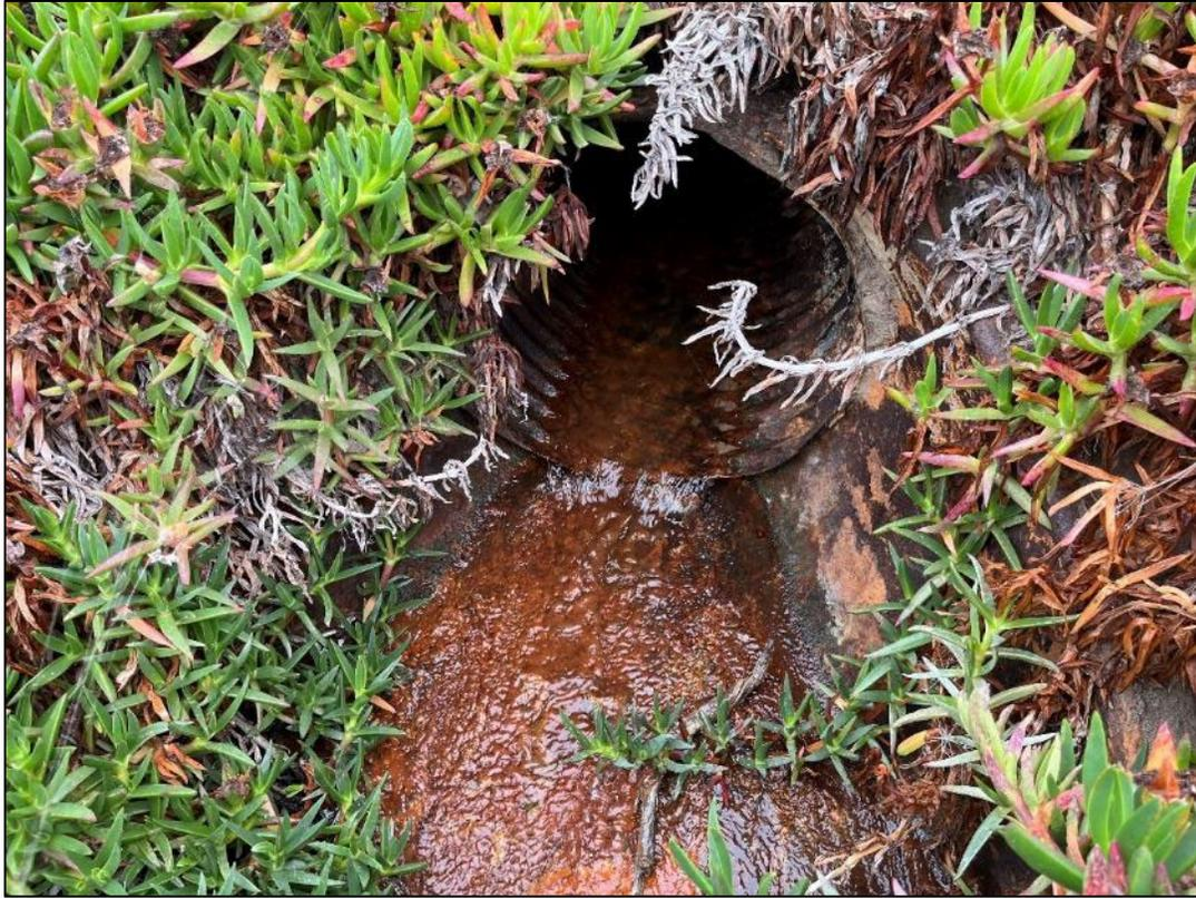
**Figure 4-12.** Outflow from culvert 9 into engineered channel on the west side of Coast Road during flushing.
