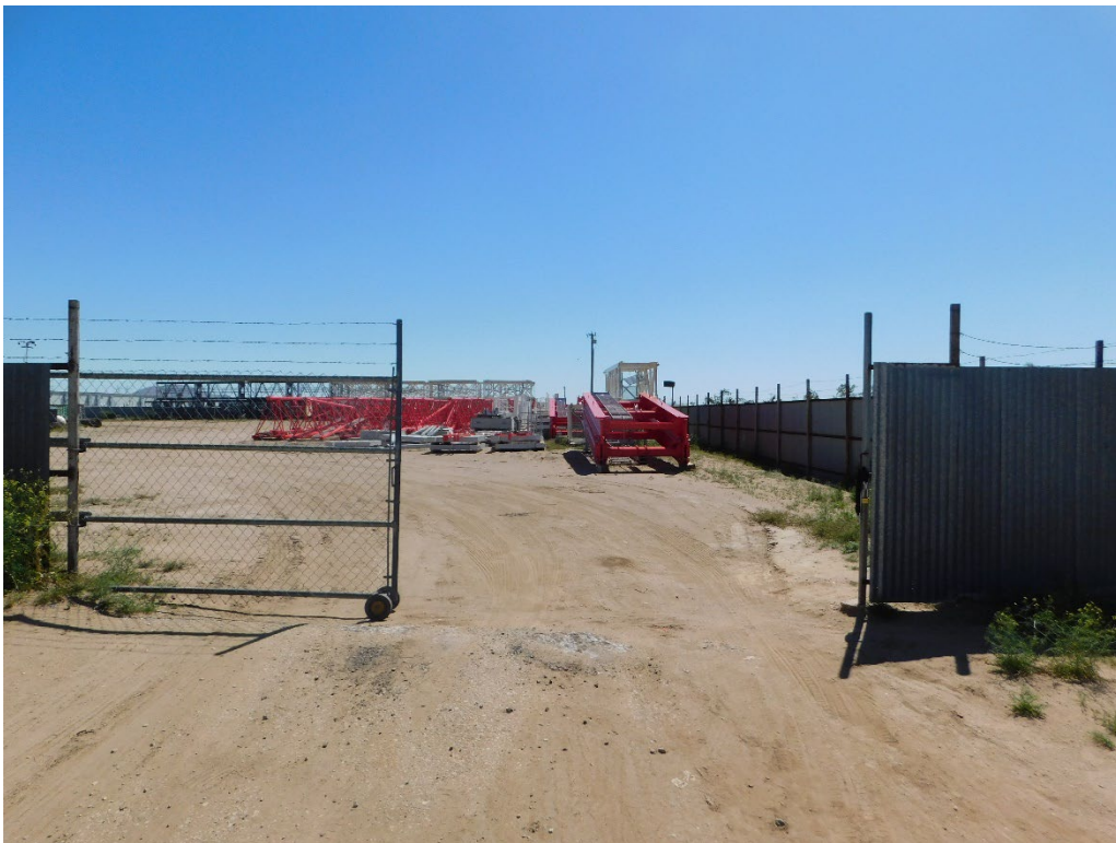
Photograph 2: Depicting the gated entry and perimeter fencing, separating the project site from the surrounding area.
