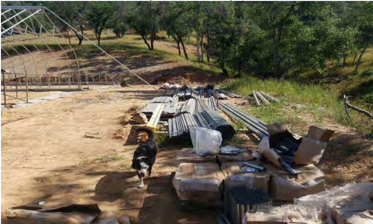
Photograph 14. Staged material for greenhouse construction. Coordinates: 37.51471 °N, -120.01556 °W facing northwest. Photo taken by Mattole Whitaker on May 17, 2023.
