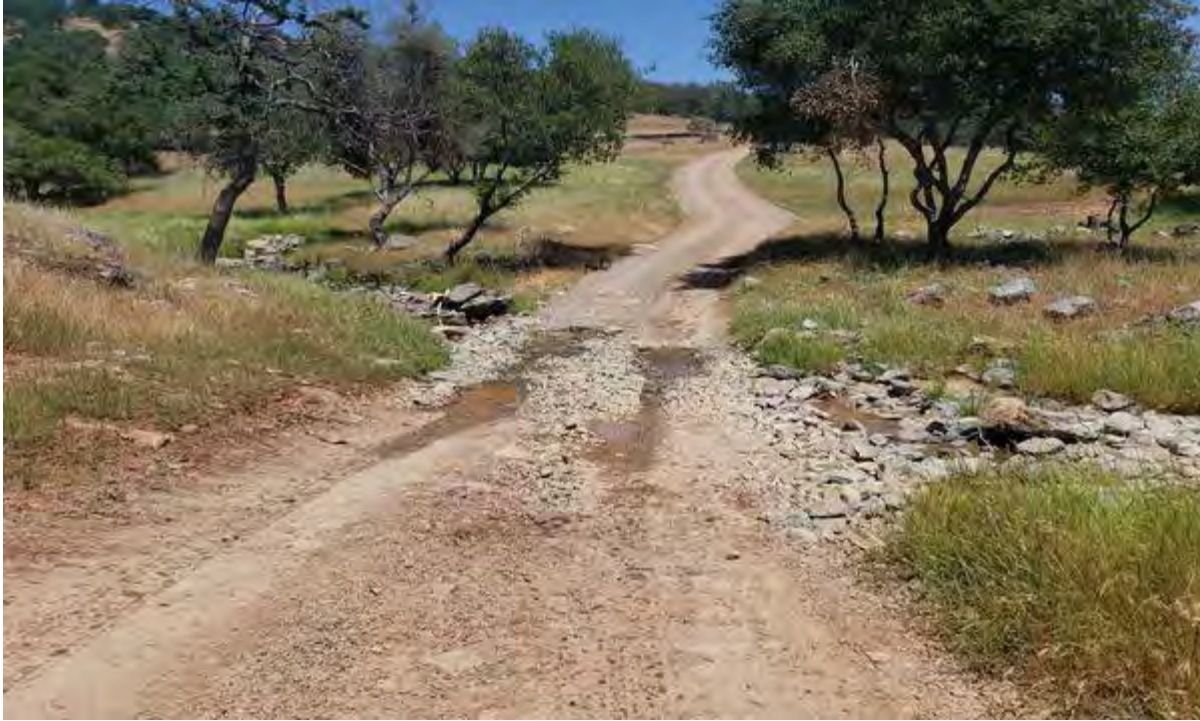
Photograph 24. Main road going through Agua Fria Creek, culverts are to be installed. Coordinates: 37.51494 °N, -120.02855 °W facing northwest. Photo taken by Mattole Whitaker on May 17, 2023.
