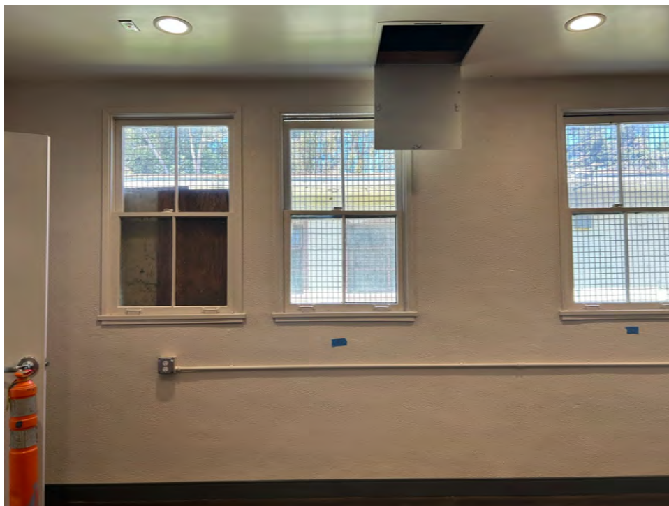
Photo 6. View of interior of Warehouse, view of personnel side of building. Note original, double hung, sash windows.
