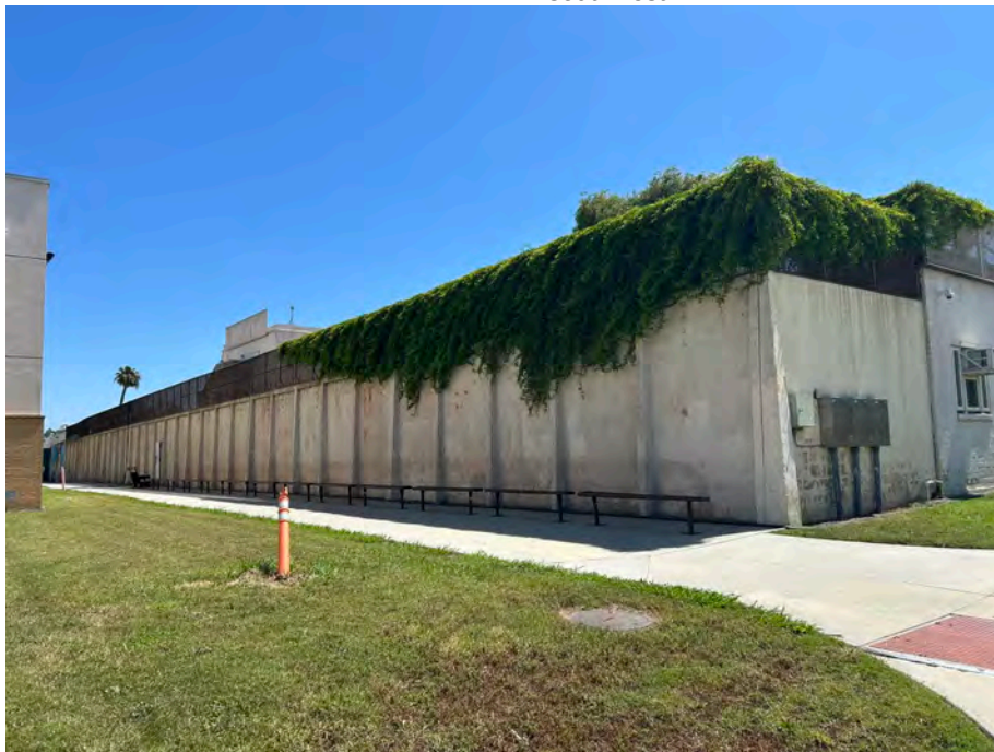
Image 2. View from interior of Central Juvenile Hall Campus, example of 15-foot concrete walls that surround the facility. View toward northeast.
