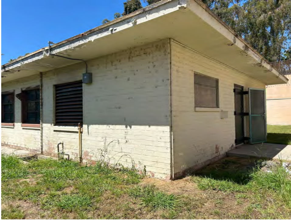
Photo 5. Side end of the building, with windows visible and vents for the “X” room visible. View toward northwest.
