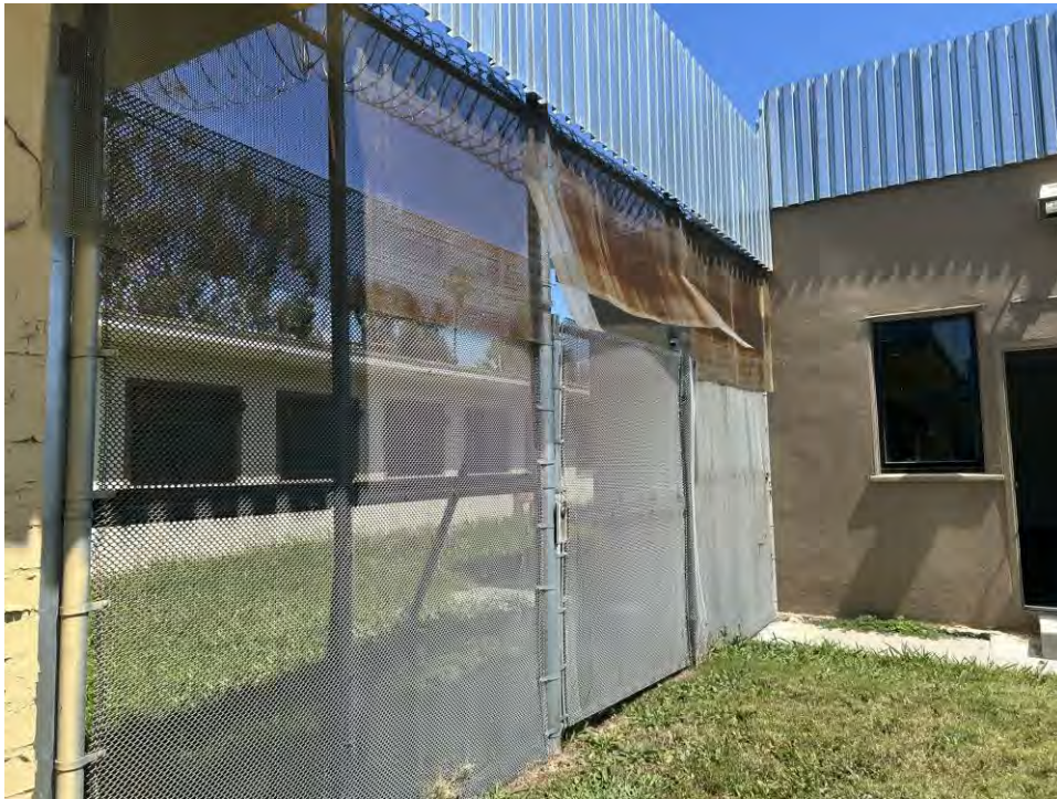
Figure 47. Detail of entrance to Warehouse building, with gate visible and Boys Maximum Security Unit in background. View toward northeast.
