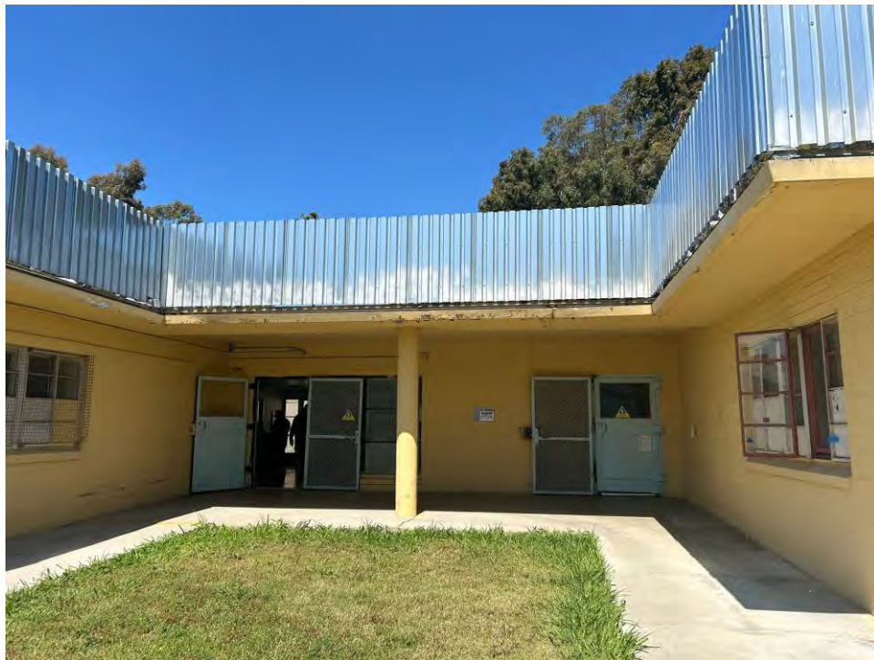
Figure 27. Primary façade dual entrance space. View toward northwest.
