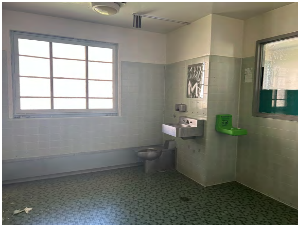
Photo 10. View of toilet and shower room. View toward north.
