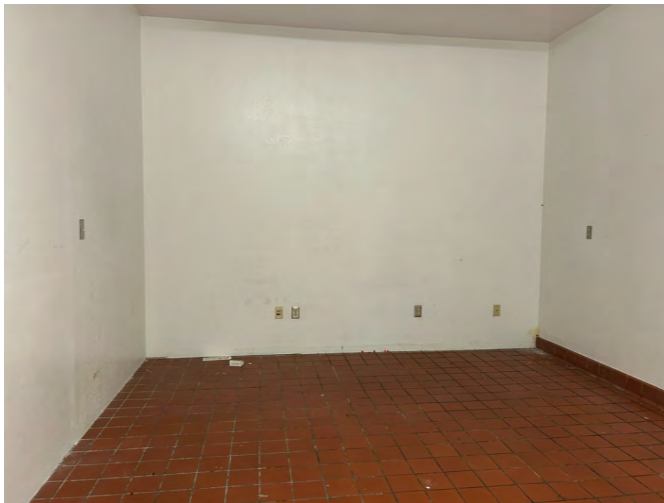
Photo 3. Interior of Mess Hall, view of old kitchen/food preparatory area. View toward northwest.
