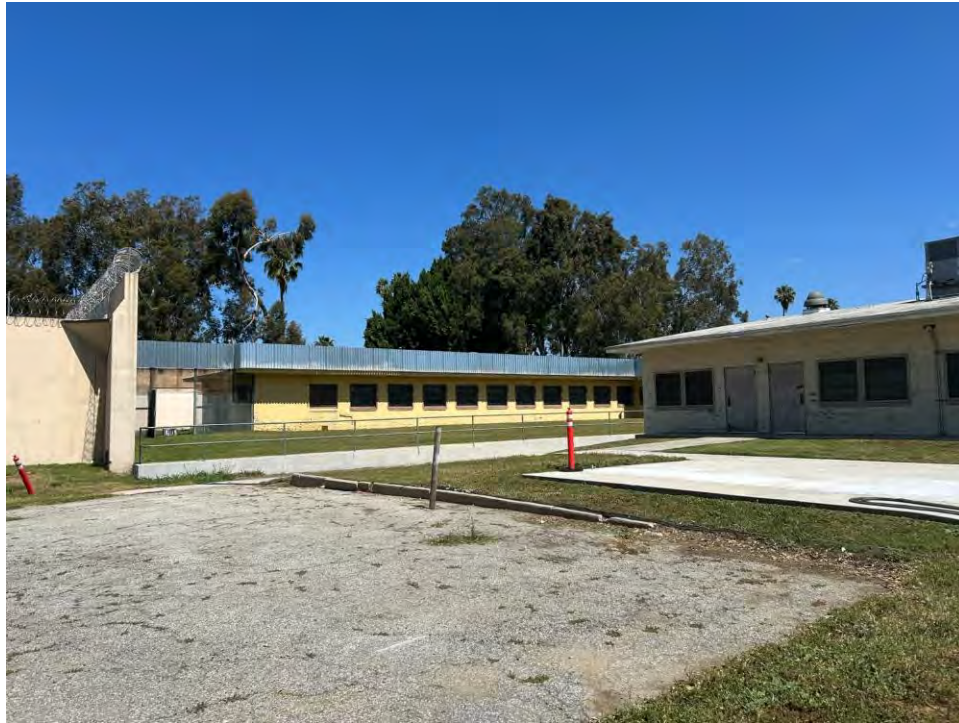
Figure 24. Boys Maximum Security Unit. View toward north.
