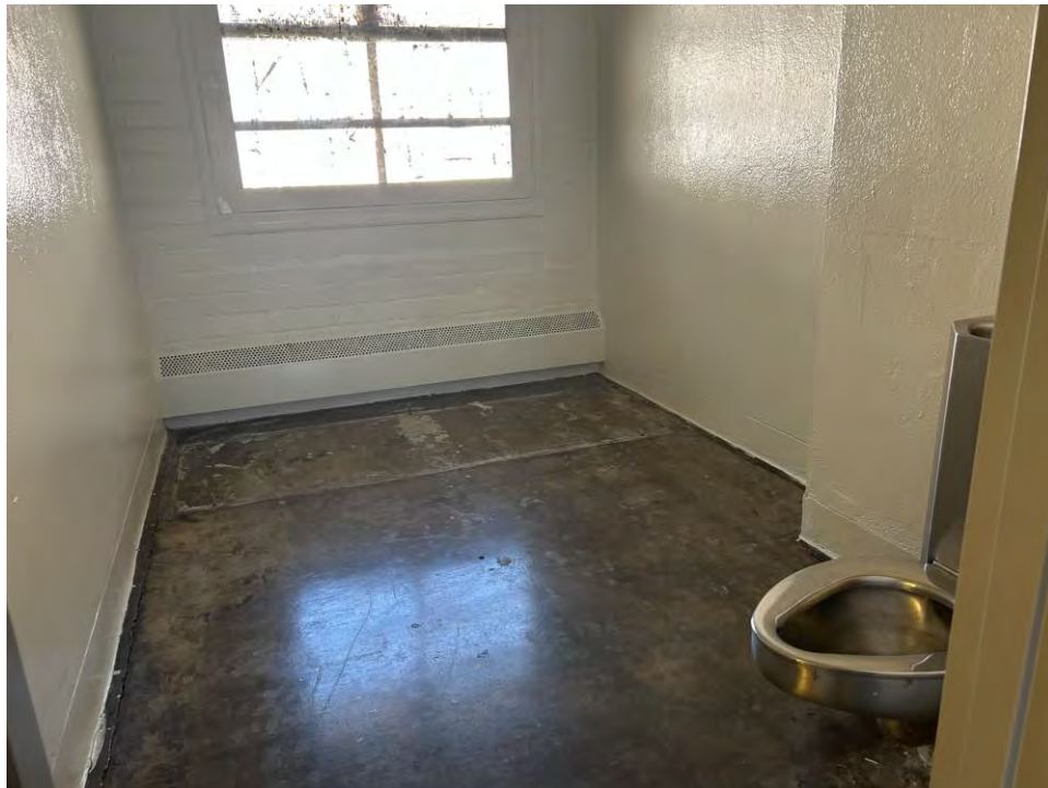
Figure 35. Example of a single cell within the Boys Secure Housing Unit. View toward north.
