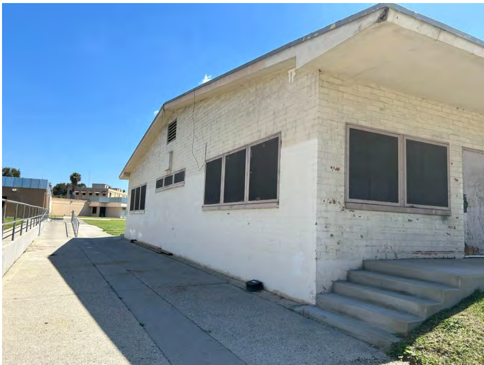
Figure 40. Side façade and detail of windows. View toward east.
