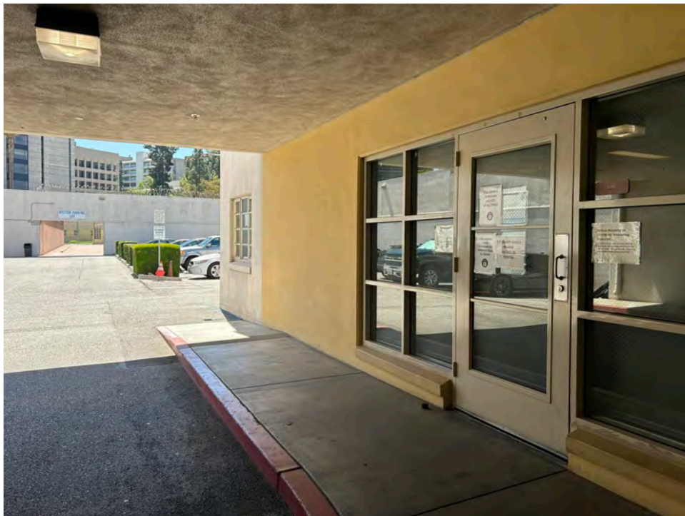
Image 3. Entrance into Court and Administration Building for admittance. View toward southeast.
