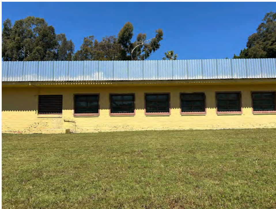
Photo 1. Detail of primary façade facing Central Juvenile Hall campus, view toward northwest.
