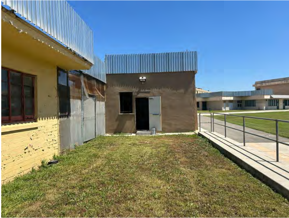
Figure 46. Side façade of Warehouse, to be accessed from juvenile delinquents. View toward northeast.
