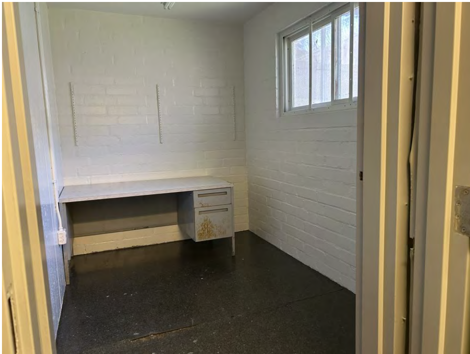
Figure 37. Example of the administration room, associated with the "X" rooms within the Boys Secure Housing Unit. View toward north.
