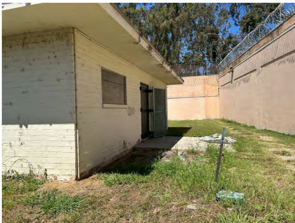
Photo 4. Side entrance into the building. View toward northwest.
