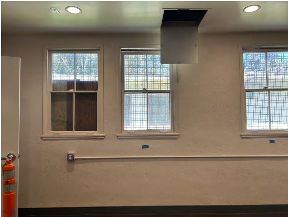
Figure 53. View of interior of Warehouse, view of personnel side of building. Note original, double hung, sash windows.
