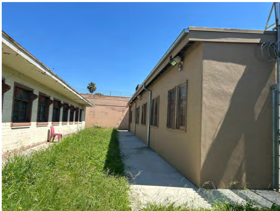
Photo 2. Side of Warehouse facing the Boys Maximum Security Unit. Note, this is the only side of the building with (historic era) windows. View toward northeast.
