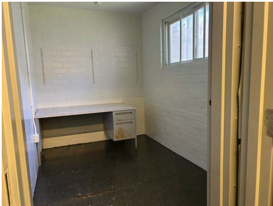
Photo 13. Example of the administration room, associated with the "X" rooms within the Boys Secure Housing Unit. View toward north.
