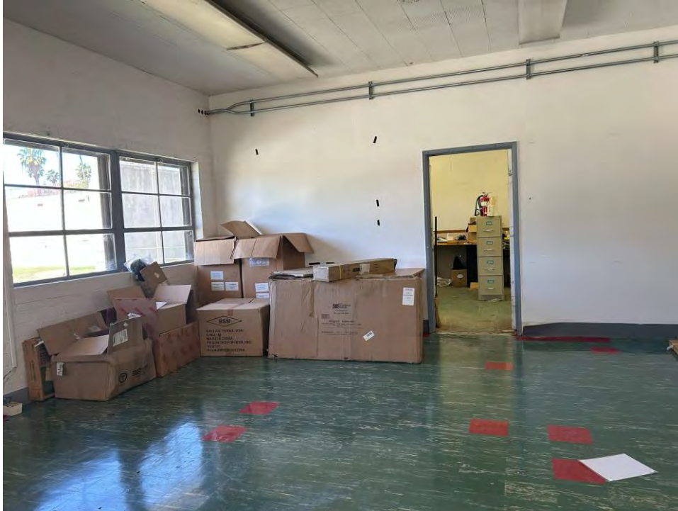
Figure 41. Interior of Mess Hall, view of dining area and asbestos tile floor. View toward northwest.
