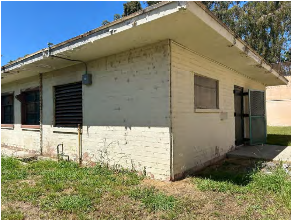
Figure 29. Side end of the building, with windows visible and vents for the “X” room visible. View toward northwest.
