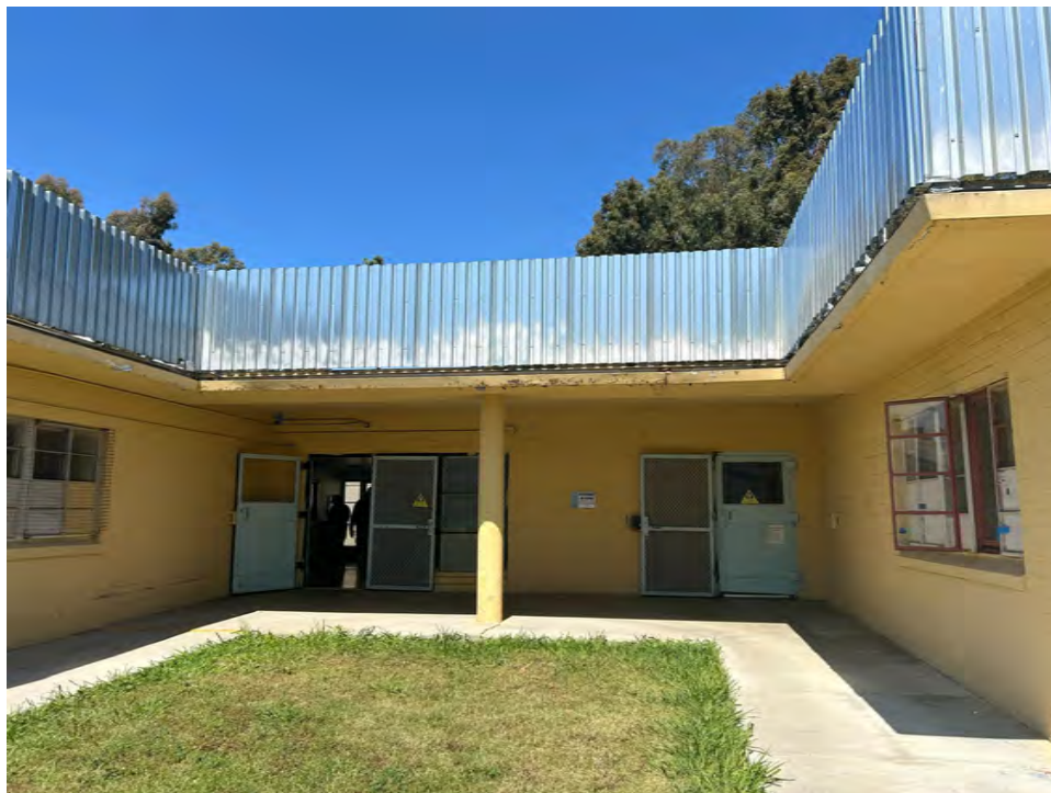
Photo 3. Primary façade dual entrance space. View toward northwest.
