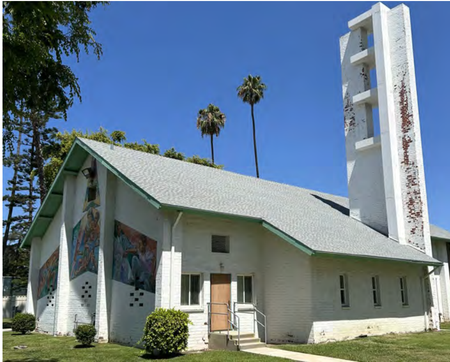
Image 5. Chapel at center of Central Juvenile Hall. View toward northeast.
