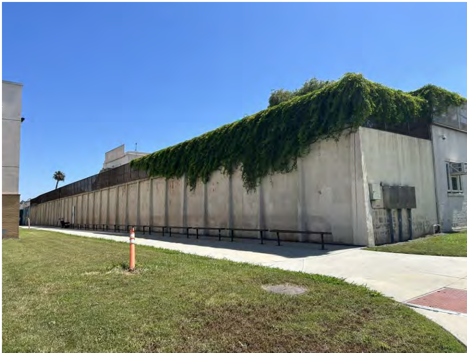
Figure 17. View from interior of Central Juvenile Hall Campus, example of 15-foot concrete walls that surround the facility. View toward northeast.
