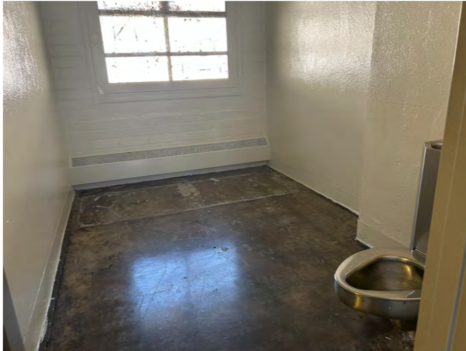
Photo 11. Example of a single cell within the Boys Secure Housing Unit. View toward north.
