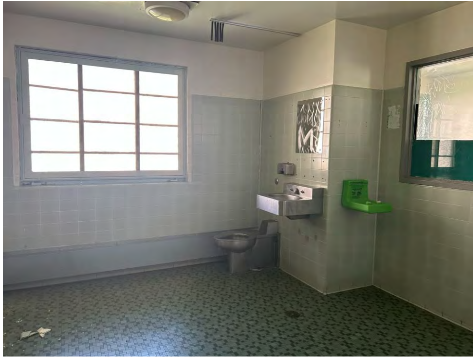
Figure 34. View of toilet and shower room. View toward north.
