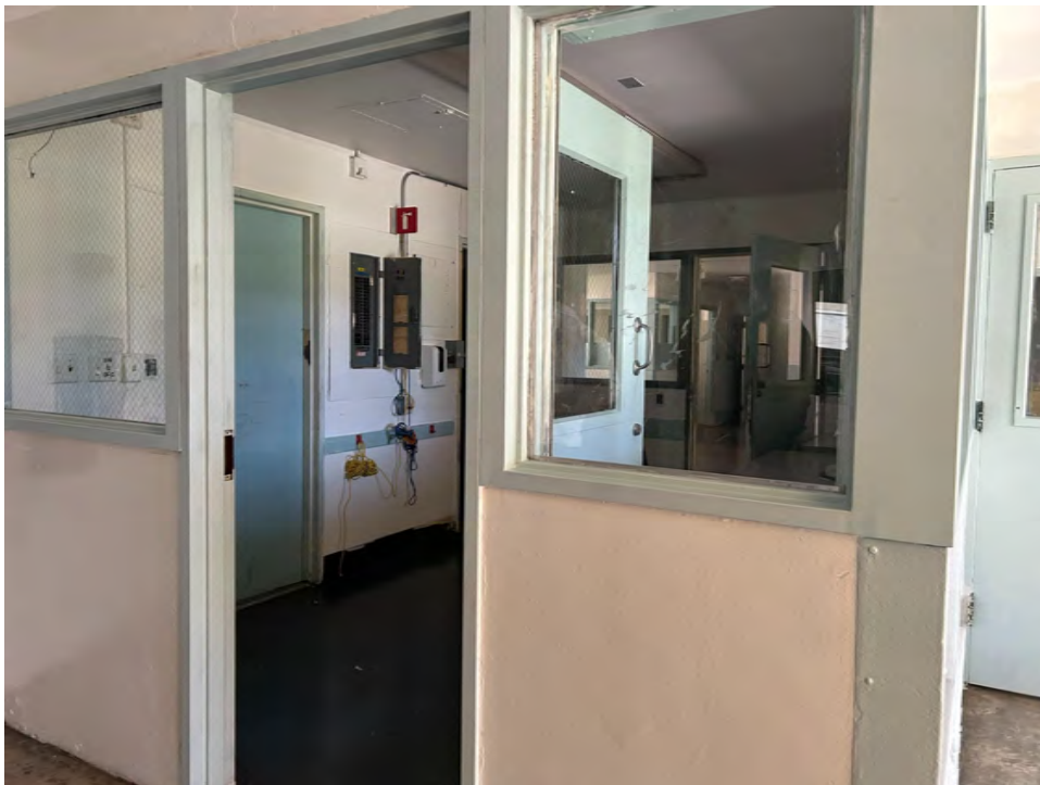
Photo 6. Interior central personnel area. View toward northeast.
