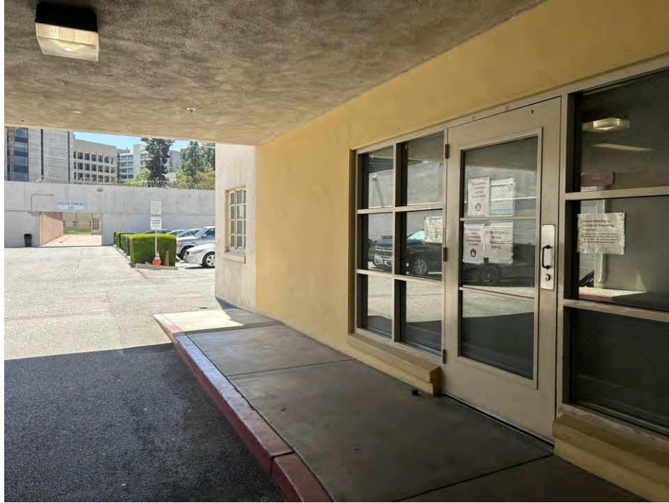
Figure 18. Entrance into Court and Administration Building for admittance. View toward southeast.
