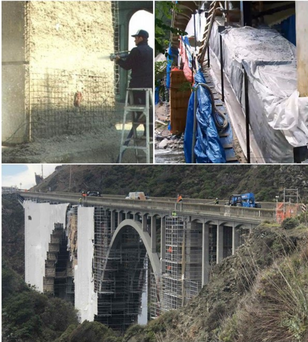
Figure 1-5: Example of Electrochemical Chloride Extraction Set-Up
