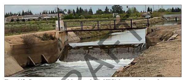
Figure 4-15 Drop structure toward the west end of the Mill Ditch segment, facing northeast.
