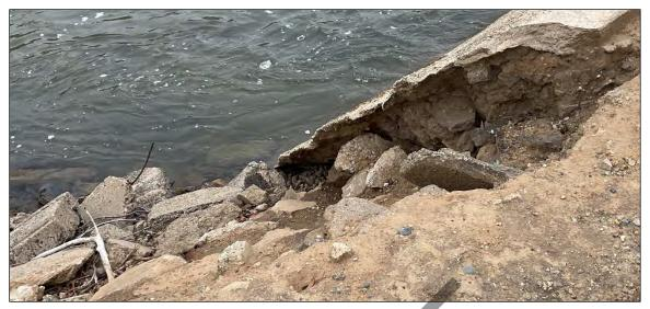
Figure 4-12 Segment conditions showing deterioration on concrete lining, facing northeast.
