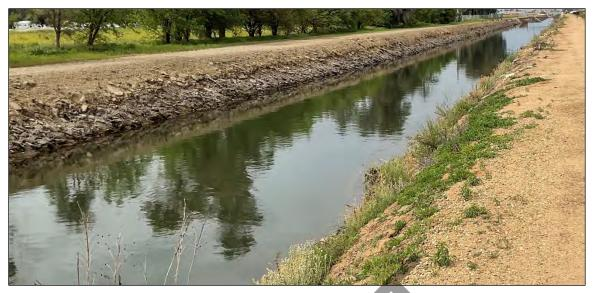
Figure 4-10 Mill Ditch segment from the north bank, with detail of vegetation intrusion on the earthen banks, facing southwest.
