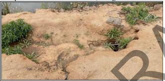
Erosion and animal burrowing on the earthen bank of the Mill Ditch segment, facing south.
