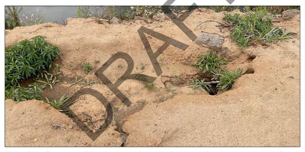
Figure 4-11 Segment condition showing erosion and animal burrowing on the earthen bank, facing south.
