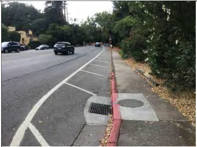
Photo 2. Storm drain inlet on Sir Francis Drake Boulevard within Project site. Taken facing south.
