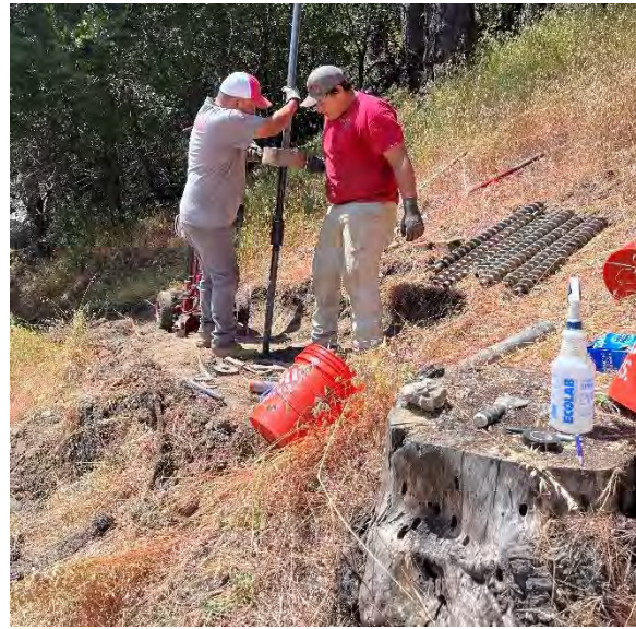
PHOTO 1.3-1: Soil sampling at Boring 1-B1.
