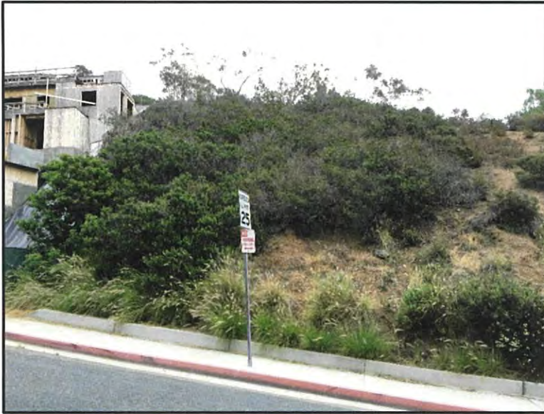
Photograph 1. Street view of front portion of the project site (right-hand side of speed limit sign). A narrow city "paper" street, Highland Road, exists between the house under construction and project site. Photograph taken facing east.
