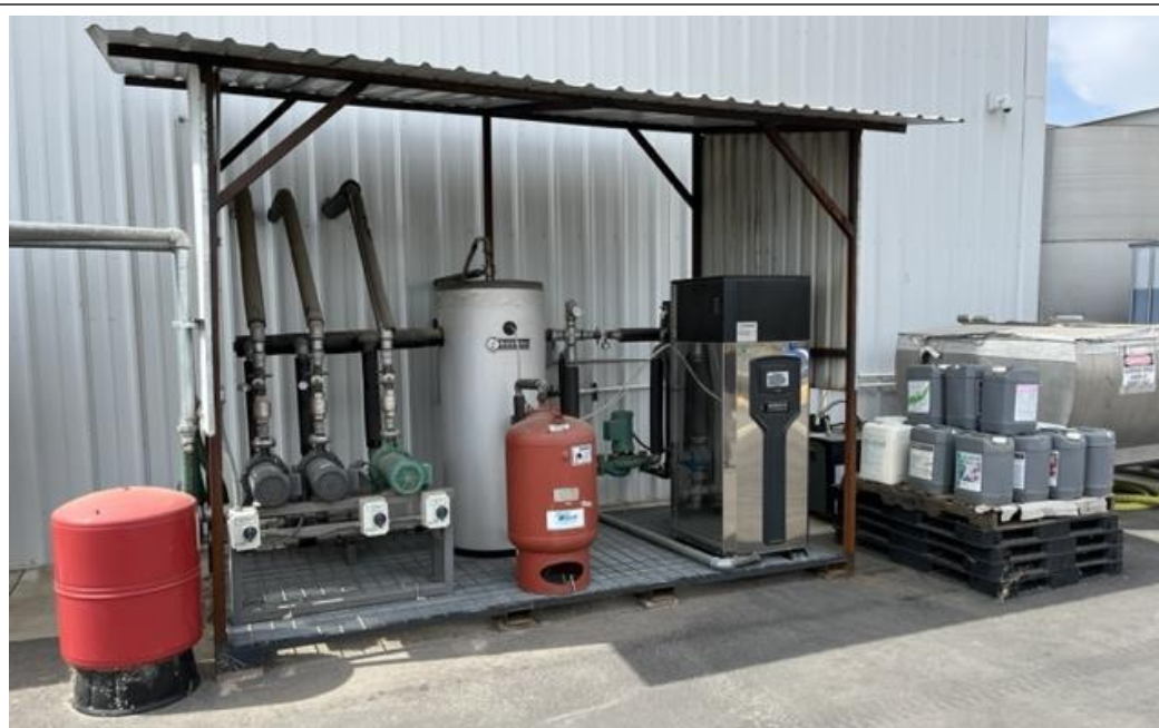
Water heater for generating hot water piped to indoor mixing tanks.
