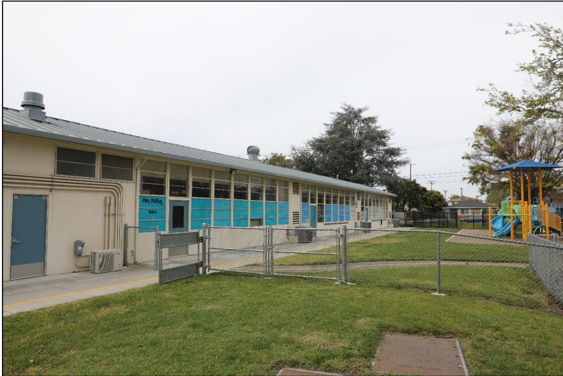
Photo 3. Viewing west along the existing Building A classroom building toward Scott Boulevard.
