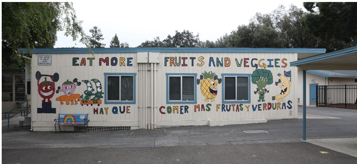
Photo 2. Building 5, north façade, view south
