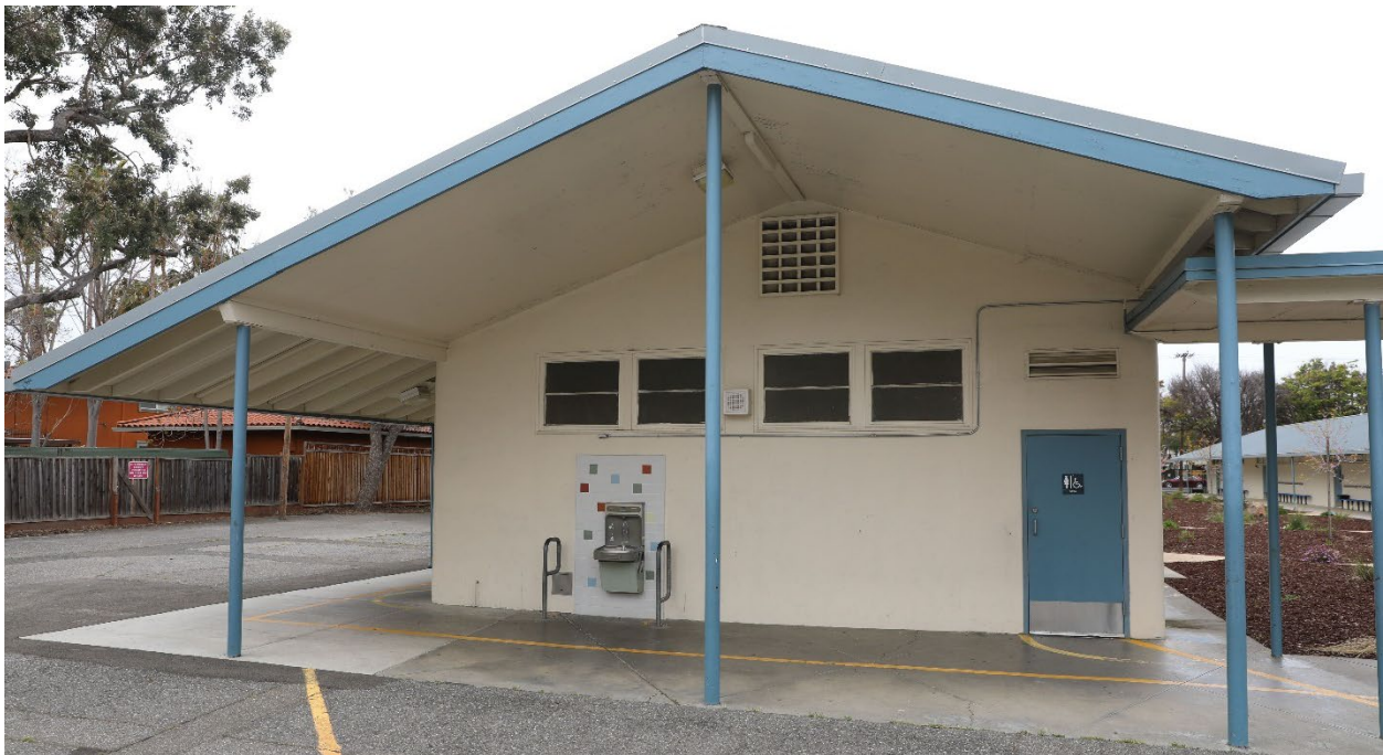
Photo 2. Building E, east façade, view west
