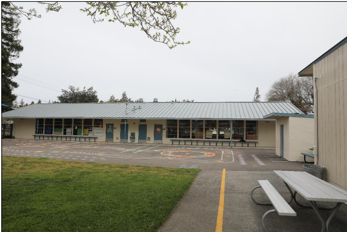
Photo 4. Viewing north toward the existing Kindergarten building.
