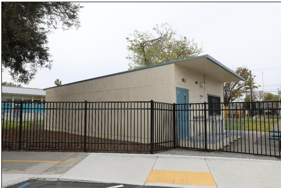
Photo 6. Existing transitional kindergarten portable.
