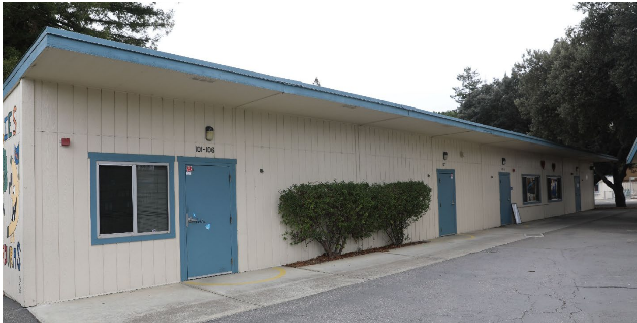
Photo 1. Building 5, west façade, view southwest
