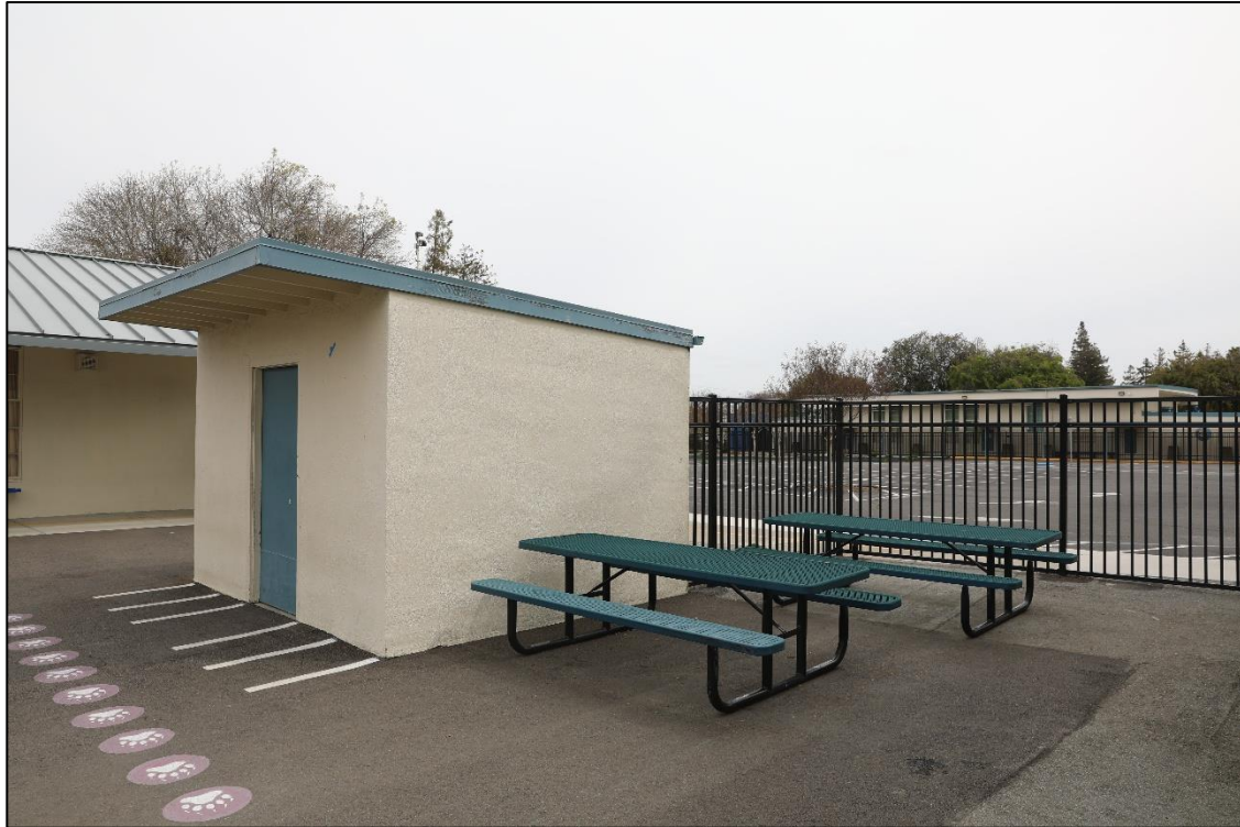
Photo 5. Existing storage building in kindergarten play area.
