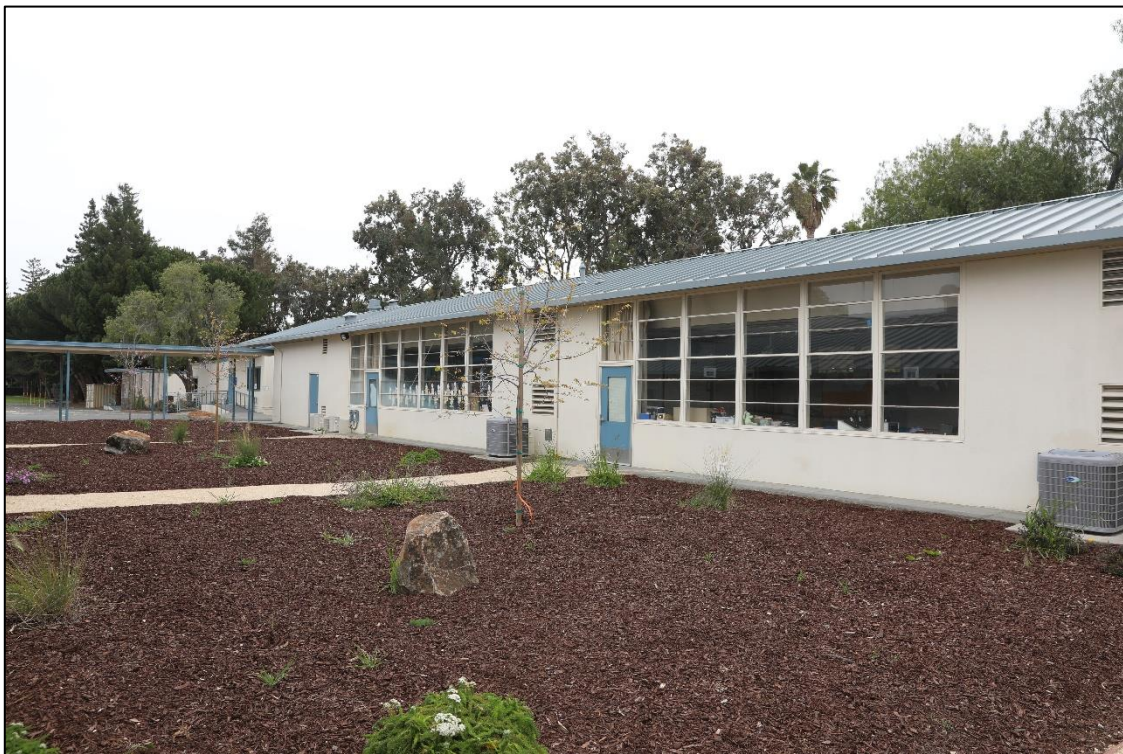
Photo 8. Viewing southeast toward the existing classroom building E from landscape area.
