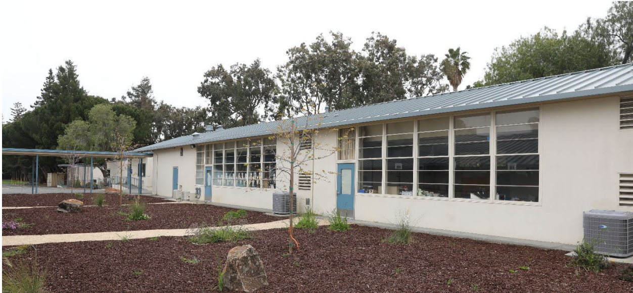
Photo 1. Building E, north façade, view southeast
