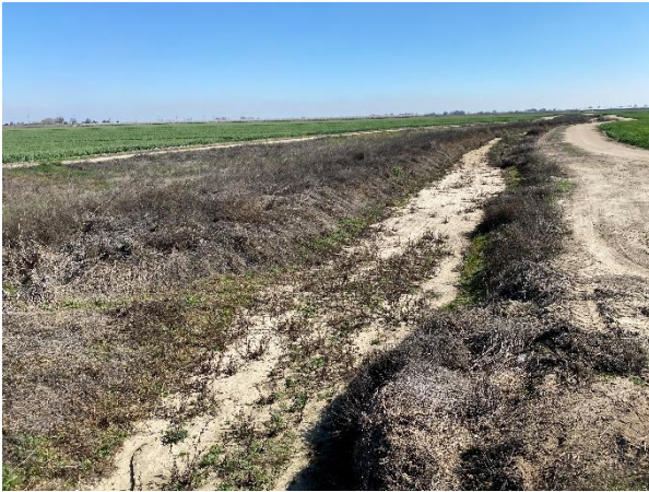
Photo 7 – Murphy Slough at S. Marks Ave., facing East.
