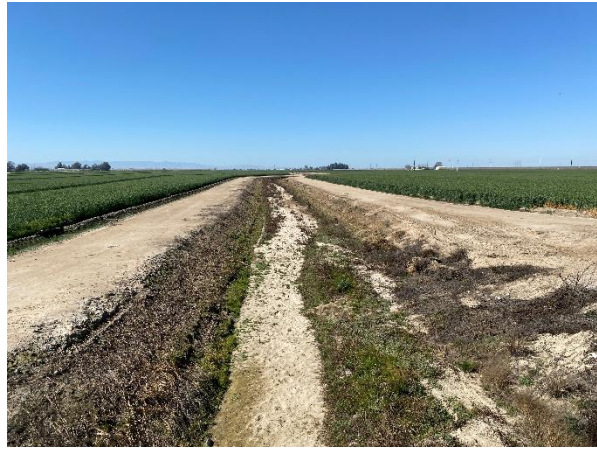
Photo 8 – Murphy Slough at S. Marks Ave., facing West.
