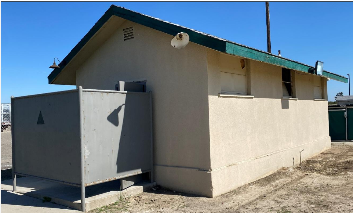
Figure 4-18 West and south elevations of the restroom facility, facing northeast.
