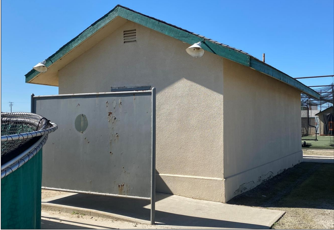
Figure 4-17 East and north elevations of the restroom facility, facing northwest.
