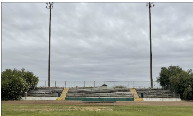
Smaller, east set of stadium seating, facing east.
