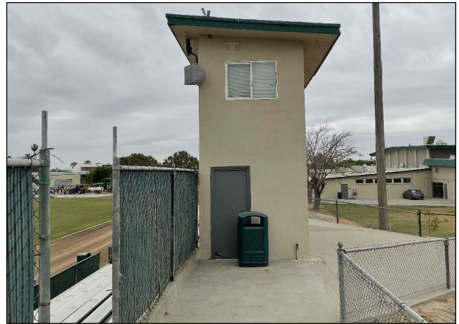
North elevation of the press box building, facing south.
