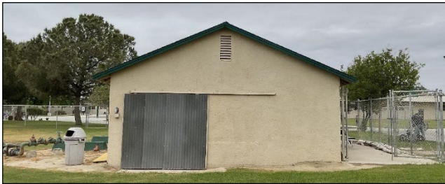
Rear (north) elevation of the pump building, facing south.
