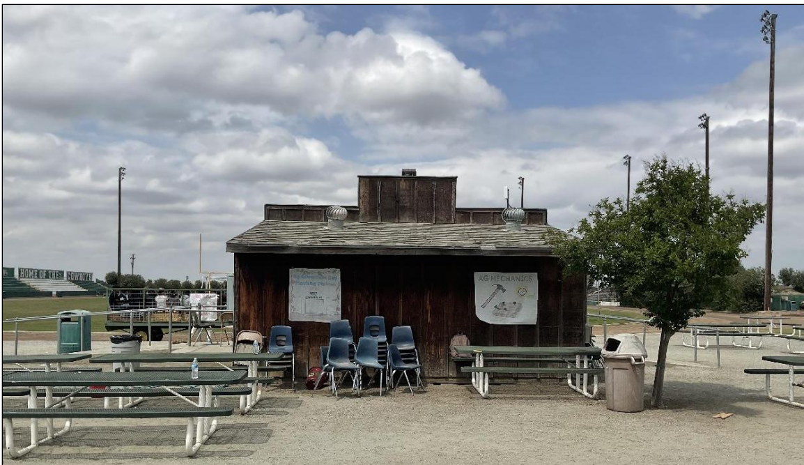
Figure 4-22 Rear (south) elevation of the concession building, facing north.
