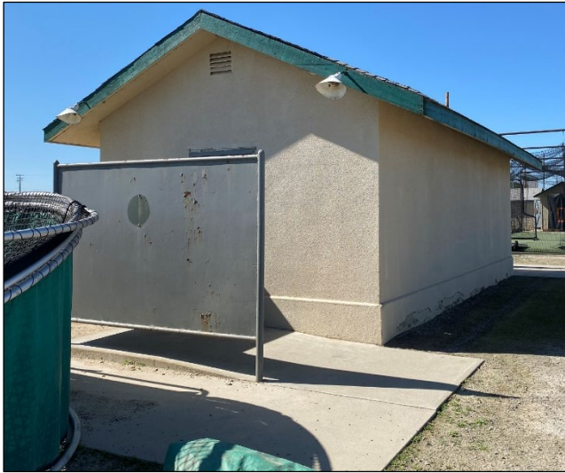
East and north elevations of the restroom facility, facing northwest.
