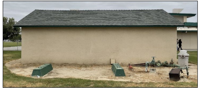
East elevation of the pump building, facing west.
