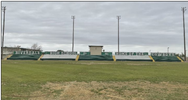
Larger, west set of stadium seating with east elevation of the press box, facing west.
