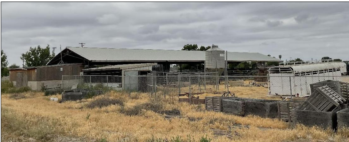
Figure 4-24 Agricultural barn facilities, facing southwest.
