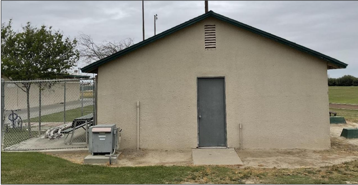
Figure 4-19 Primary (south) elevation of the pump building, facing north.
