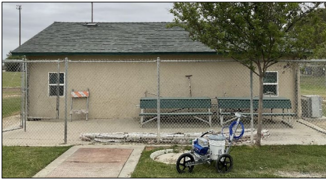
West elevation of the pump building, facing east.
