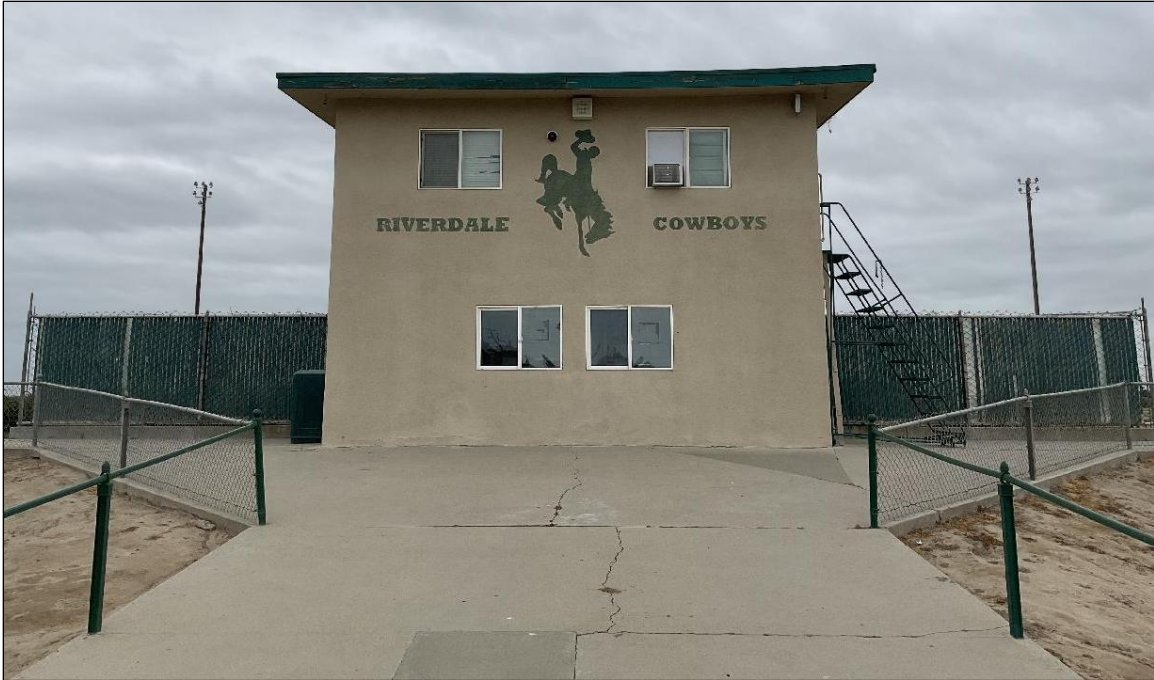
Figure 4-16 West elevation of the press box at the west entrance to the stadium, facing east.
