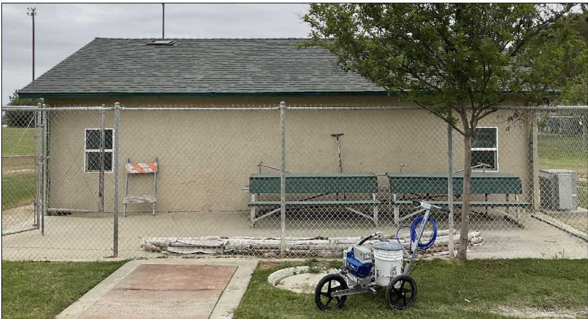
Figure 4-20 West elevation of the pump building, facing east.
