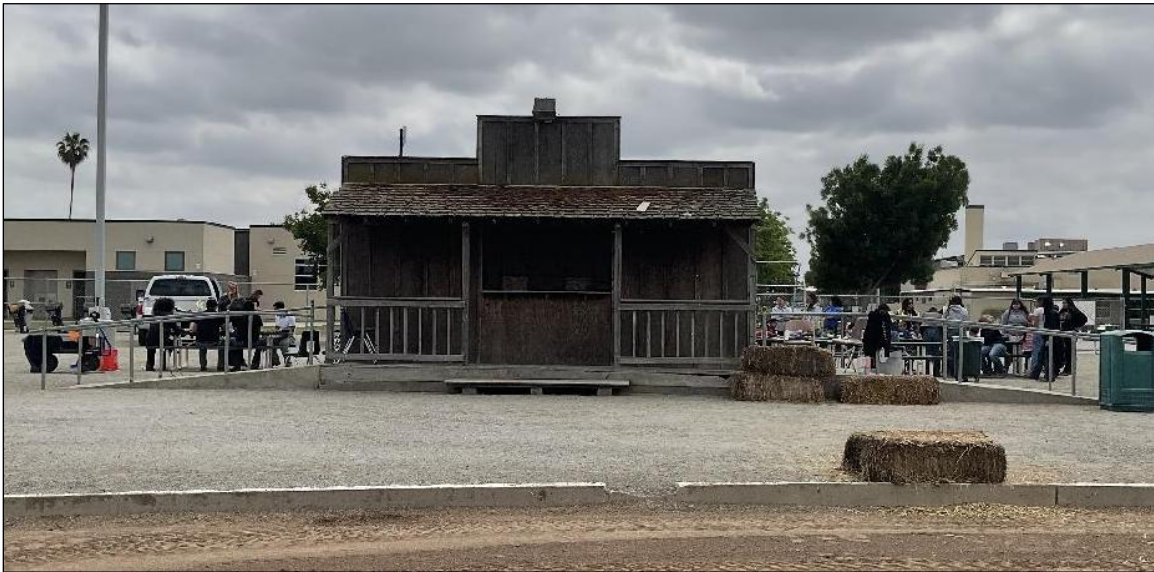
Figure 4-21 Primary (north) elevation of the concession building, facing south.
