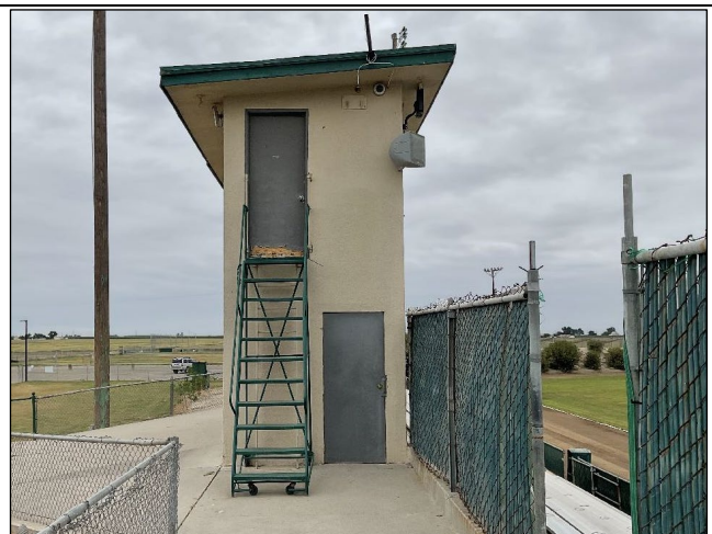
South elevation of the press box building, west entrance to the left, and west bleachers to the right, facing north.
