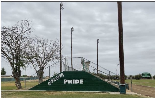
South elevation of the west stadium seating, facing north.
